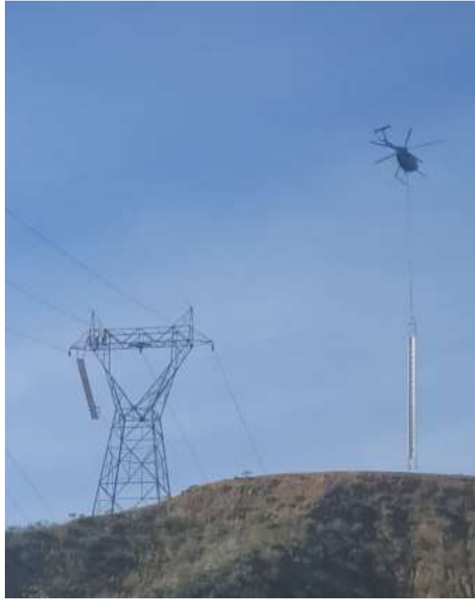
Photo 1 – Delivery of materials to wreck-out towers in Segment 3 using a helicopter.
