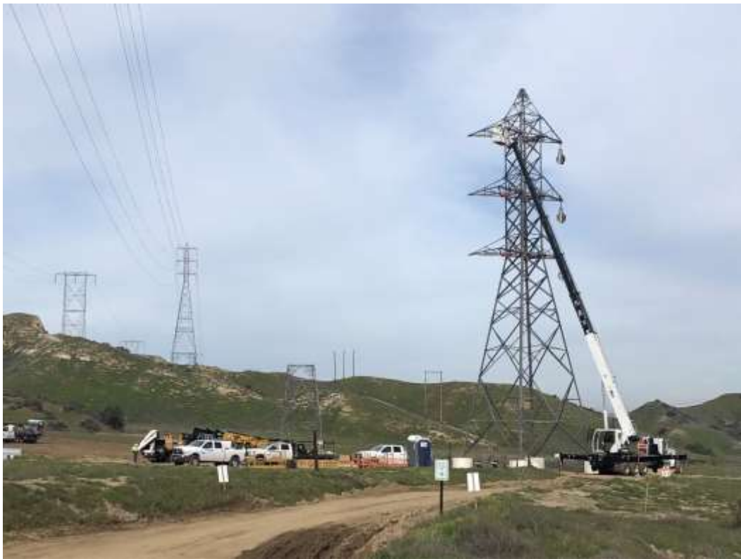
Photo 3 – Wire stringing operations between Sites 3N02 and 3X06, Segment 3.
