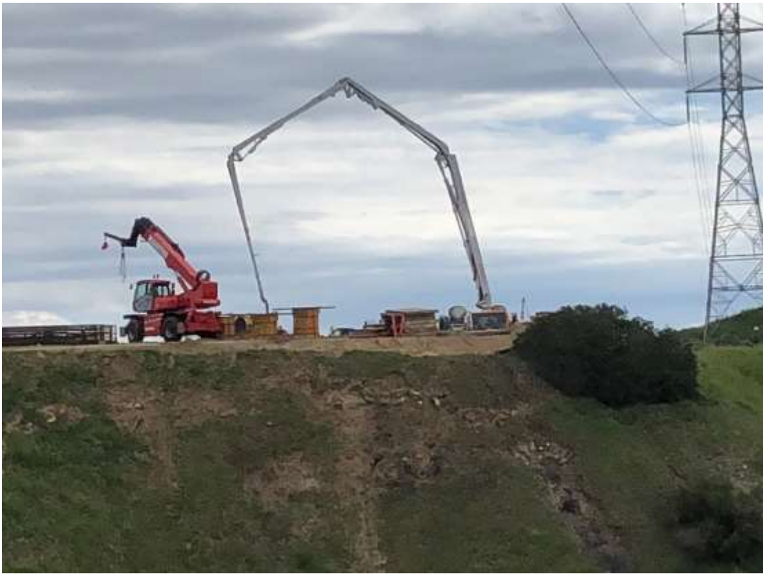
Photo 3 – Foundation pouring at Site 3X43, Segment 3.
