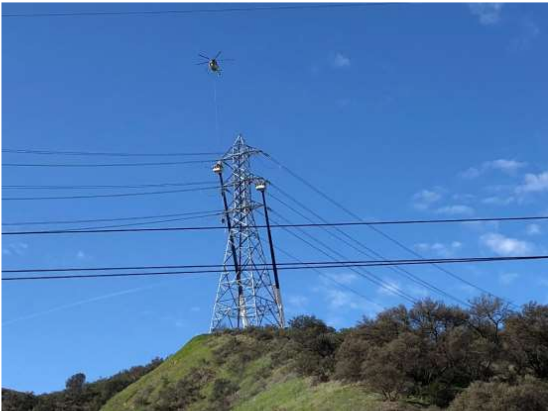
Photo 4 – Wire stringing activity at Site 3N02 with helicopter support, Segment 3.
