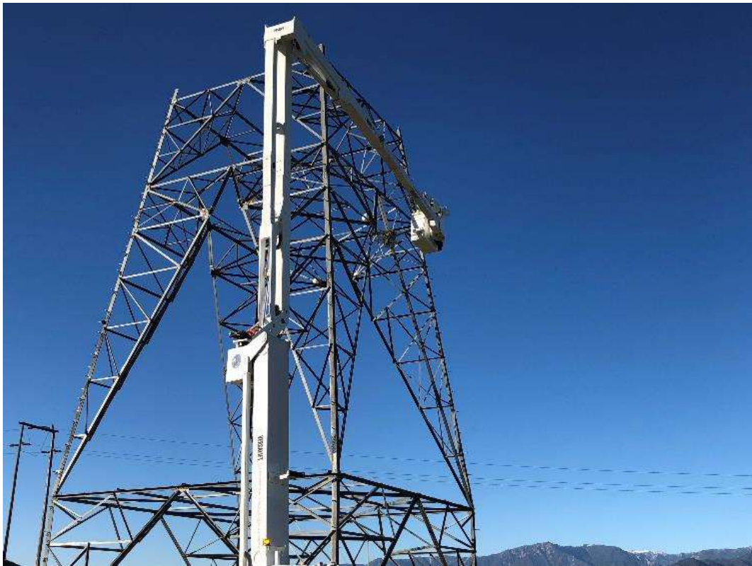
Photo 5 – Relocating active red-tailed hawk nest from tower at Site 3X06-3X07 (March 13, 2019).
