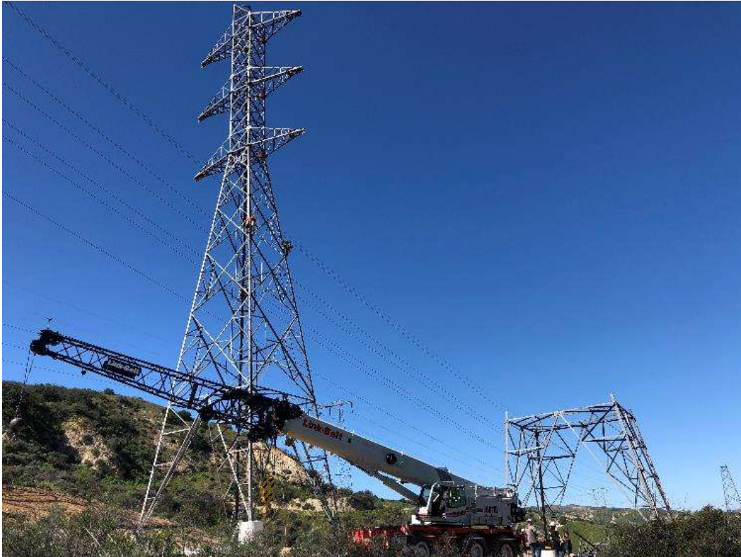
Photo 1 – Completing tower assembly at Site 3X21, Segment 3.
