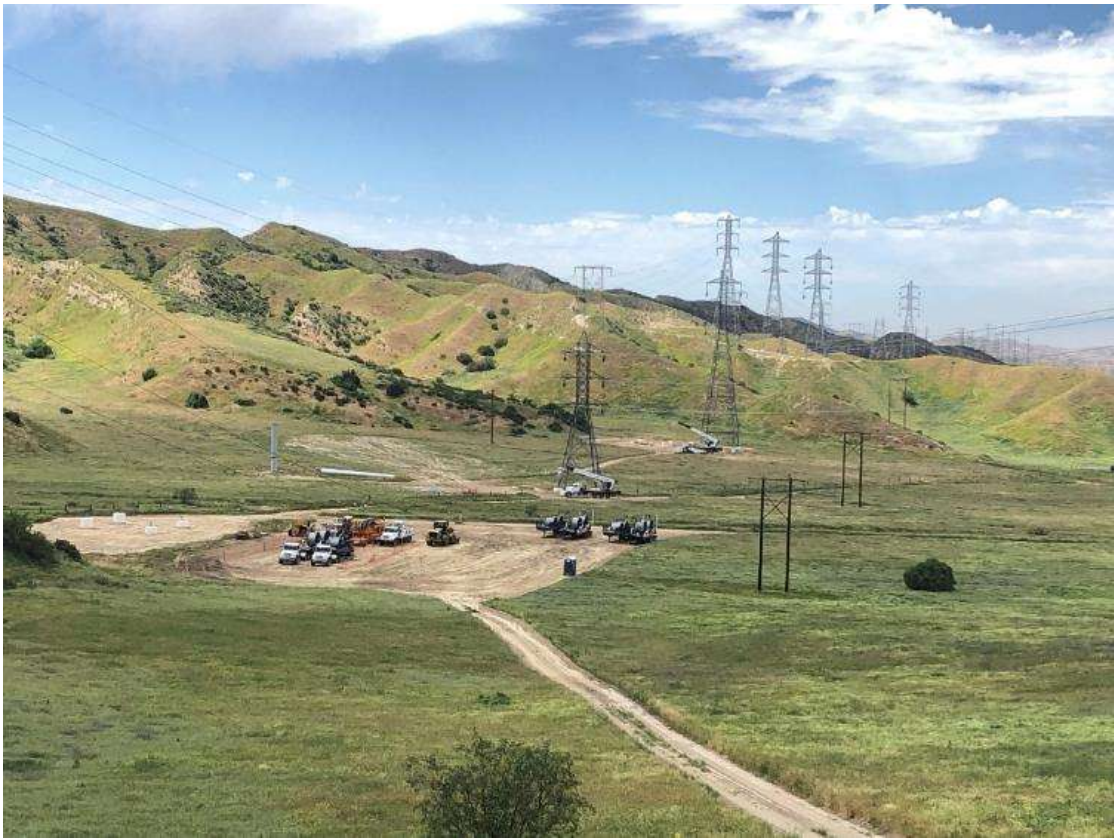
Photo 5 – Stringing activities occurred in Segment 3 (April 19, 2019).
