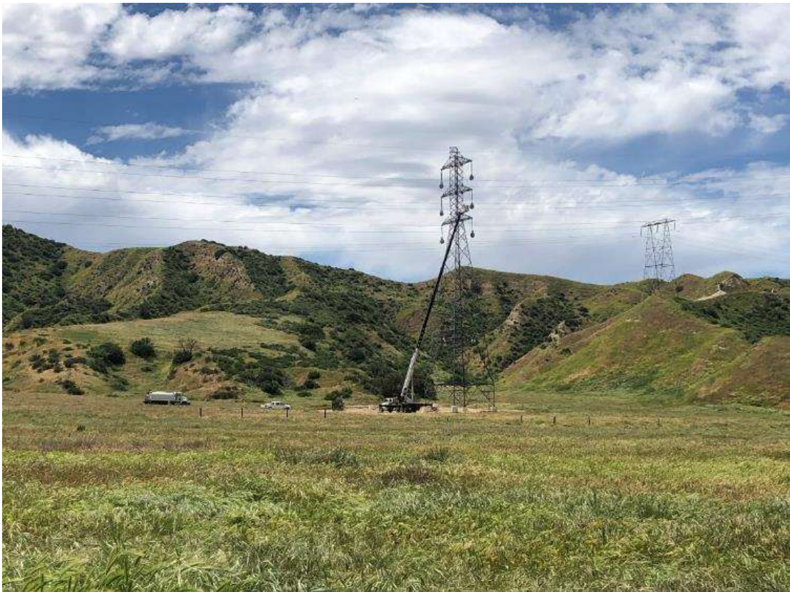
Photo 4 – Stringing activities occurred in Segment 3 (April 19, 2019).
