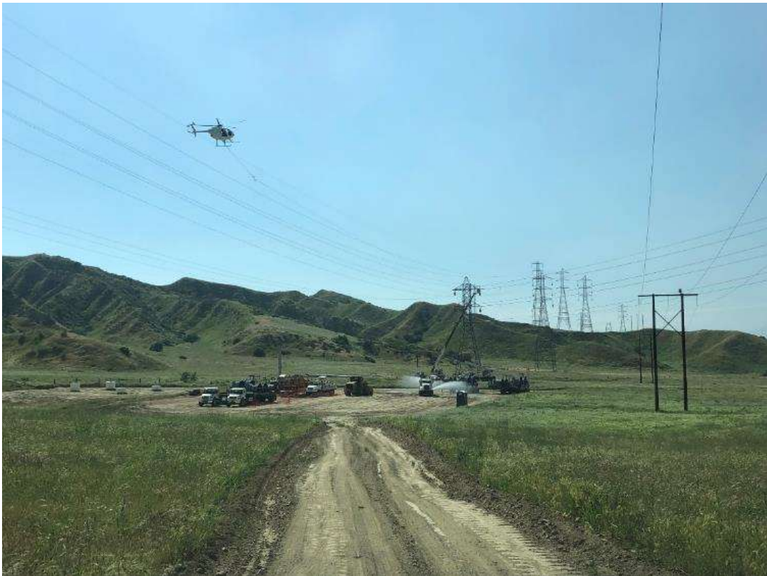
Photo 6 – Helicopter pulling line in Segment 3 (April 19, 2019).
