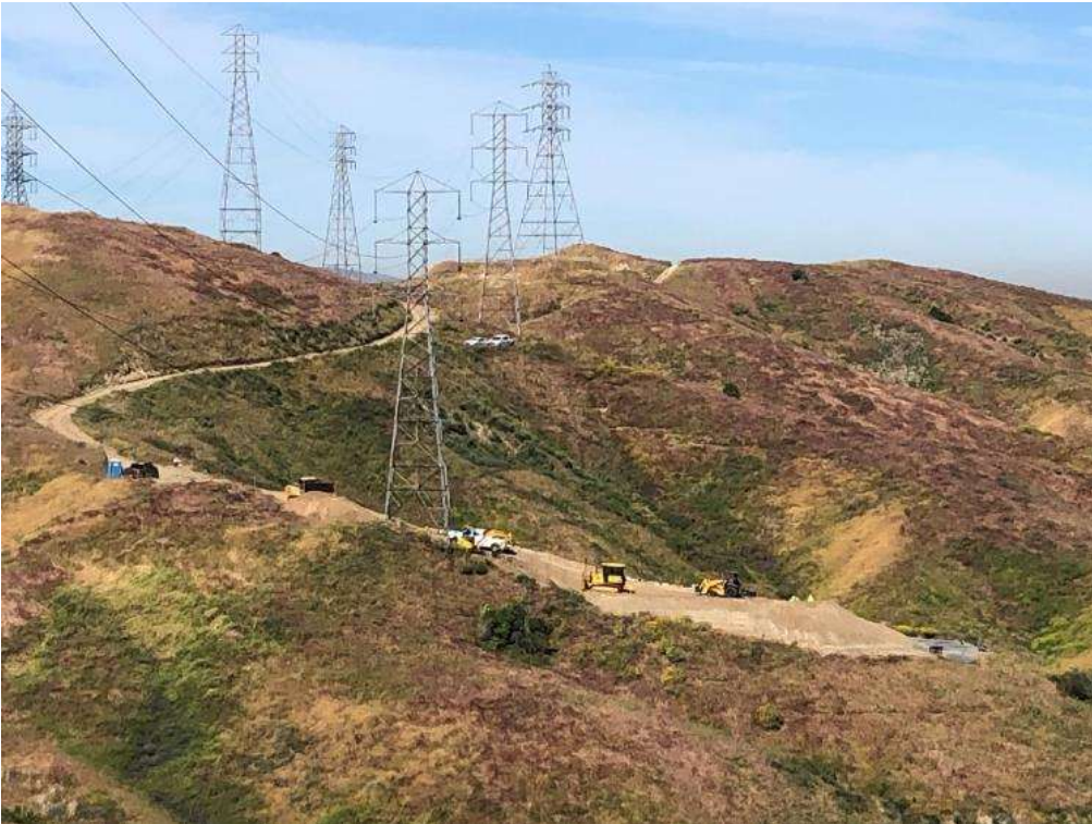
Photo 2 – Grading occurred at sites in Segment 2 (April 16, 2019).
