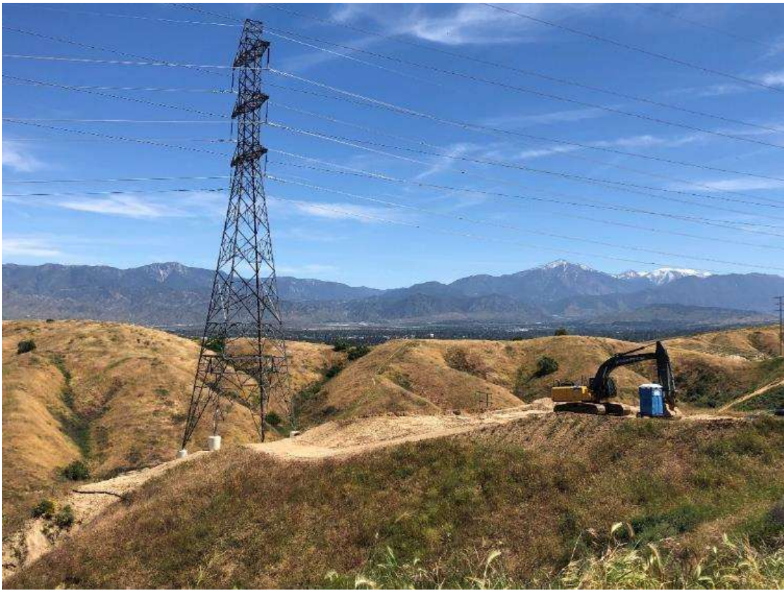
Photo 3 – Grading occurred in Segment 3 (April 17, 2019).
