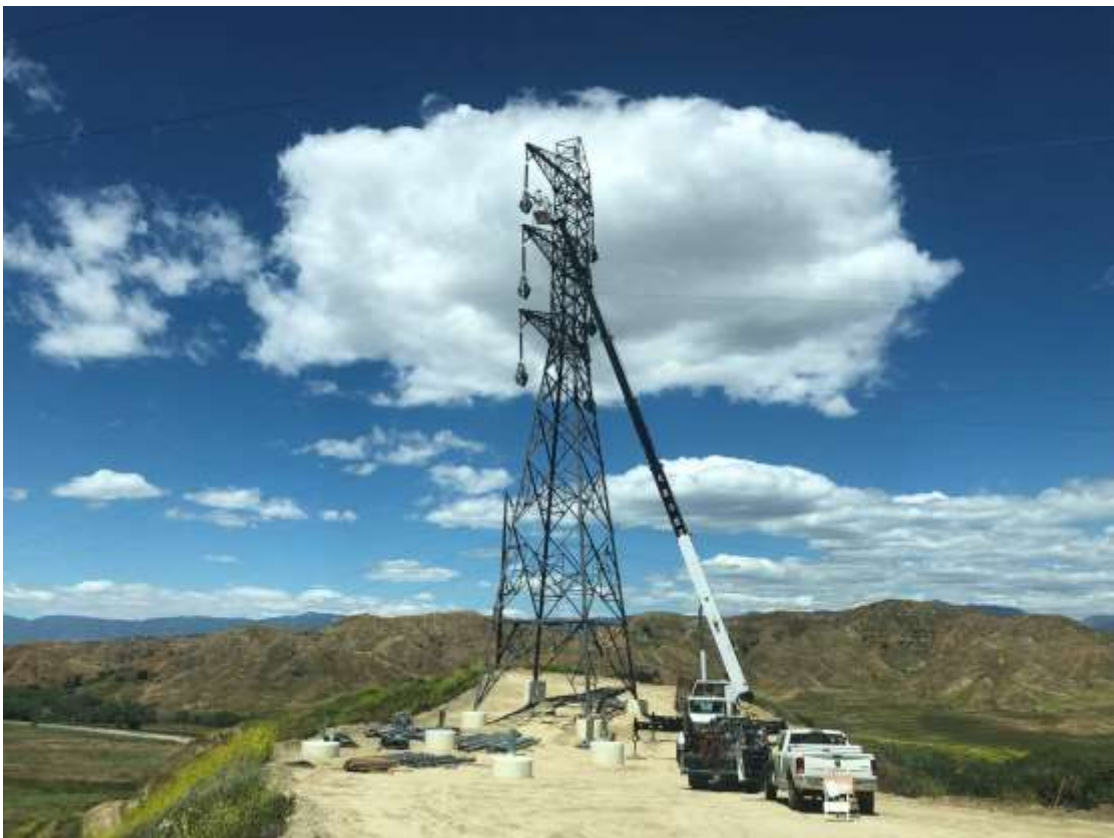
Photo 4 – Wire stringing activities occurred in Segment 3 (April 23, 2019).
