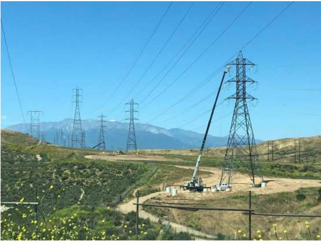
Photo 3 – Wire stringing activities occurred in Segment 3 (April 23, 2019).
