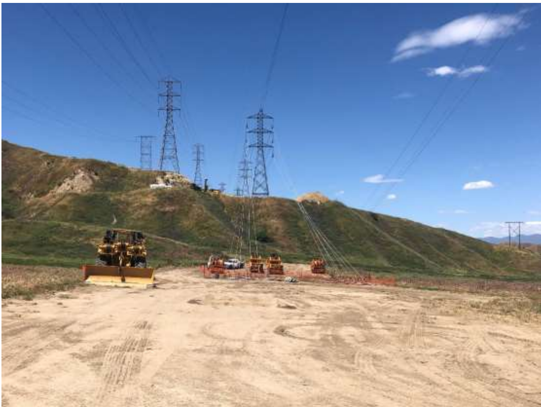
Photo 6 – Wire pulling activities occurred in Segment 3 (April 24, 2019).
