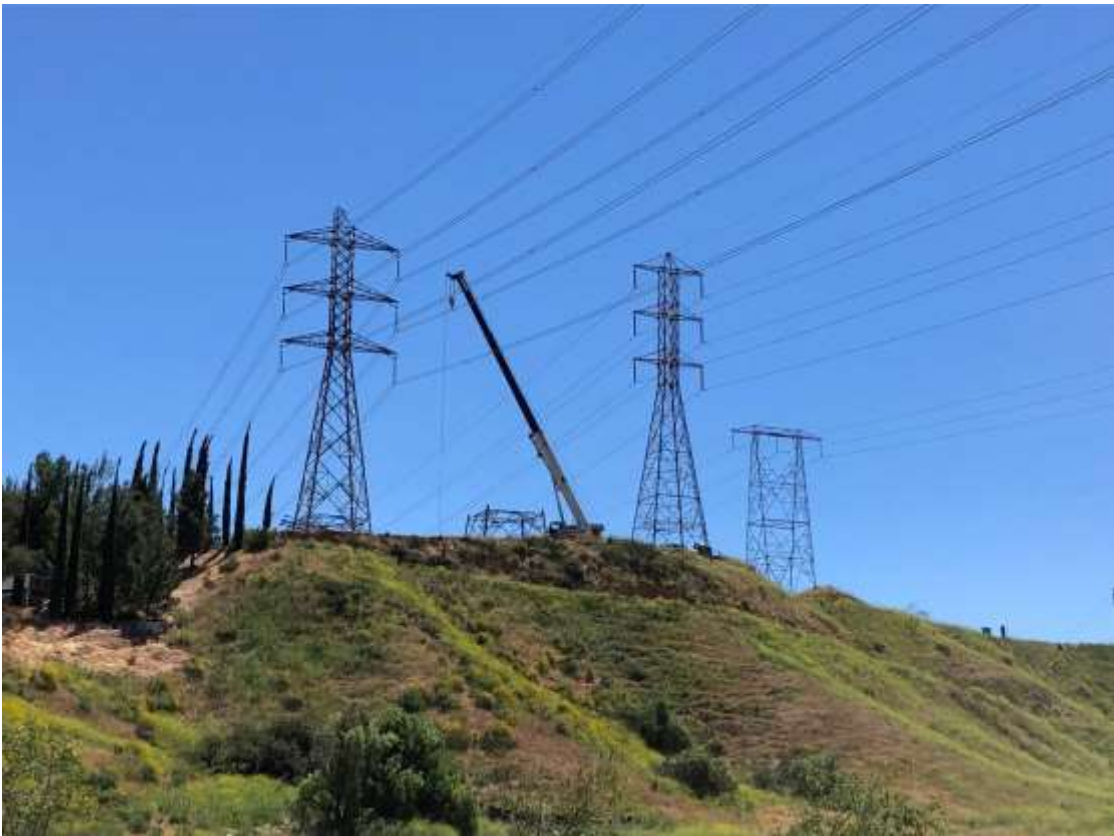
Photo 5 – Tower assembly activities occurred in Segment 3 (April 23, 2019).
