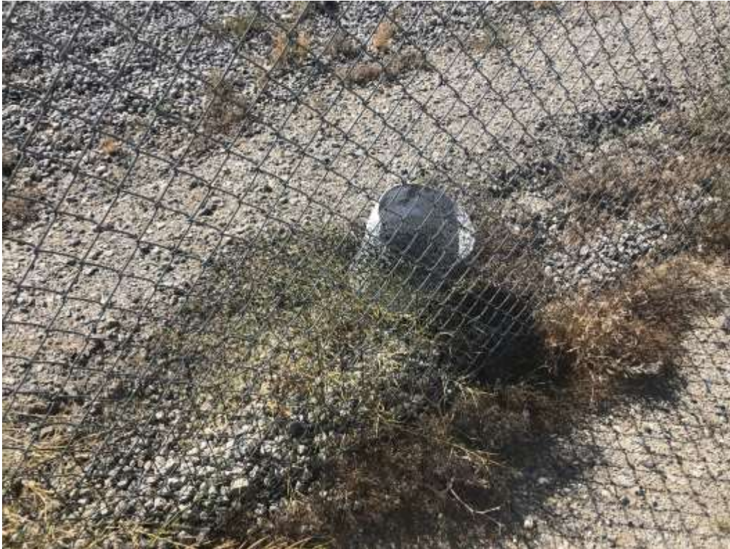
Photo 1 – Loose monofilament netting was observed in the Devers MY. The issue was corrected. (April 22, 2019).
