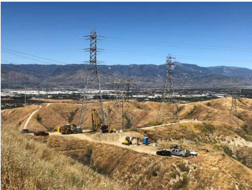
Photo 2 – Grading and drilling occurred in Segment 2 (April 24, 2019).
