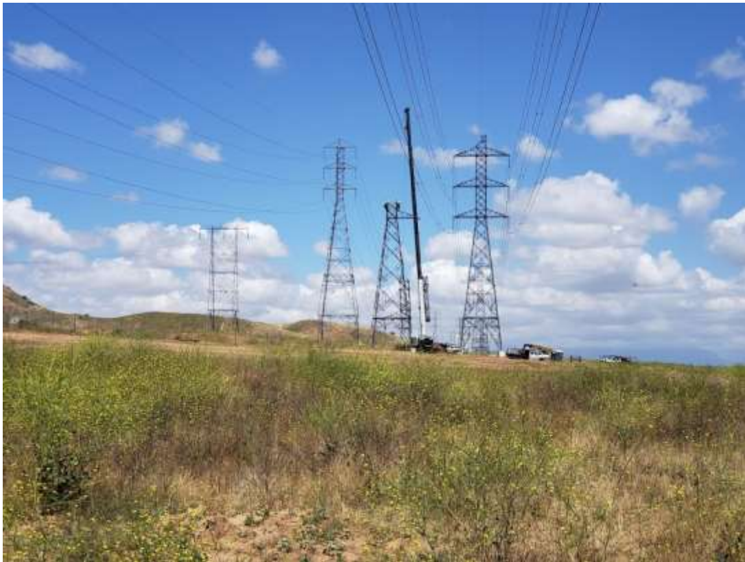
Photo 3 – Tower Assembly on Segment 3 (May 20, 2019).
