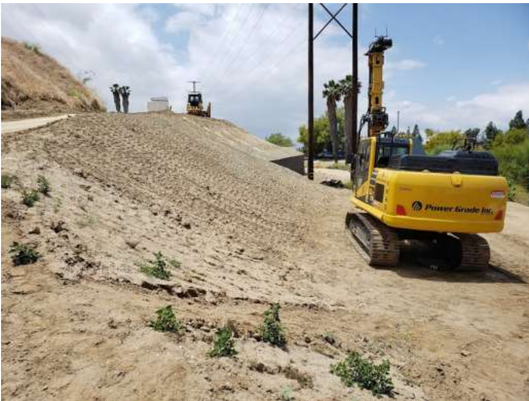
Photo 2 – Grading activities on Segment 2 (May 21, 2019).
