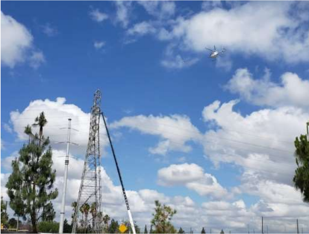
Photo 1 – Wire removal activities on Segment 1 (May 20, 2019).
