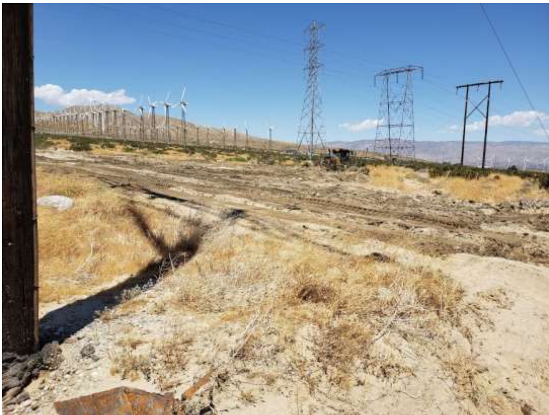
Photo 4 – Clearing and grubbing activities on Segment 6 (May 20, 2019)
