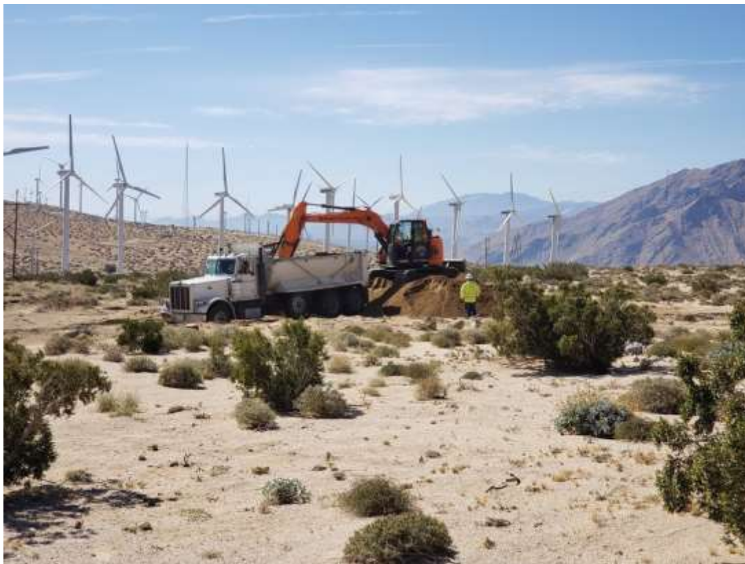
Photo 4 – Clearing, grubbing, and soil export activities on Segment 6 (May 28, 2019)
