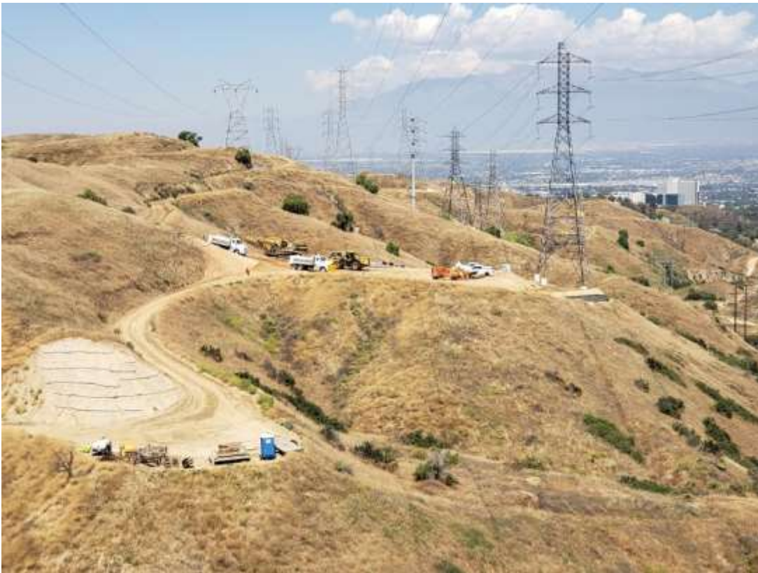
Photo 3 – Grading and soil export activities on Segment 3 (May 28, 2019).
