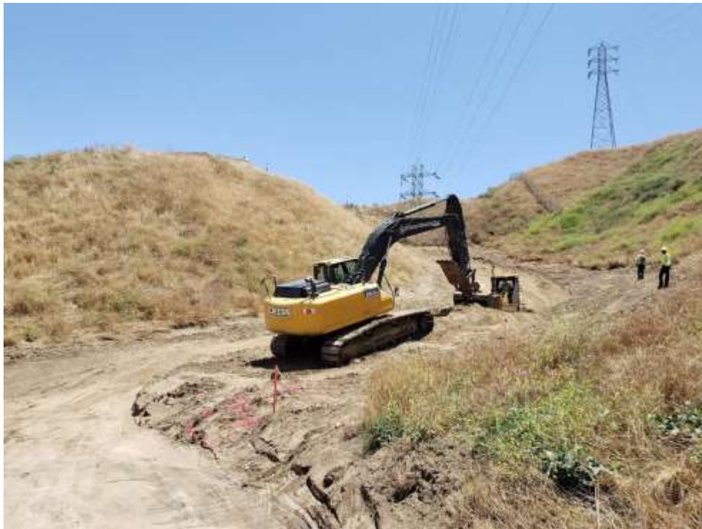
Photo 2 – Grading activities on Segment 2 (May 28, 2019).
