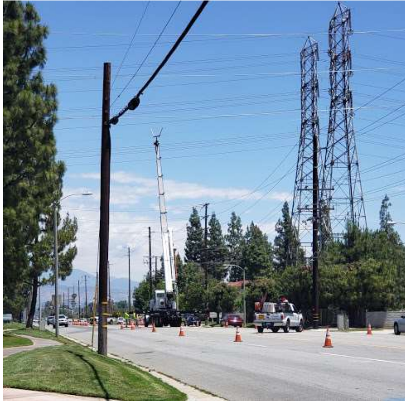
Photo 1 – Wire removal activities on Segment 1 with proper traffic control (May 29, 2019).
