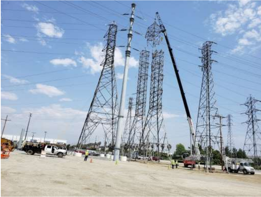
Photo 1 – Tower wreck-out activities on Segment 1 (June 3, 2019).
