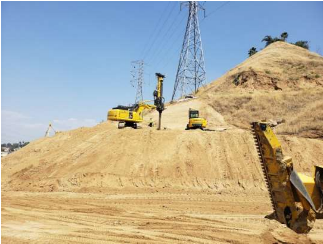
Photo 3 – Soldier pile wall drilling on Segment 2 (June 5, 2019).
