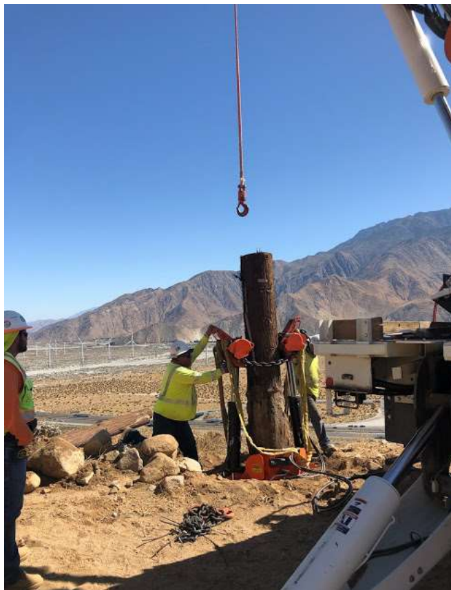
Photo 6 – H-frame removal at Construction Area T248 on Segment 6 (September 12, 2019).
