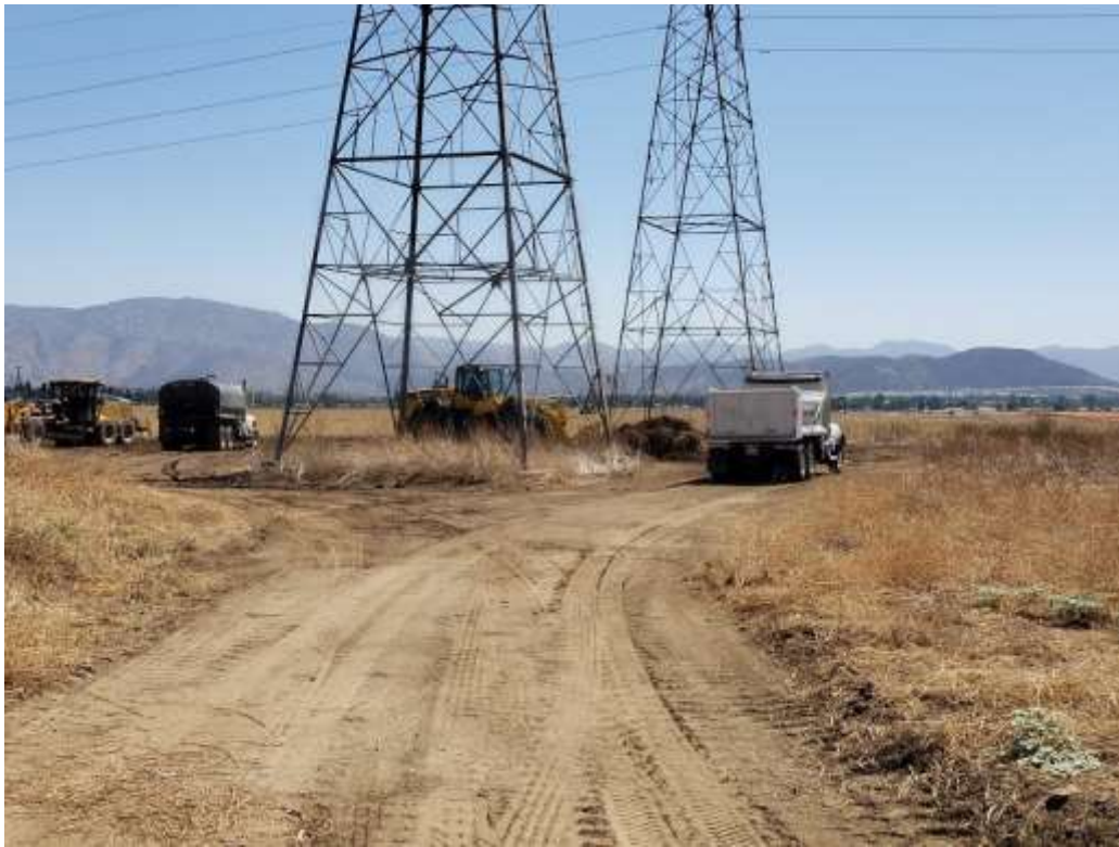
Photo 3 – Grading and soil export at Construction Area 4X20 on Segment 4 (September 11, 2019).
