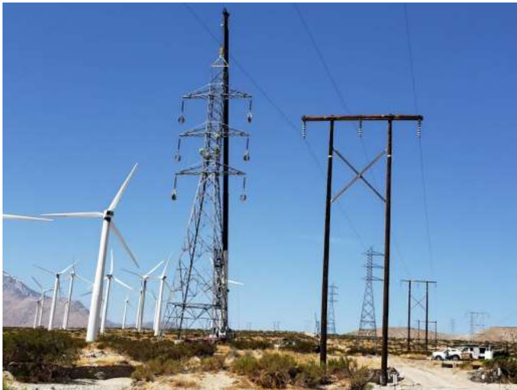
Photo 5 – Tower assembly at Construction Area 6S23 on Segment 6 (September 9, 2019).
