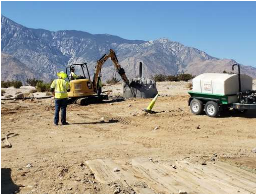
Photo 4 – Foundation wreck-out at Construction Area 6N27 on Segment 6 (September 9, 2019).
