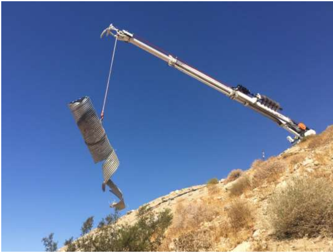
Photo 3 – Corrugated pipe retrieval at T248 (September 20, 2019) (Photo courtesy of SCE).
