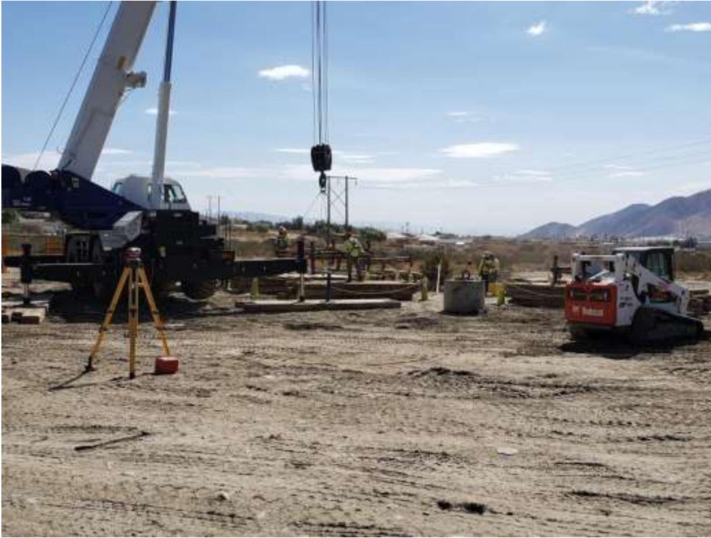
Photo 1 – Foundation activities at Construction Area 6X41 (September 16, 2019).
