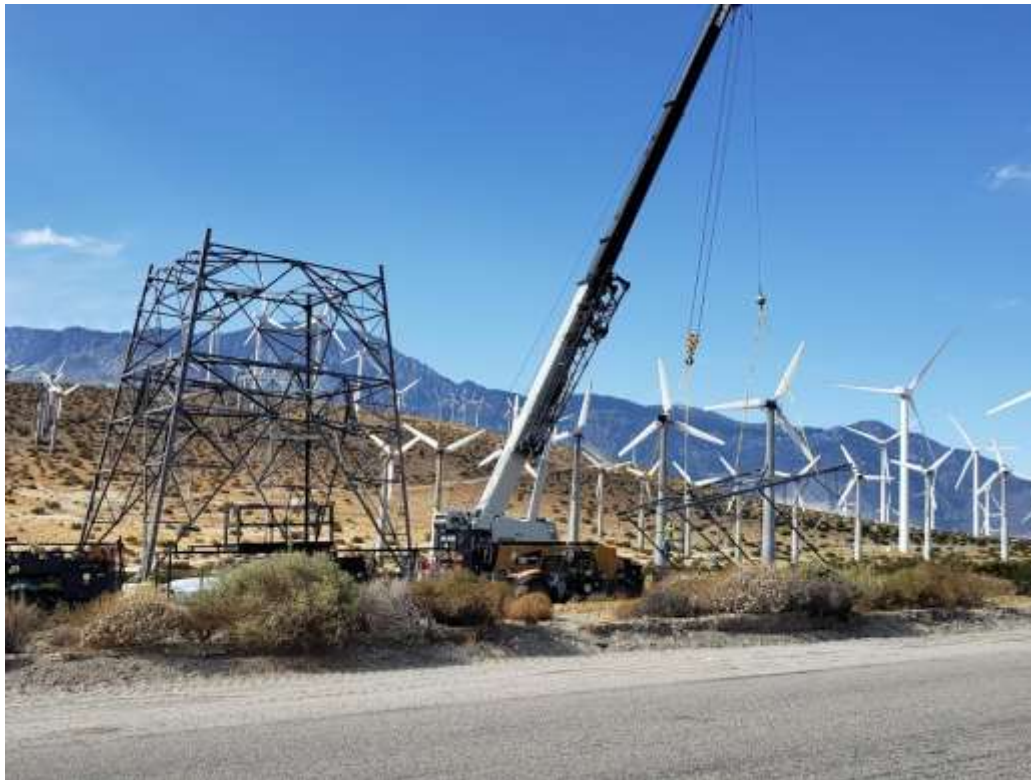
Photo 2 – Tower Assembly at Construction Area 6S20 (September 16, 2019).
