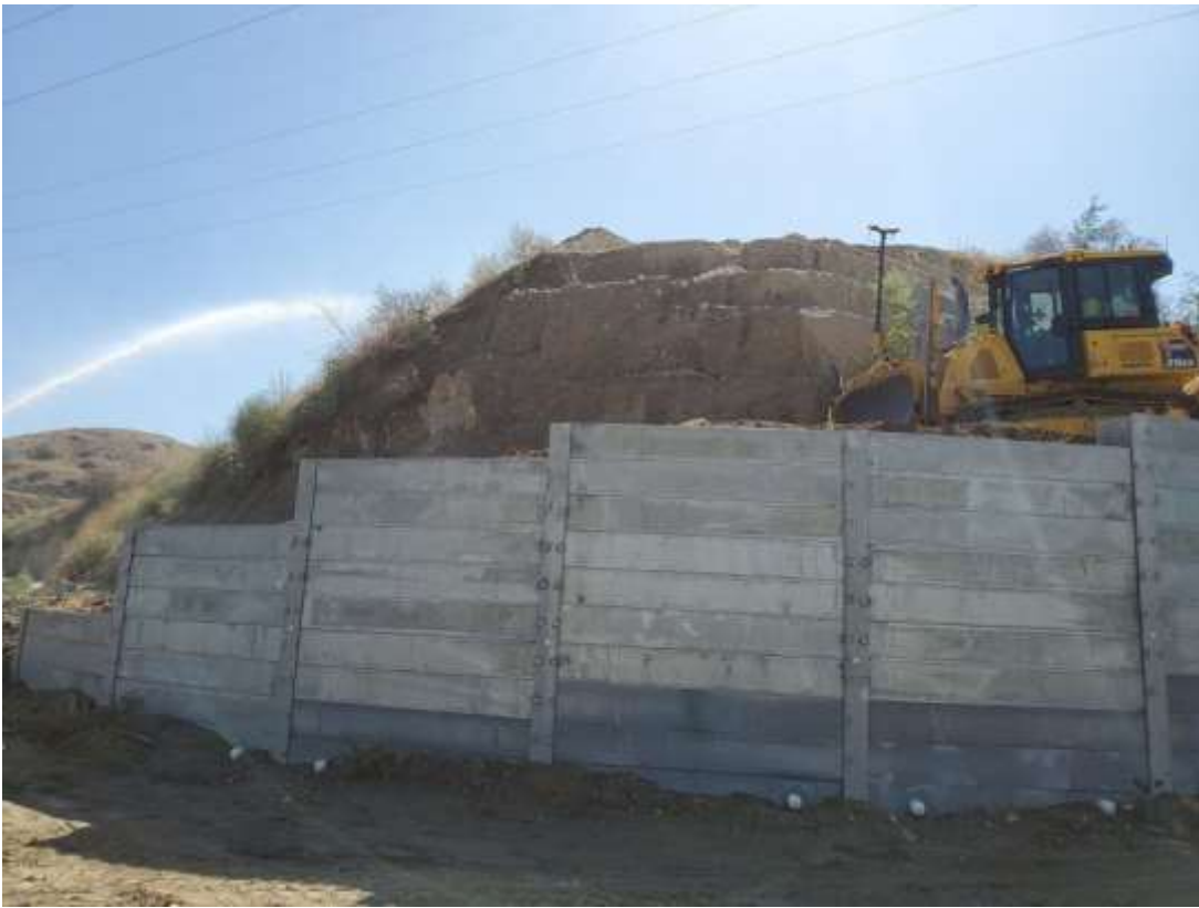
Photo 3 – Grading activities at Construction Area 3X36, Segment 3 (October 9, 2019).
