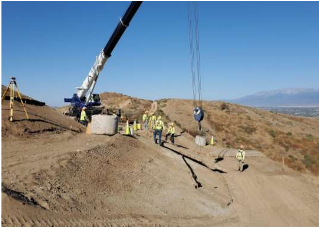
Photo 2 – Foundation activities at Construction Area 2N12, Segment 2 (October 7, 2019).
