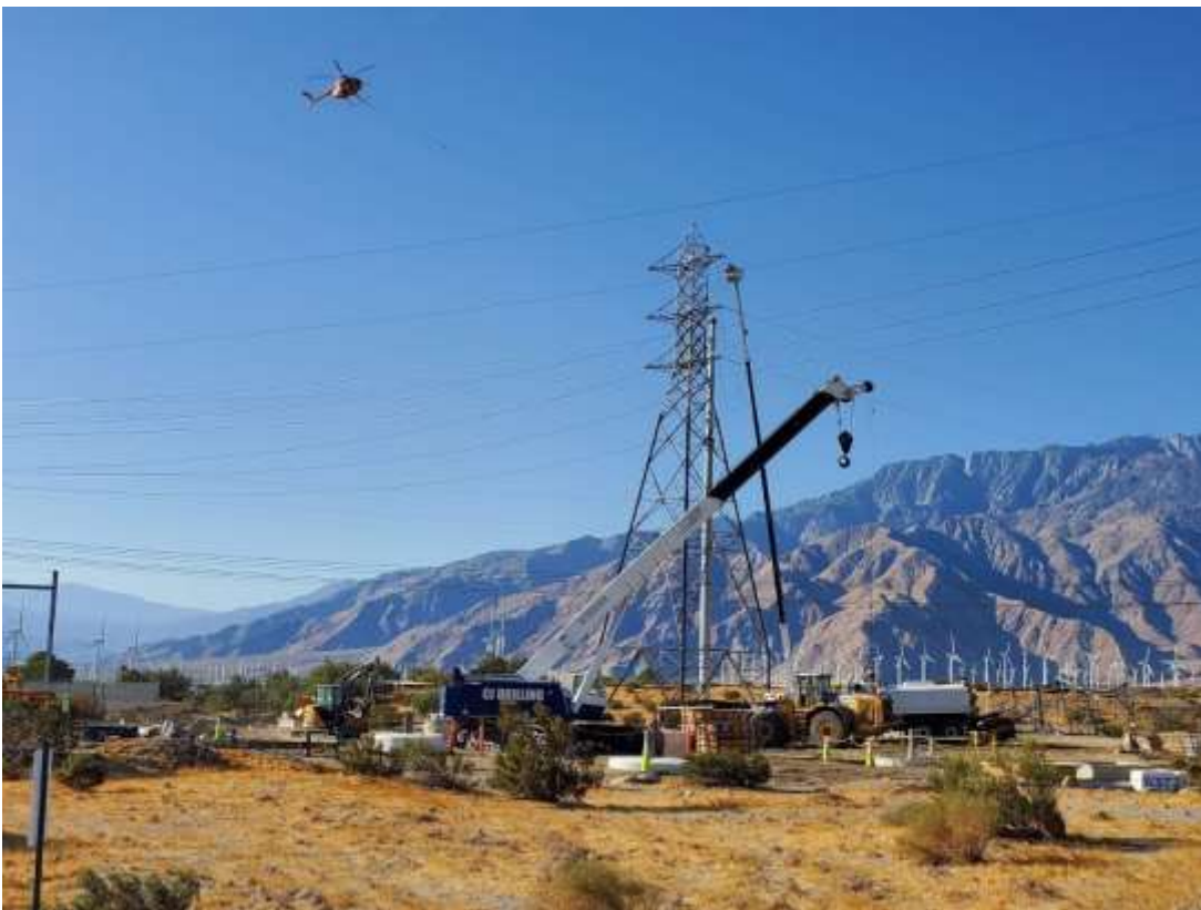
Photo 4 – Wire stringing activities at Construction Area 6S10, Segment 6 (October 8, 2016).
