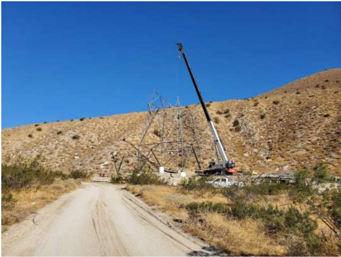
Photo 5 – Tower Assembly at Construction Area 6S31A, Segment 6 (October 8, 2019).
