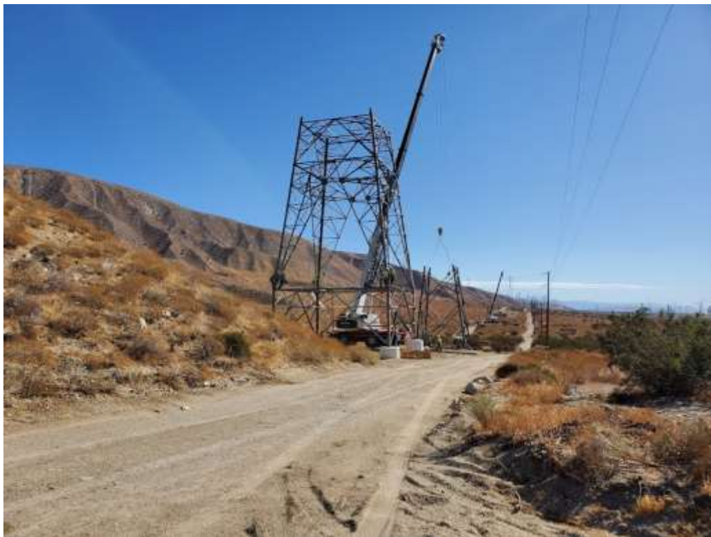
Photo 4 – Tower assembly at Construction Area 6S36, Segment 6 (October 17, 2016).
