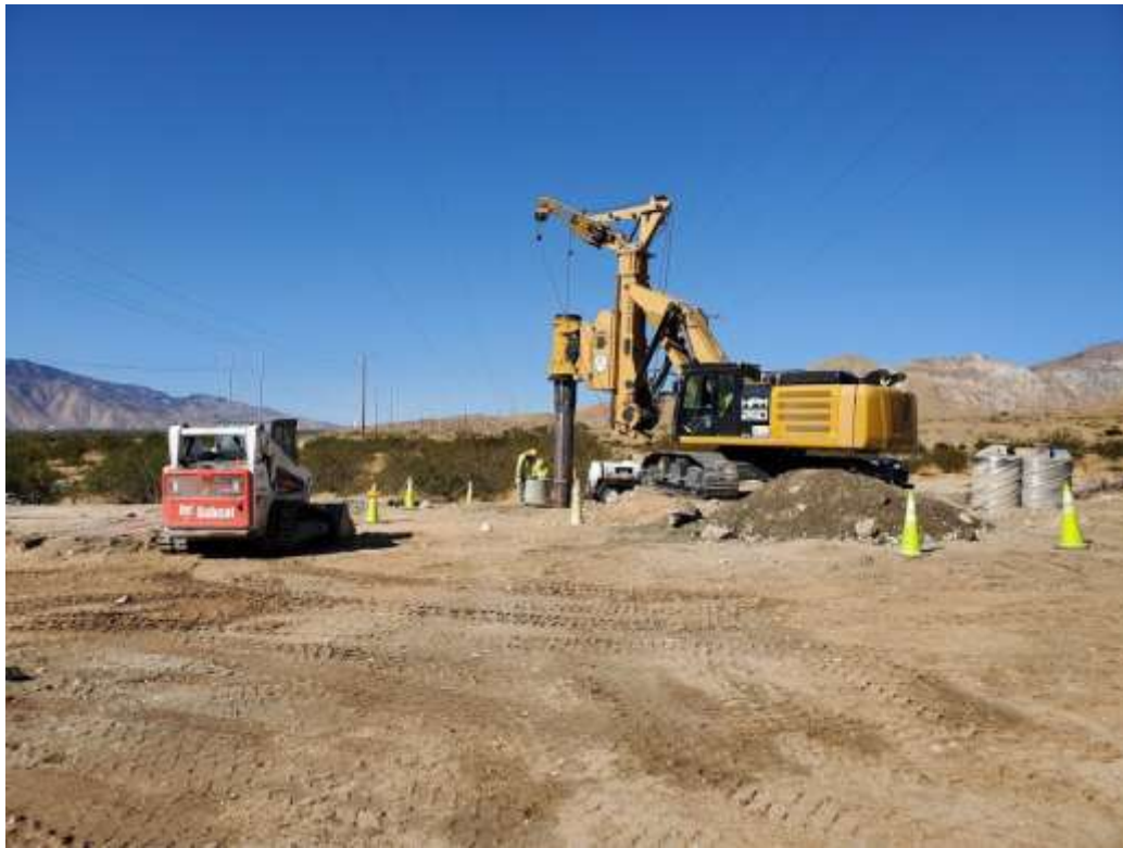
Photo 3 – Foundation activities at Construction Area 5X03, Segment 5 (October 17, 2019).
