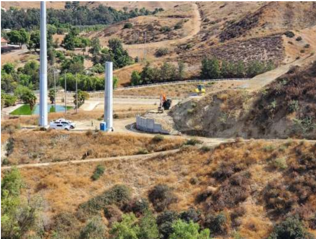
Photo 2 – Grading activities at Construction Area 3X36, Segment 3 (October 16, 2019).
