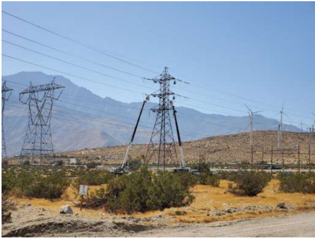
Photo 5 – Wire stringing activities on Segment 6 (October 14, 2019).
