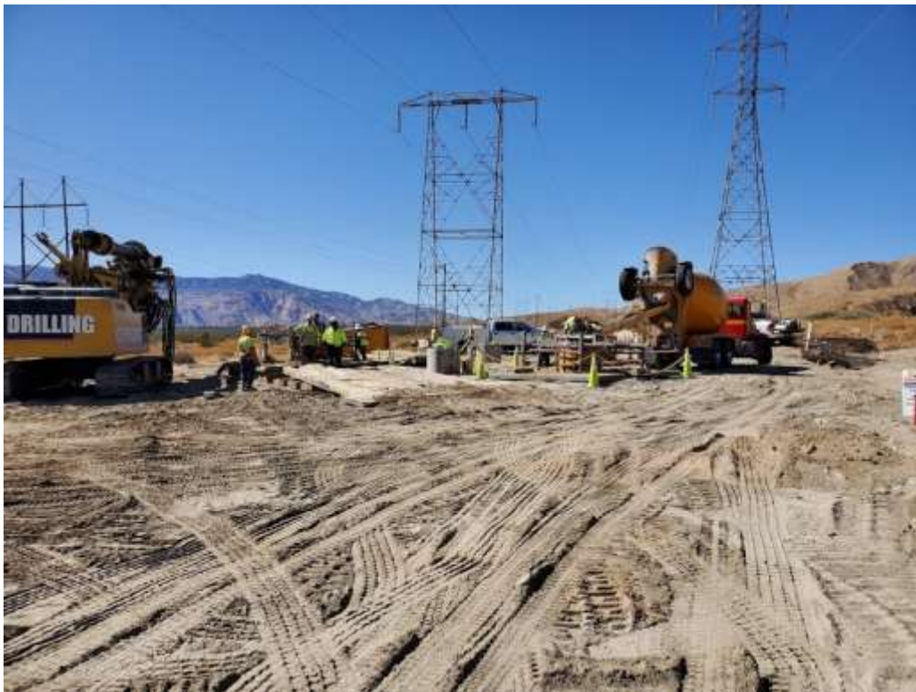
Photo 2 – Foundation activities at Construction Area 5X04, Segment 5 (October 28, 2019).
