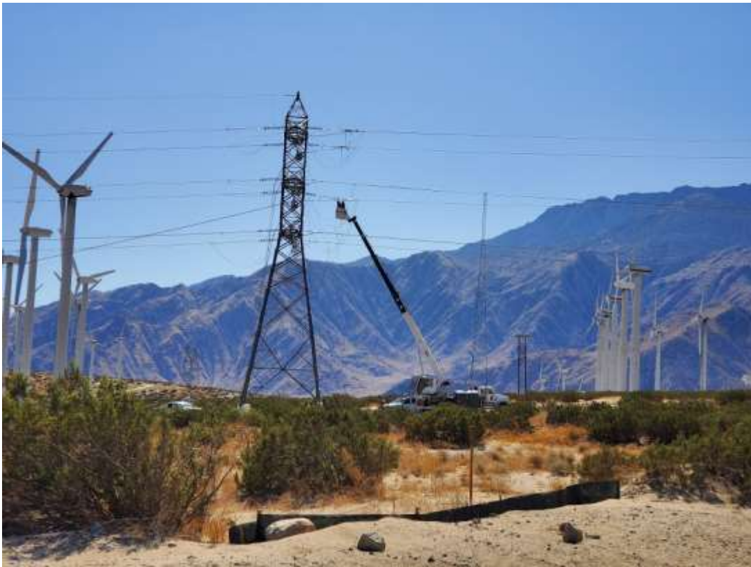
Photo 3 – Wire stringing activities at Construction Area 6S26, Segment 6 (October 28, 2019).
