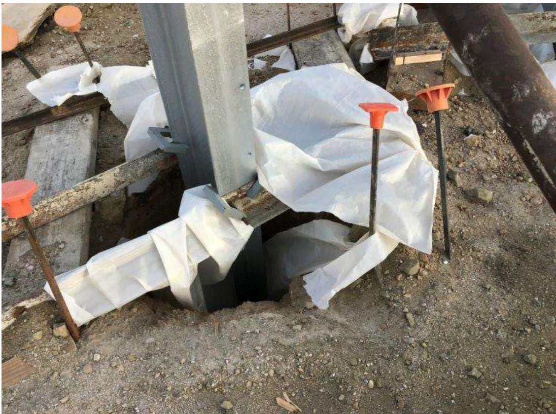
Photo 4 – Uncovered drill hole at Construction Area 4X13, Segment 4 (October 30, 2019).
