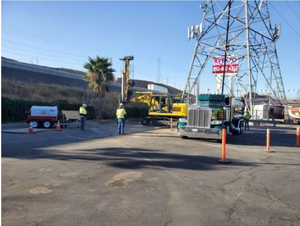
Photo 1 – Guard pole drilling at GS-2-W-2N32, Segment 2 (October 29, 2019).
