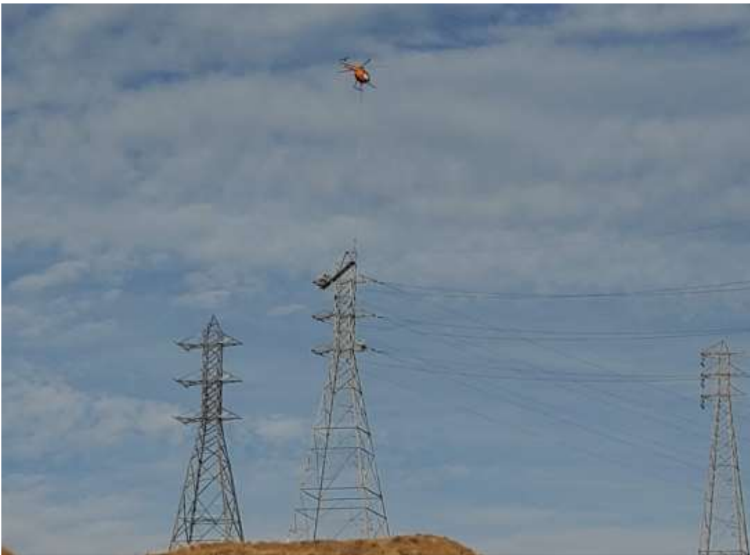
Photo 2 – Wire wreck-out activities at Construction Area 2N12, Segment 2 (November 14, 2019).
