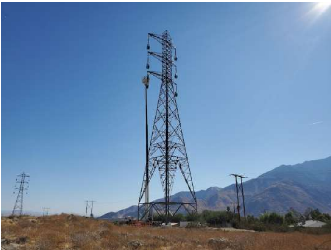
Photo 4 – Wire stringing activities at Construction Area 6S38, Segment 6 (November 11, 2019).
