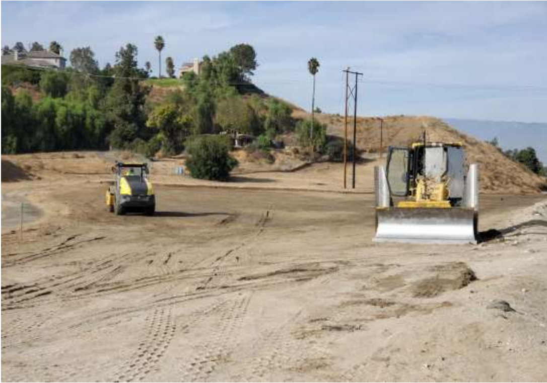
Photo 1 – Grading at Construction Area WSS-2-2N21-2N22, Segment 2 (November 14, 2019).
