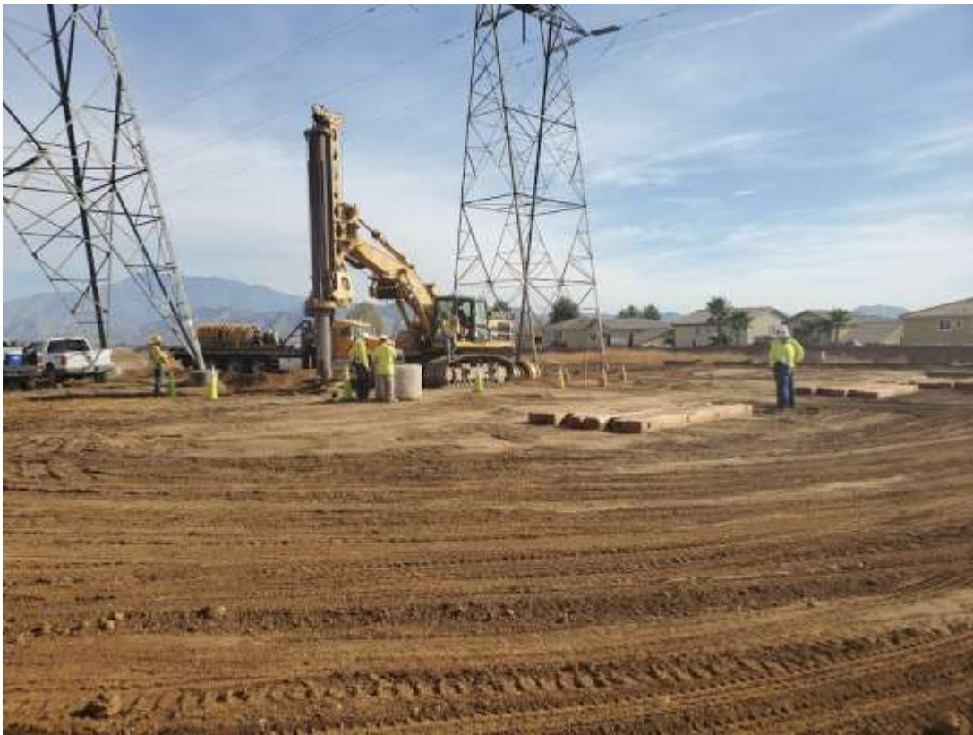
Photo 3 – Foundation activities at Construction Area 4X23, Segment 4 (November 13, 2019).
