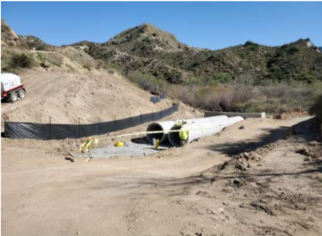
Photo 2 – Concrete crossing activities at Construction Area 4X04, Segment 4 (February 4, 2020).
