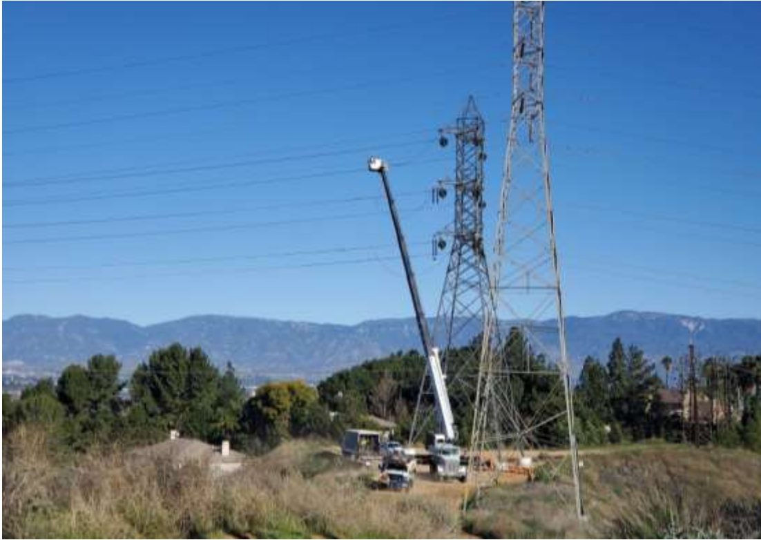
Photo 1 – Wire stringing activities at Construction Area 2N22, Segment 2 (February 4, 2020).
