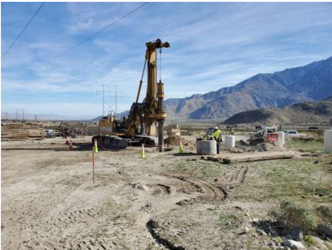
Photo 4 – Foundation activities at Construction Area 6X45, Segment 6 (February 5, 2020).
