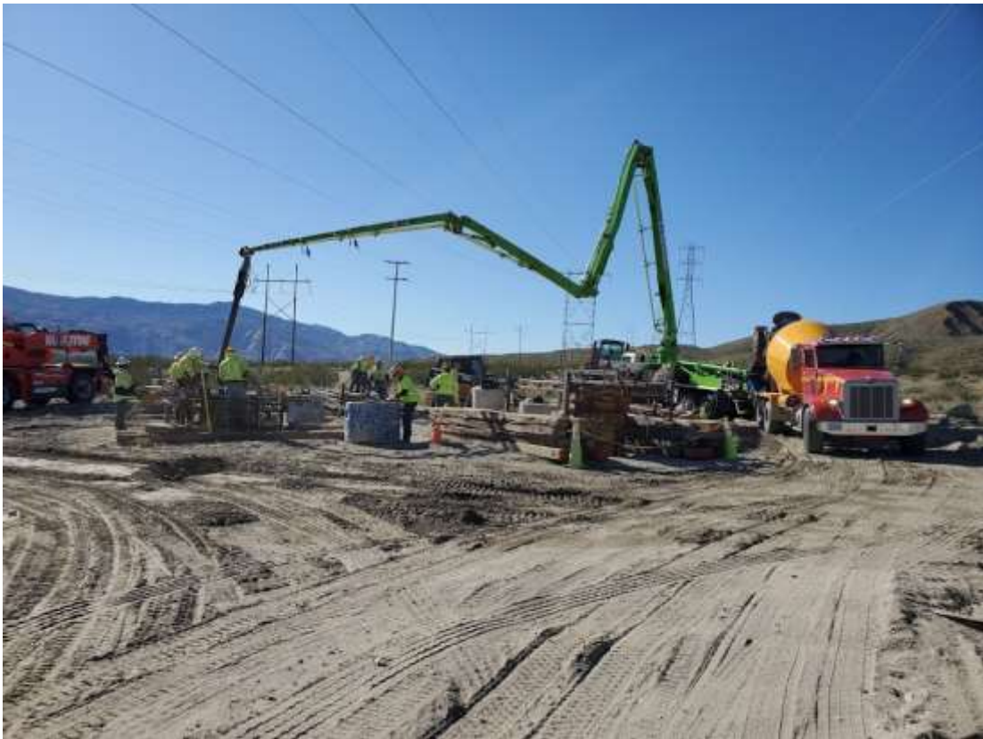
Photo 3 – Foundation activities at Construction Area 5X05, Segment 5 (February 4, 2020).
