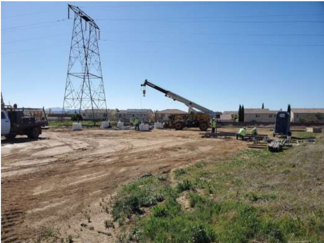
Photo 4 – Tower assembly at Construction Area 4X24, Segment 4 (February 17, 2020).
