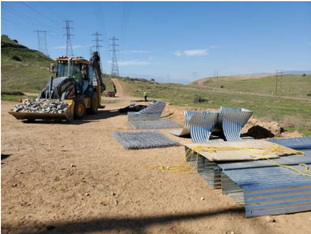
Photo 3 – MAC drain installation at Construction Area 3X60, Segment 3 (February 17, 2020).
