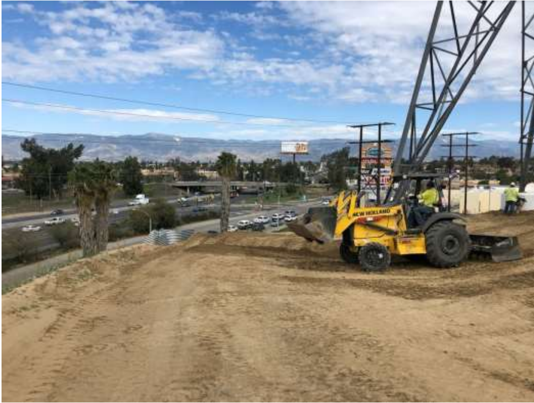
Photo 1 – Restoration grading at Construction Area 2N32 (February 21, 2020).
