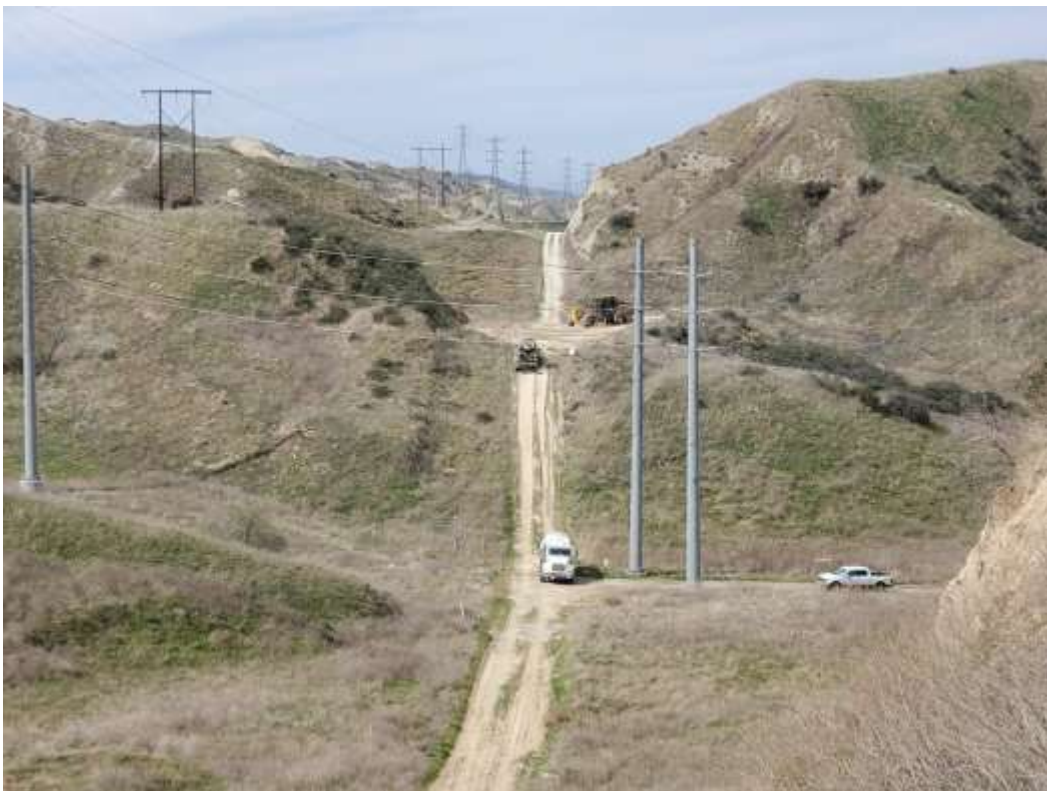
Photo 2 – Grading at Construction Area 3S03, Segment 3 (February 17, 2020).
