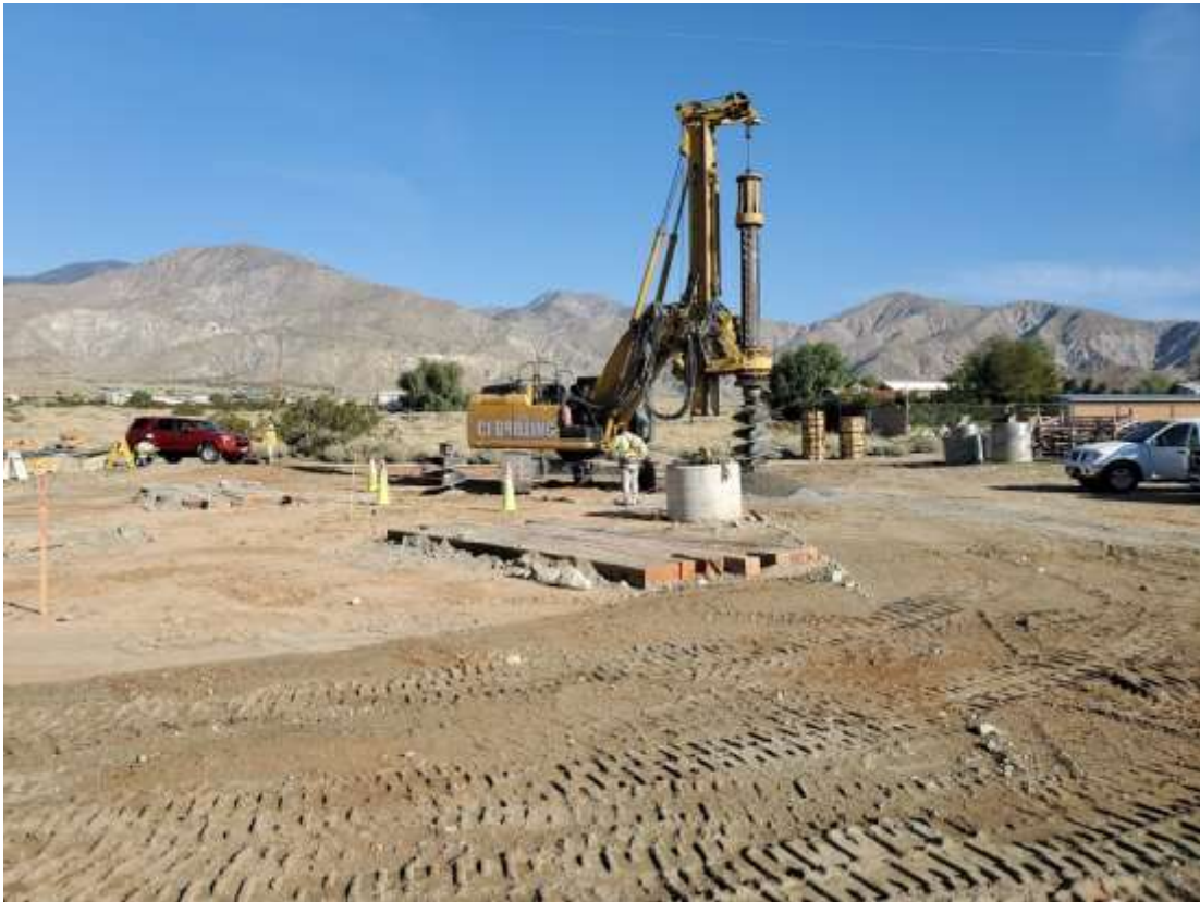
Photo 5 – Foundation activities at Construction Area 6X40, Segment 6 (February 17, 2020).
