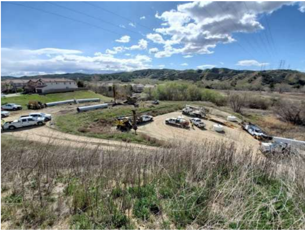
Photo 3 – Foundation activities and shoofly installation at Construction Area 4S60, Segment 4 (March 2, 2020).
