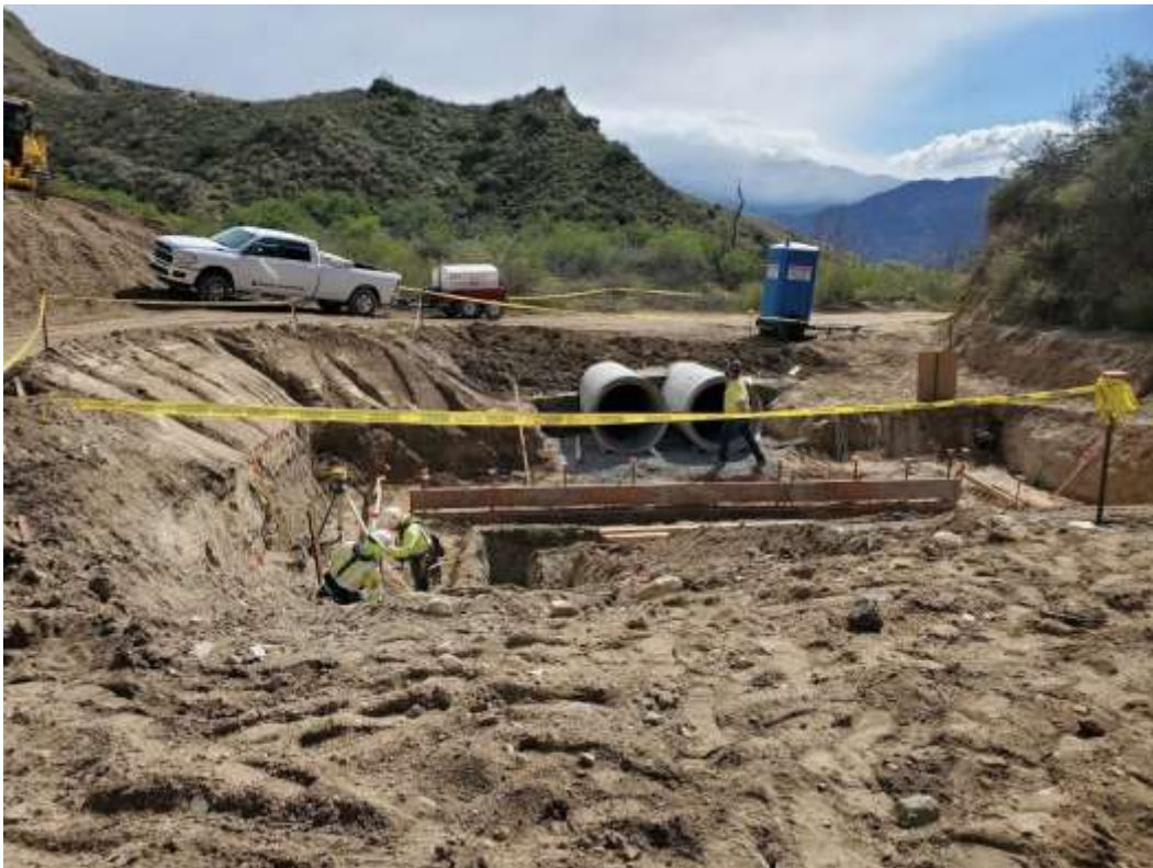
Photo 4 – Rebar installation on access road to Construction Area 4X04, Segment 4 (March 2, 2020).
