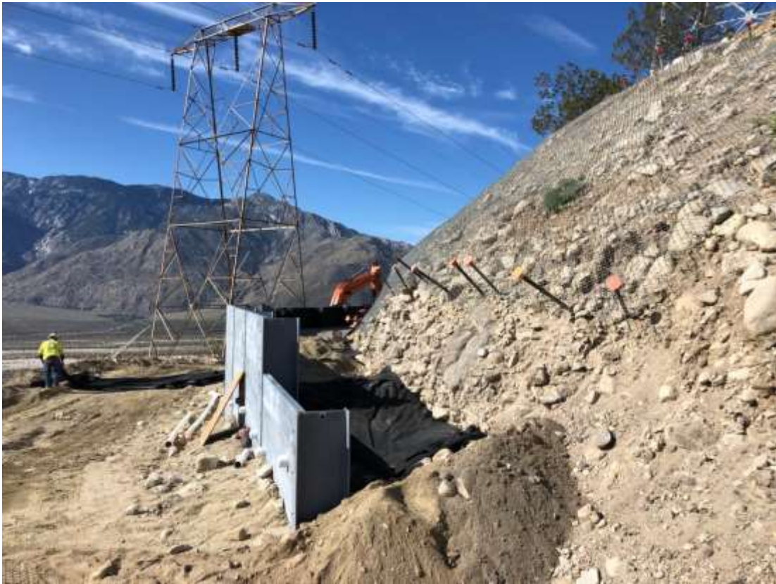
Photo 5 – Soldier pile wall construction at Construction Area 6N30, Segment 6 (March 6, 2020).
