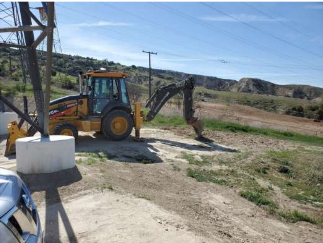
Photo 2 – Scarification at Construction Area 3X25, Segment 3 (March 4, 2020).
