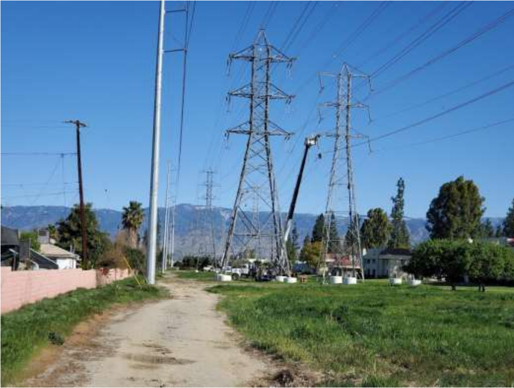
Photo 1 – Wire wreck-out preparation at Construction Areas 1E17 and 1E18, Segment 1 (March 3, 2020).
