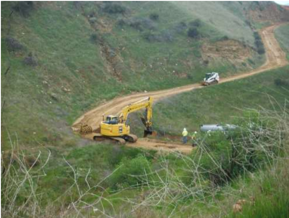
Photo 4 – Access road recontouring between Construction Areas 4X06 and 4X07, Segment 4 (March 24, 2020) (Photo courtesy of SCE).
