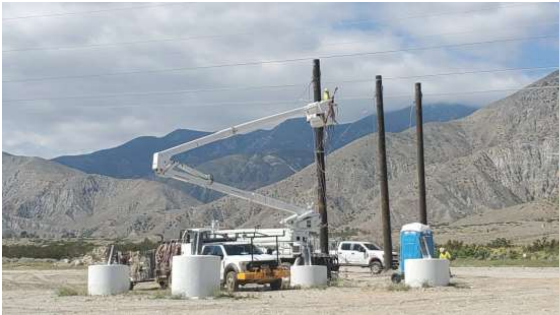
Photo 6 – Anchor installation at Construction Area 6X43, Segment 5 (March 24, 2020) (Photo courtesy of SCE).
