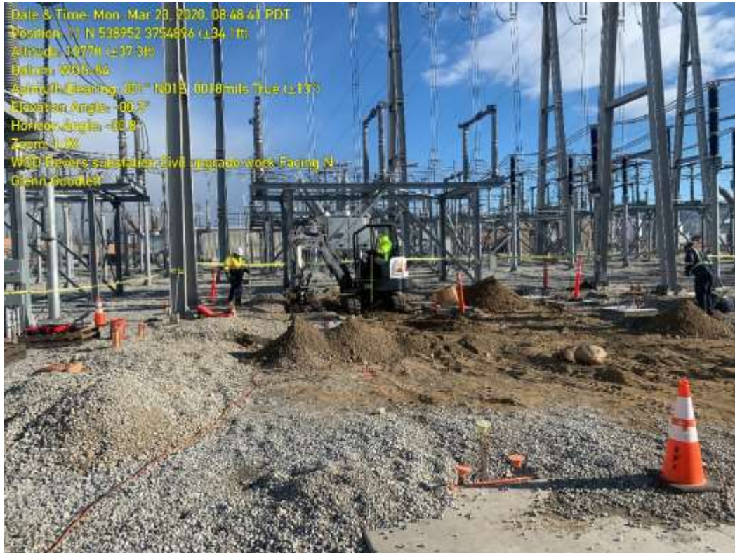
Photo 1 – Construction activities at Devers Substation (March 23, 2020) (Photo courtesy of SCE).
