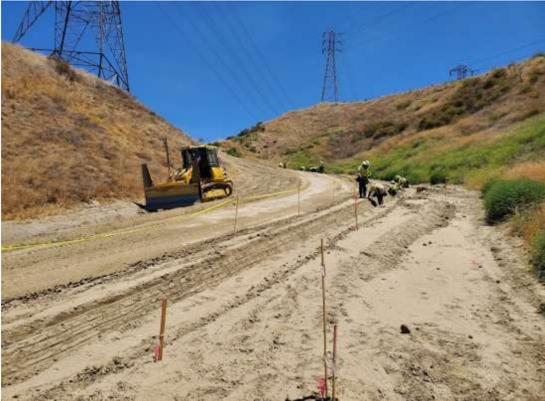
Photo 1 – V-ditch preparation activities at Construction Area 2N18, Segment 2 (June 29, 2020).
