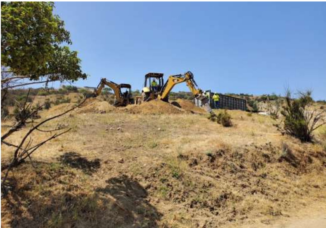
Photo 2 – Foundation wreck-out activities at Construction Area 3X25, Segment 3 (July 1, 2020).
