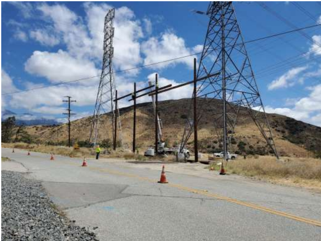
Photo 3 – Guard structure removal activities at Construction Area 4X01, Segment 4 (June 29, 2020).
