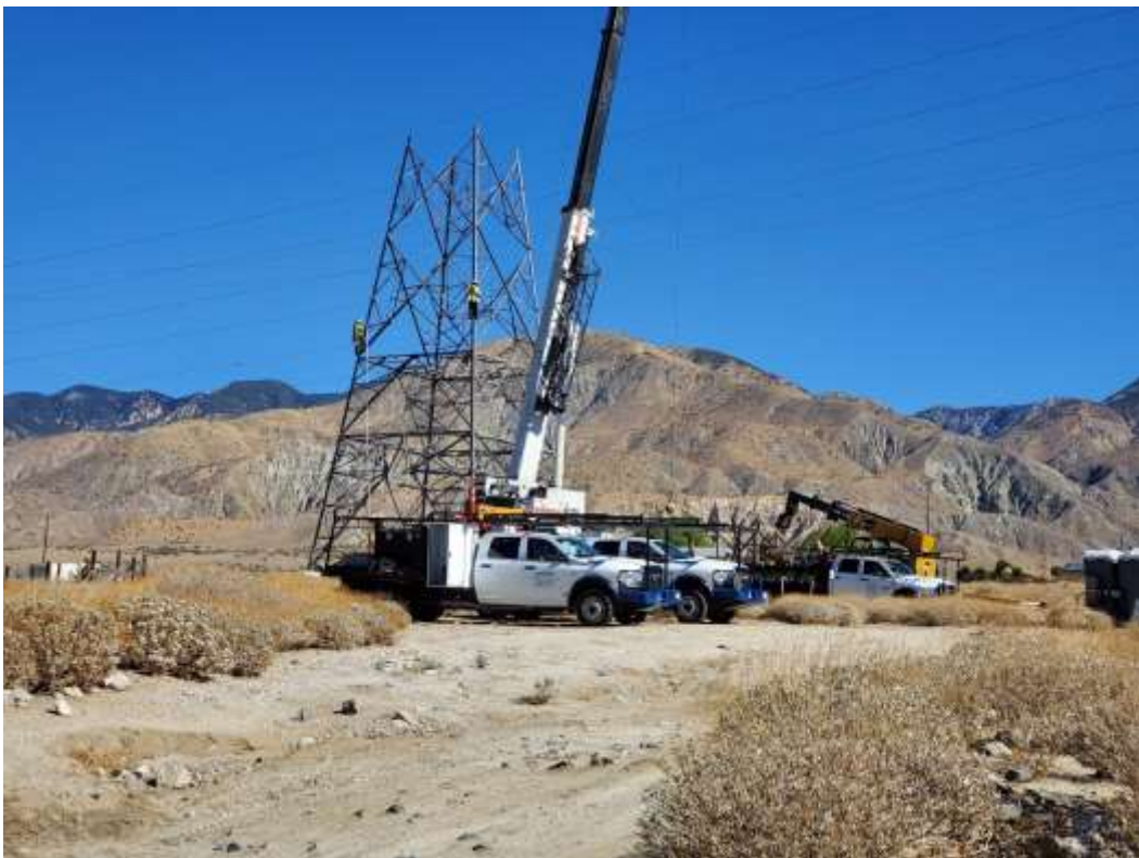
Photo 6 – Tower assembly at Construction Area 6N39, Segment 6 (July 13, 2020).
