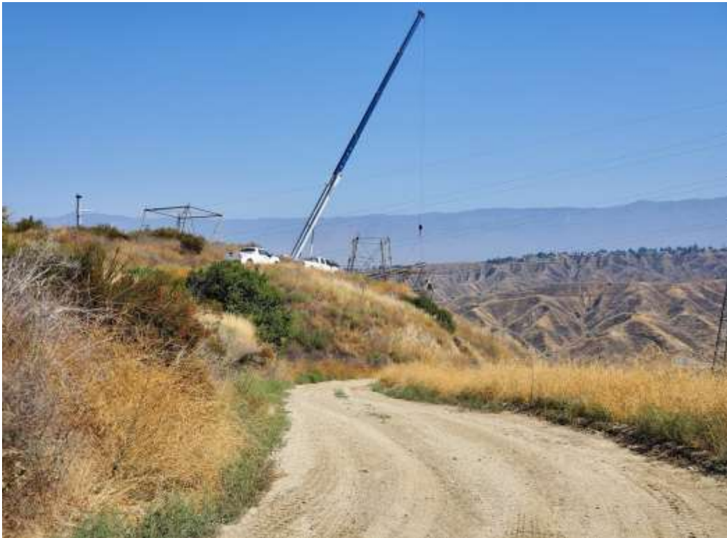
Photo 2 – Tower wreck-out activities at Construction Area 3X38, Segment 3 (July 15, 2020).
