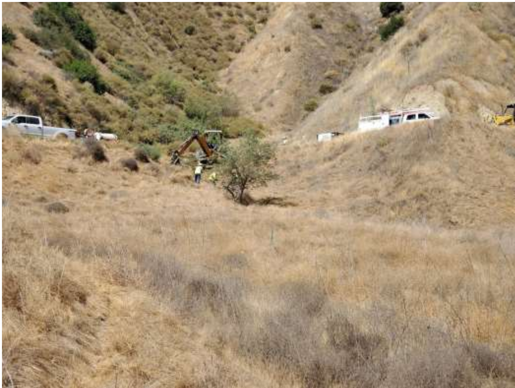
Photo 3 – MAC drain installation at Construction Area 3X31, Segment 3 (July 15, 2020).
