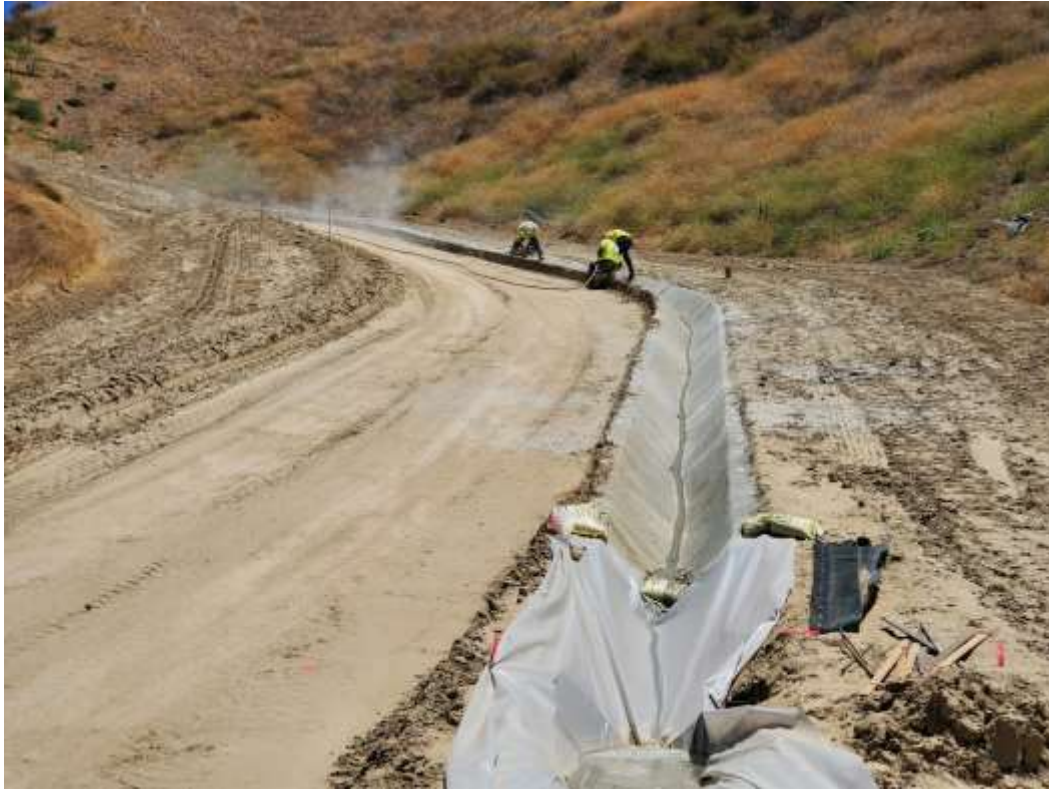
Photo 1 – V-ditch removal activities at Construction Area 2N18, Segment 2 (July 13, 2020).
