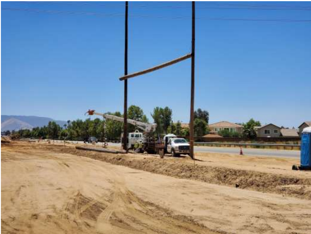
Photo 5 – Guard pole installation at Construction Area GS-4X22-4X23, Segment 4 (July 15, 2020).
