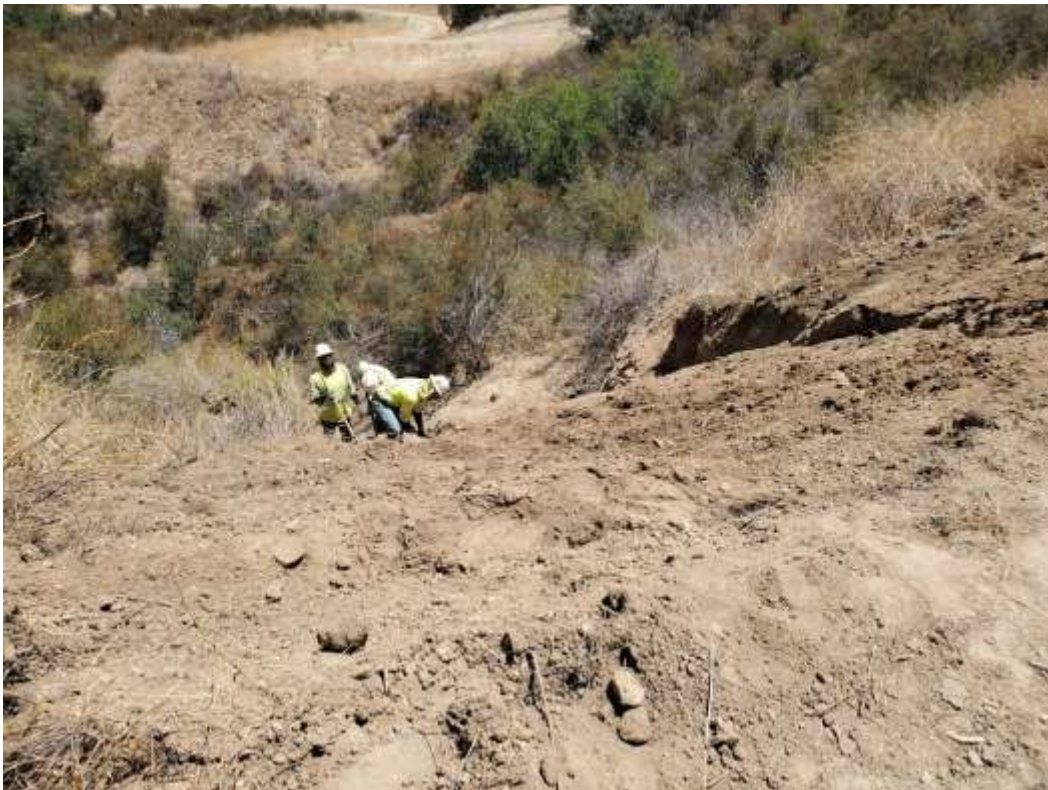
Photo 3 – MAC drain installation at Construction Area 3S02, Segment 3 (July 29, 2020).
