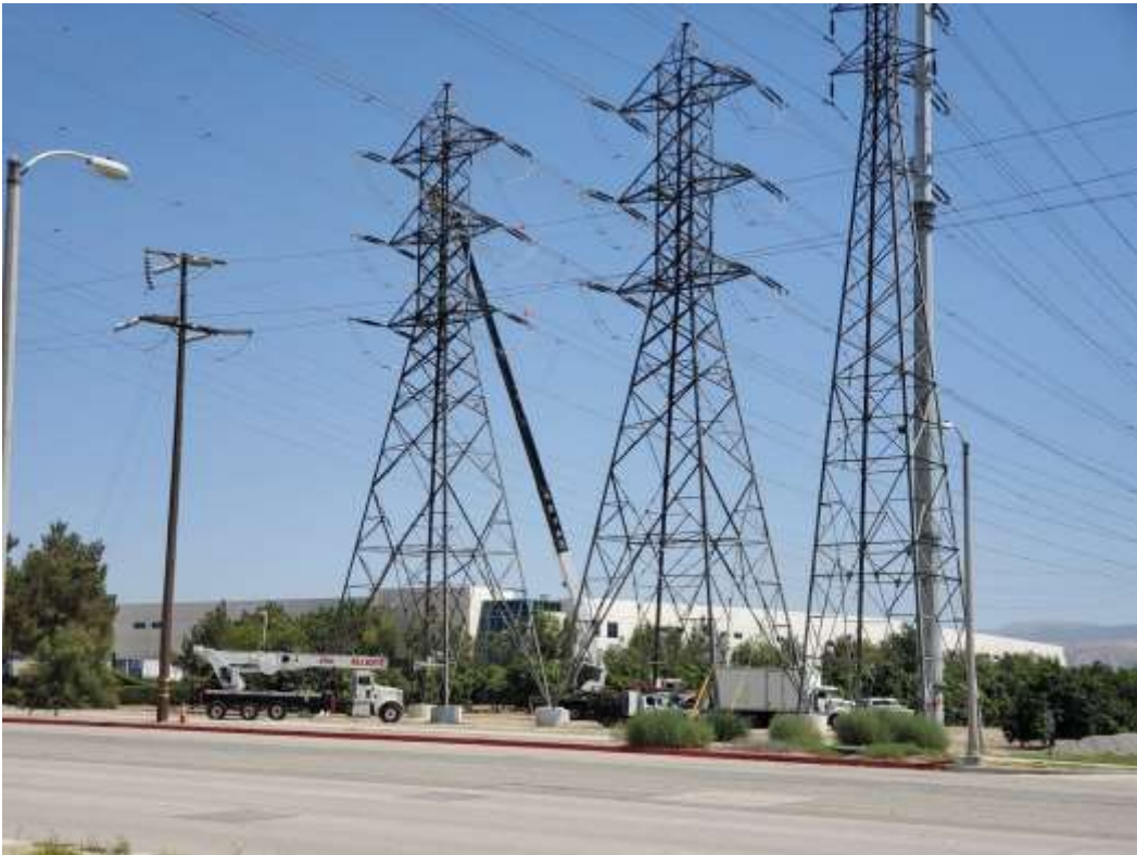
Photo 2 – Conductor re-sagging activities at Construction Area 1X25, Segment 1 (July 29, 2020).
