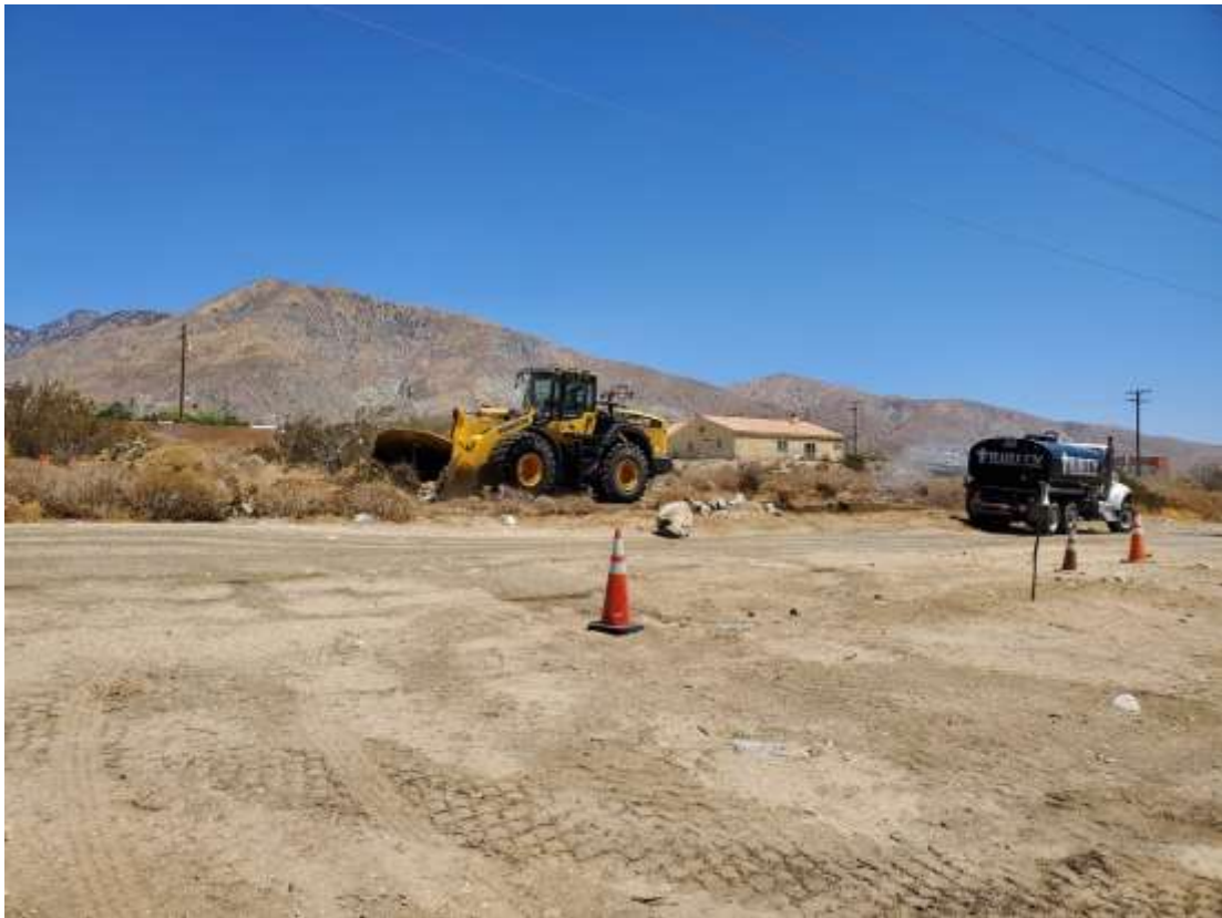
Photo 5 – Vegetation clearing at Construction Area 5X01, Segment 5 (July 28, 2020).
