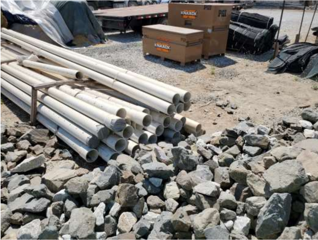
Photo 1 – Uncovered construction pipes within the Poultry MY (August 3, 2020).
