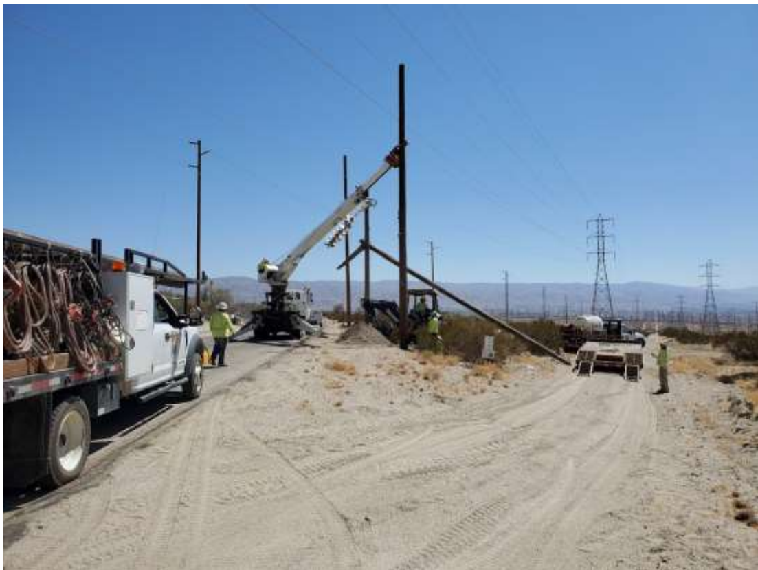
Photo 6 – Guard pole installation at Construction Area GS-6N20-6N21-1, Segment 6 (July 27, 2020).
