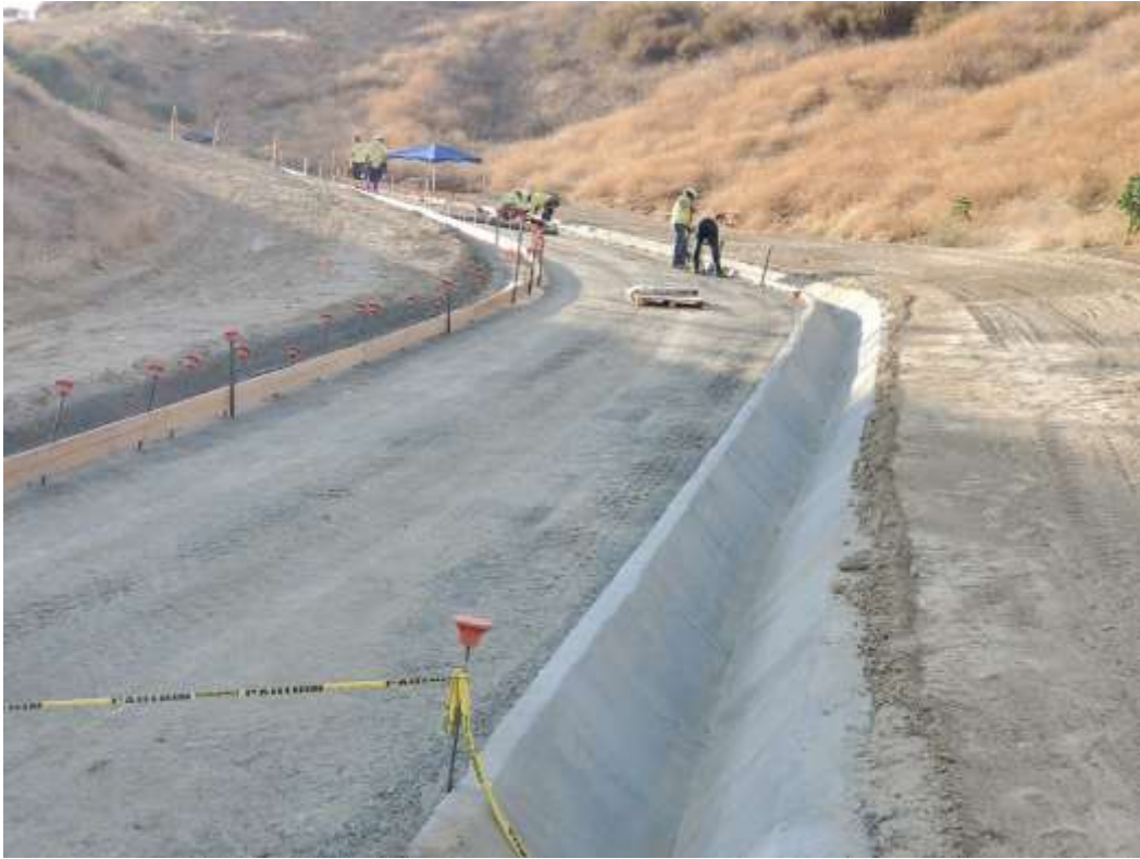
Photo 1 – Rebar installation activities at Construction Area 2N18 (August 18, 2020).
