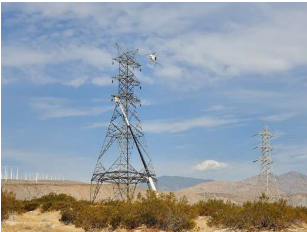
Photo 5 – Wire stringing activities at Construction Area 6N27, Segment 6 (August 17, 2020).
