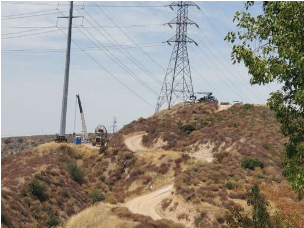
Photo 2 – Foundation activities at Construction Area 4X03, Segment 4 (August 17, 2020).
