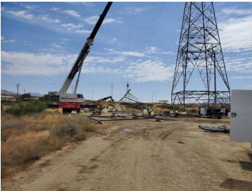
Photo 4 – Tower assembly at Construction Area 5X27, Segment 5 (August 17, 2020).
