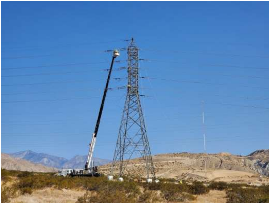
Photo 5 – Wire stringing activities at Construction Area 6N26, Segment 6 (August 24, 2020).
