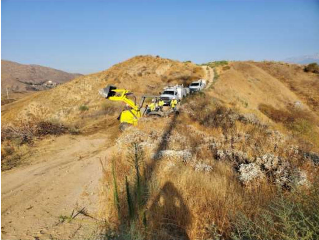
Photo 1 – MAC drain installation activities at Construction Area 2N12 (August 25, 2020).
