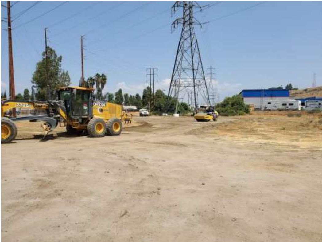
Photo 2 – Site restoration and compaction activities at Construction Area 2N35, Segment 2 (August 24, 2020).
