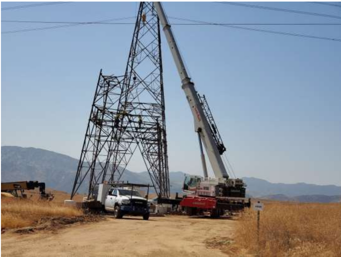
Photo 3 – Tower assembly at Construction Area 4X09, Segment 4 (August 24, 2020).
