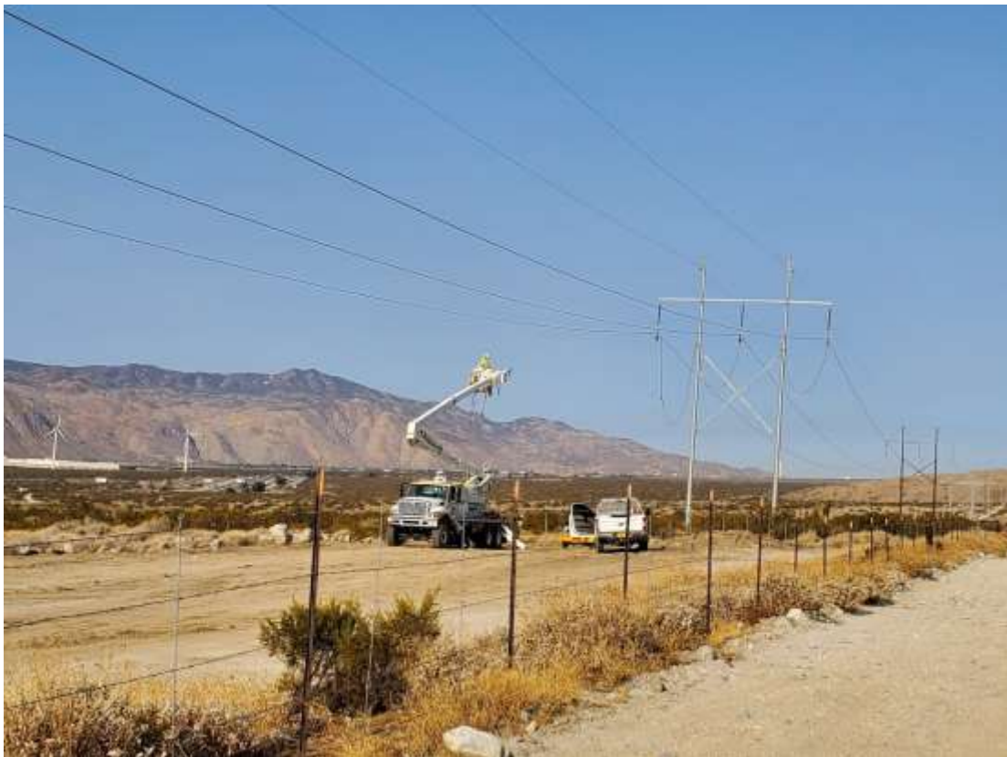
Photo 4 – Wire wreck-out activities at Construction Area 5X01, Segment 5 (August 26, 2020).
