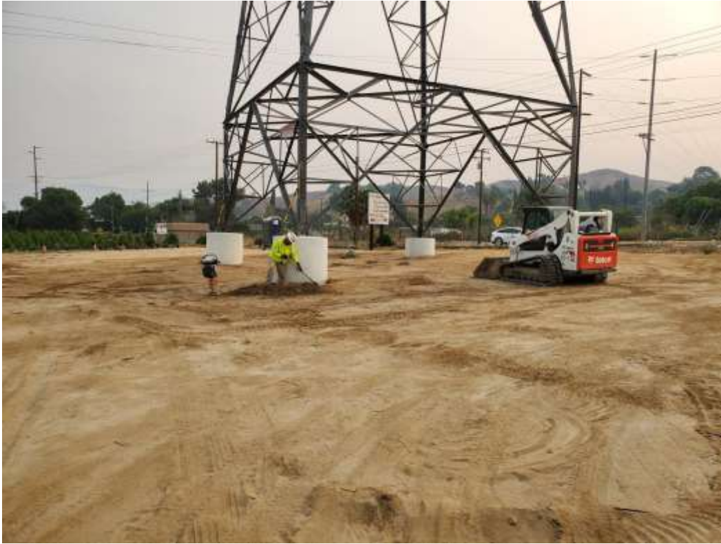
Photo 1 – Site restoration activities at Construction Area 2N21, Segment 2 (September 11, 2020).
