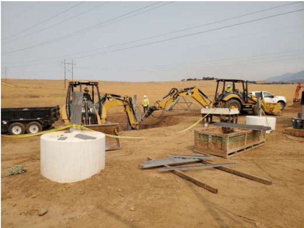
Photo 3 – Foundation wreck-out at Construction Area 4N07, Segment 4 (September 11, 2020).
