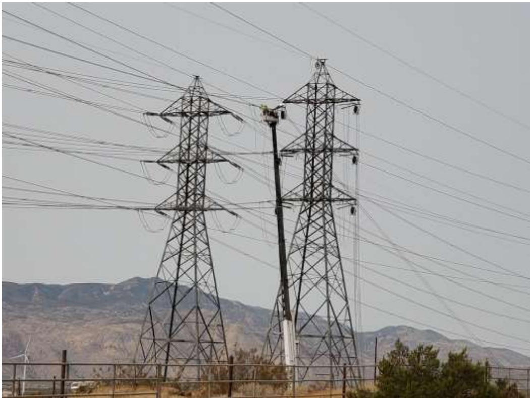
Photo 6 – Wire stringing activities at Construction Area 5X01, Segment 5 (September 11, 2020).
