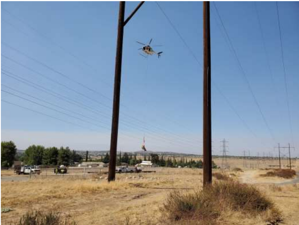
Photo 5 – Helicopter operations at Construction Area 4X14, Segment 4 (September 9, 2020).
