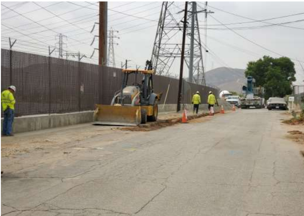
Photo 2 – Conduit installation at Construction Areas 2N36 through 2N38 (TWA-2-VistaSub-MPR-37), Segment 2 (September 8, 2020).
