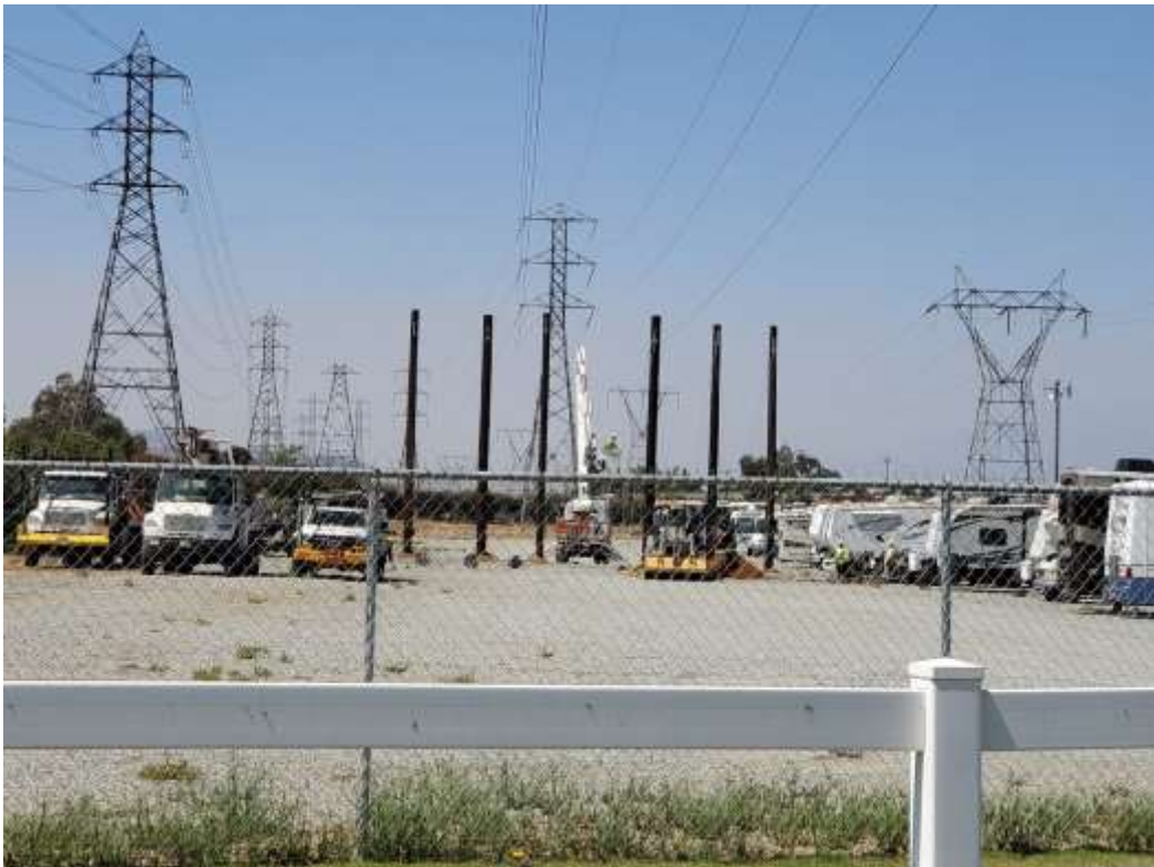
Photo 4 – Snub installation activities at Construction Area WSS-4X44-4X45, Segment 4 (September 9, 2020).
