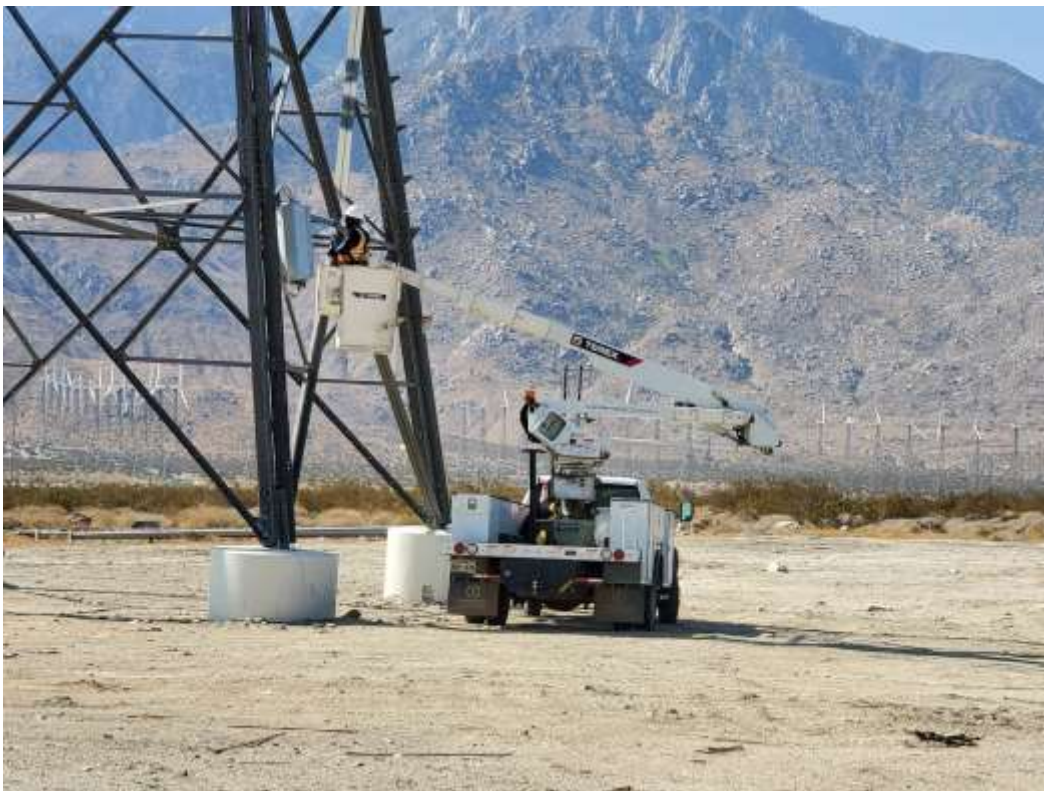
Photo 6 – Fiber splicing activities at Construction Area 6N42, Segment 6 (September 23, 2020).
