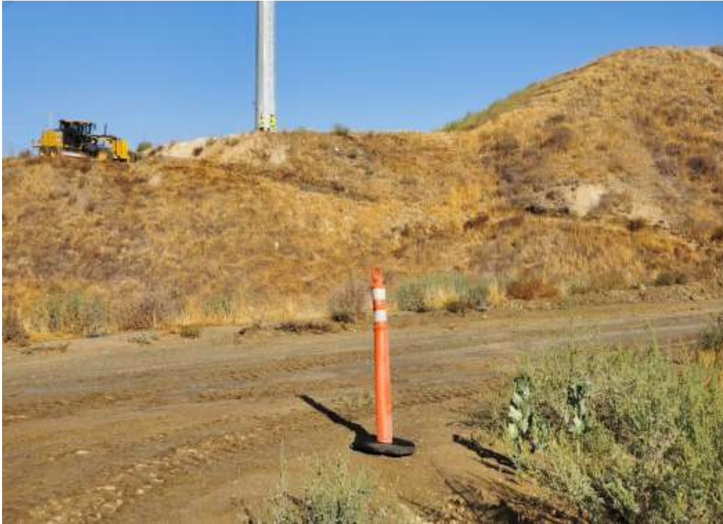
Photo 1 – Site restoration activities at Construction Area 2N15, Segment 2 (September 22, 2020).
