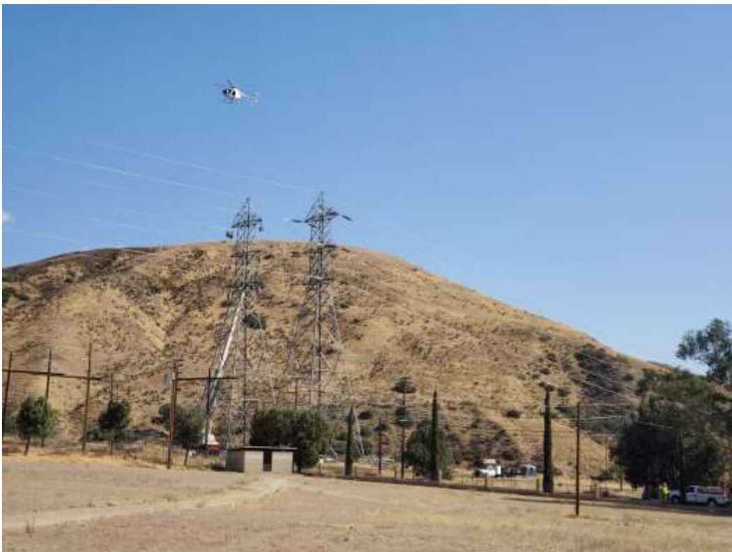
Photo 4 – Wire stringing activities at Construction Area 4X01, Segment 4 (September 21, 2020).
