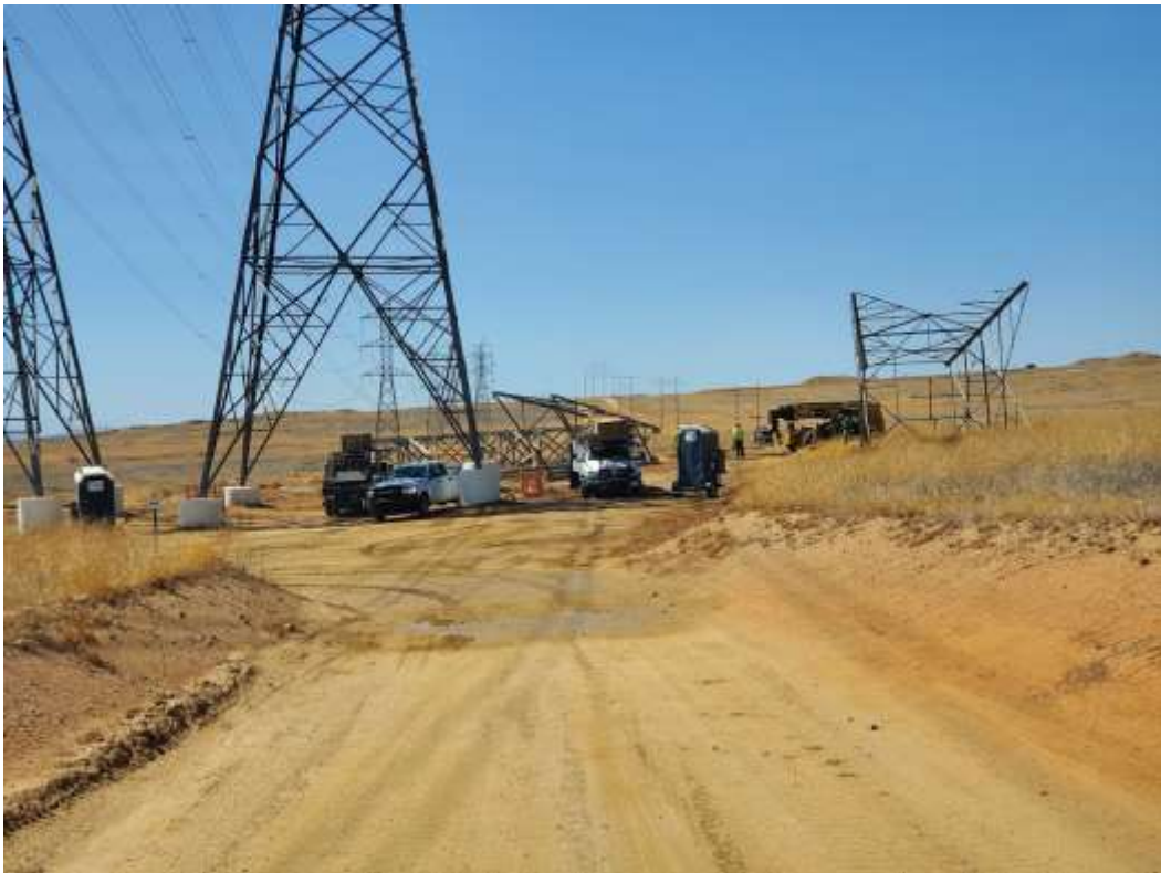
Photo 3 – Tower wreck-out activities at Construction Area 4X06, Segment 4 (September 22, 2020).
