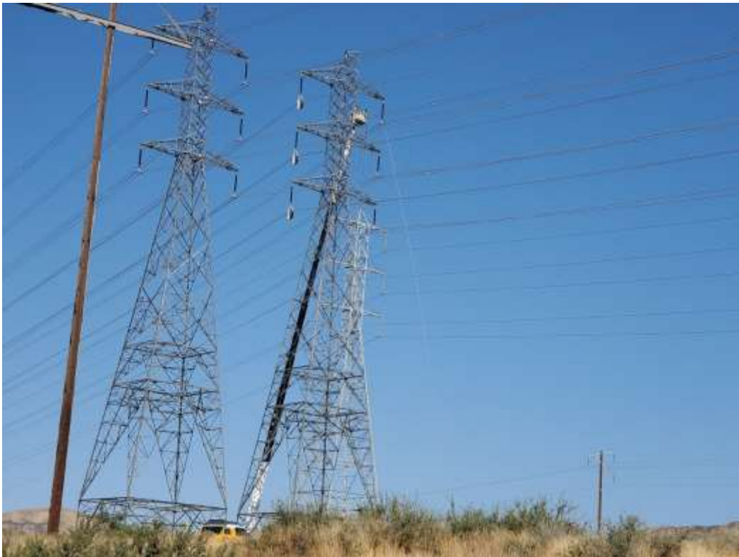
Photo 5 – Wire stringing activities at Construction Area 5X24, Segment 5 (September 21, 2020).
