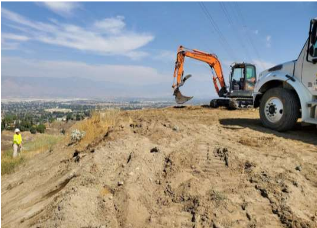
Photo 2 – Site restoration activities at Construction Area 2N12, Segment 2 (October 5, 2020).
