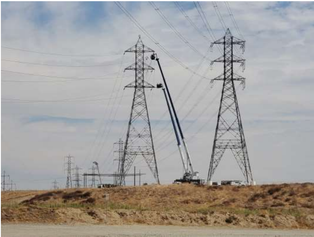
Photo 5 – Wire wreck-out activities at Construction Area 4X34, Segment 4 (October 6, 2020).
