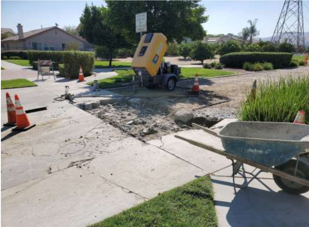
Photo 1 – Curb replacement activities at Construction Area 1X12-1X13, Segment 1 (October 7, 2020).
