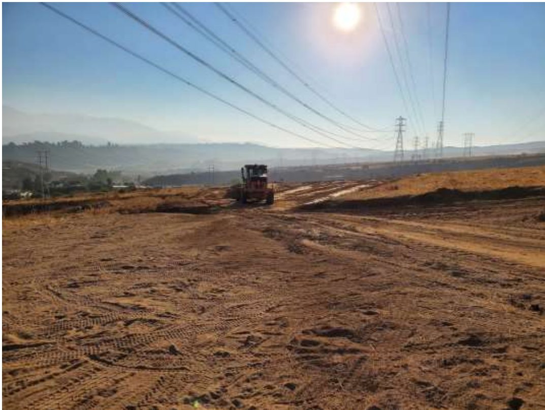
Photo 4 –Grading activities at Construction Area 3X59, Segment 3 (October 7, 2020).
