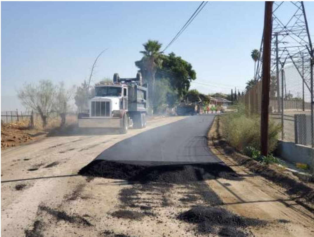
Photo 3 – Road paving activities at Construction Area TWA-2-VistaSub-MPR-37, Segment 2 (October 7, 2020).
