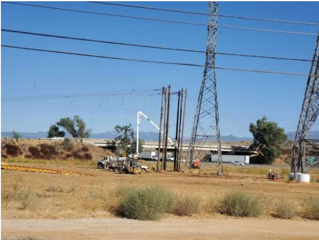
Photo 3 – Wire wreck-out activities at Construction Area 4X45, Segment 4 (October 13, 2020).
