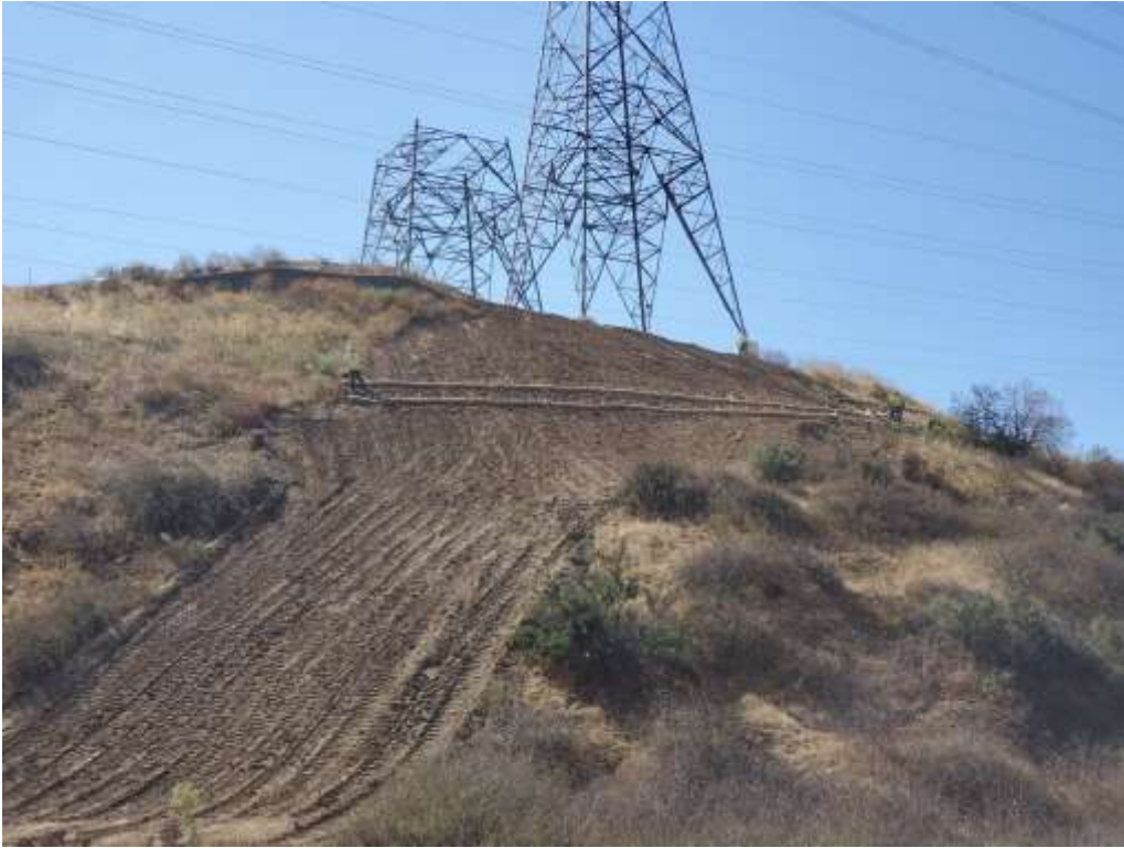
Photo 1 – BMP installation at Construction Area WA-3-3N64-MPR-38, Segment 3 (October 14, 2020).
