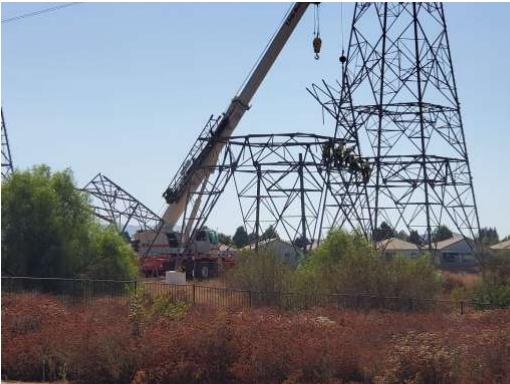
Photo 2 – Tower assembly at Construction Area 4X41, Segment 4 (October 14, 2020).
