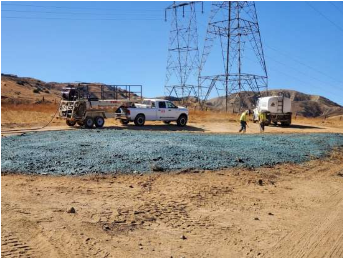
Photo 3 – Hydroseed application at Construction Area 3X56, Segment 3 (October 29, 2020).
