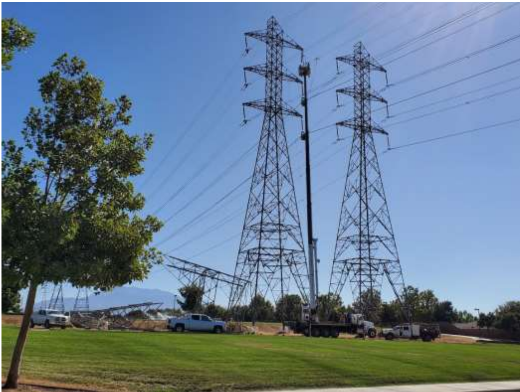
Photo 5 – Wire stringing activities at Construction Area 4X43, Segment 4 (October 27, 2020).
