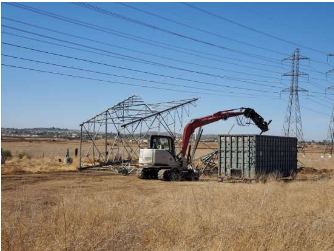
Photo 4 – Tower wreck-out at Construction Area M20-T3, Segment 4 (October 27, 2020).
