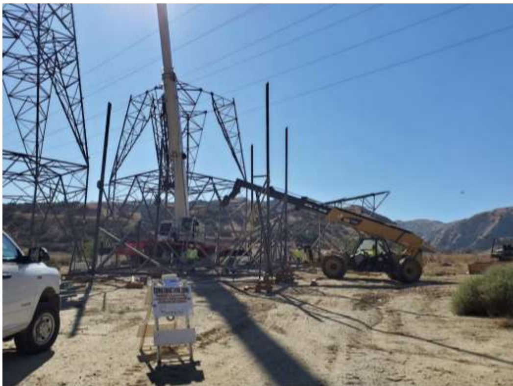
Photo 2 – Assembly at Construction Area 3X29, Segment 3 (October 28, 2020).
