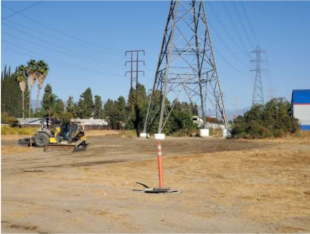
Photo 1 – Site restoration activities at Construction Area 2N35, Segment 2 (November 4, 2020).
