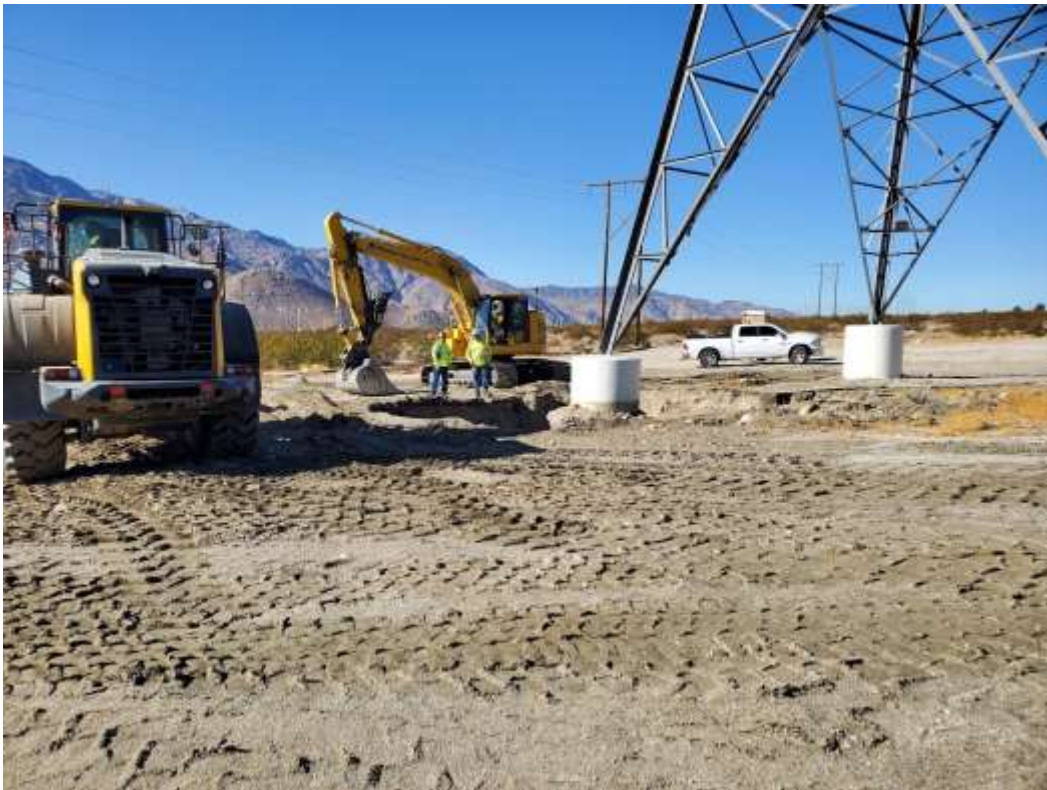
Photo 5 – Scour prevention activities at Construction Area 6X41, Segment 6 (November 4, 2020).
