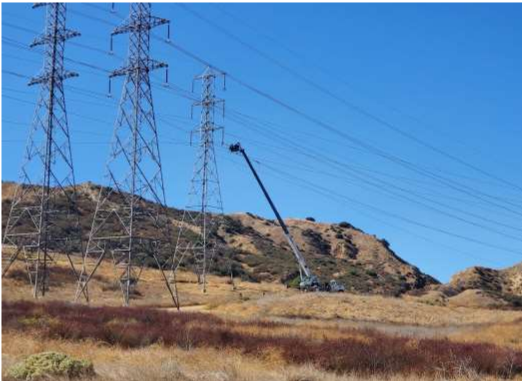
Photo 2 – Wire wreck-out activities at Construction Area 3X14, Segment 3 (November 2, 2020).
