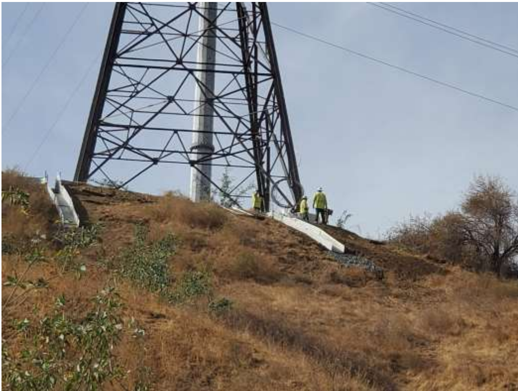
Photo 3 – MAC drain installation at Construction Area 3X65, Segment 3 (November 3, 2020).
