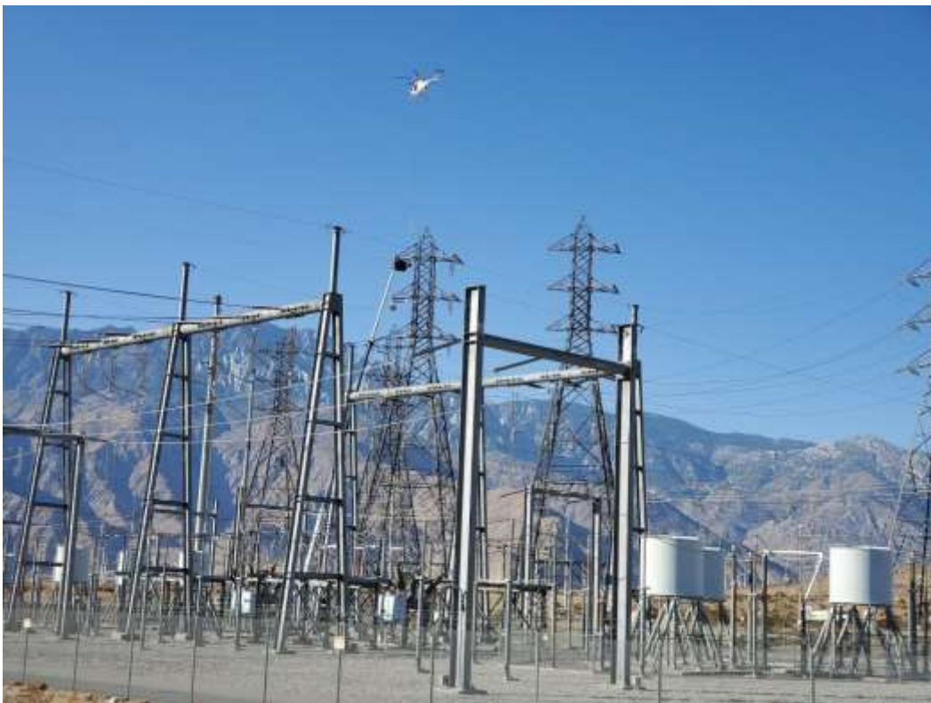
Photo 6 – Wire stringing activities at Construction Area 6X09, Segment 6 (November 4, 2020).
