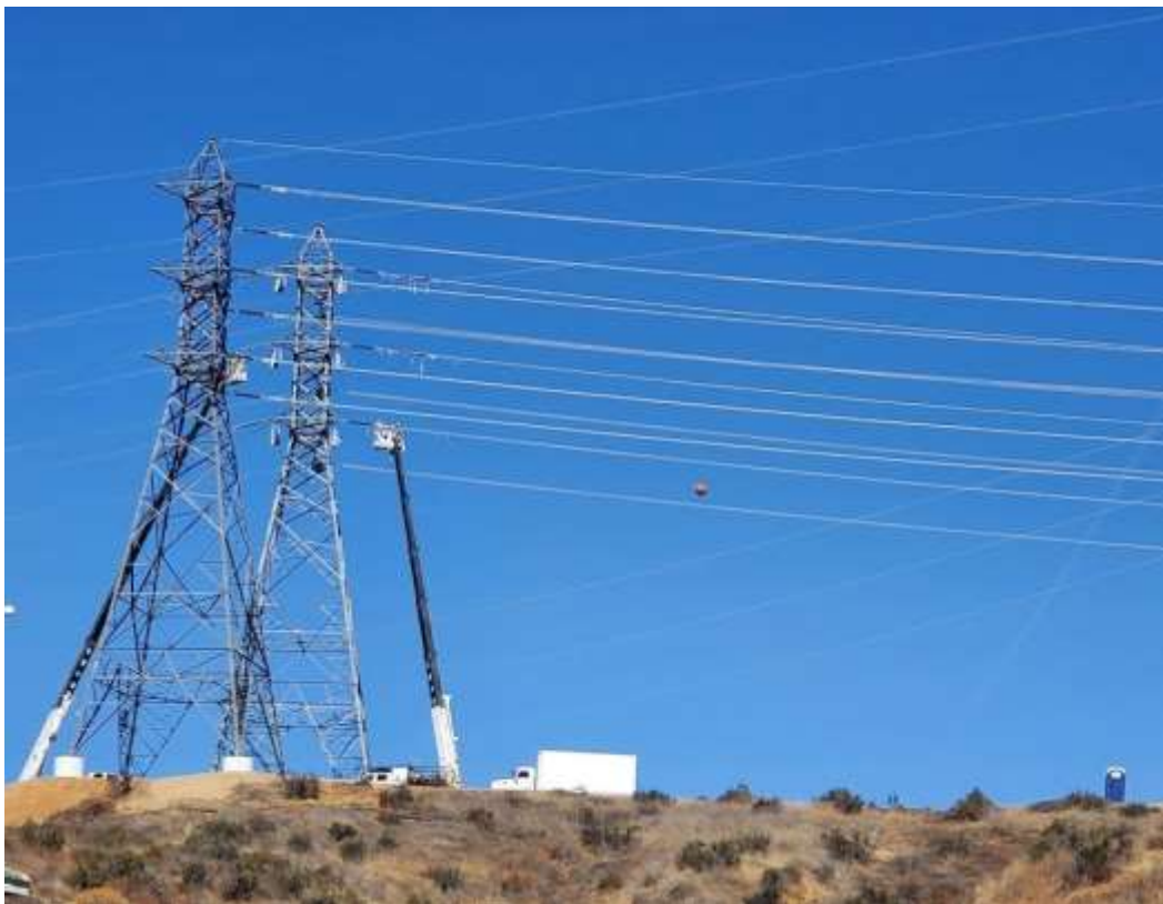
Photo 4 – Wire stringing activities at Construction Area 4X56, Segment 4 (November 2, 2020).
