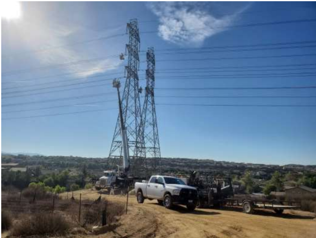
Photo 5 – Spacer installation at Construction Area 4X51, Segment 4 (November 11, 2020).
