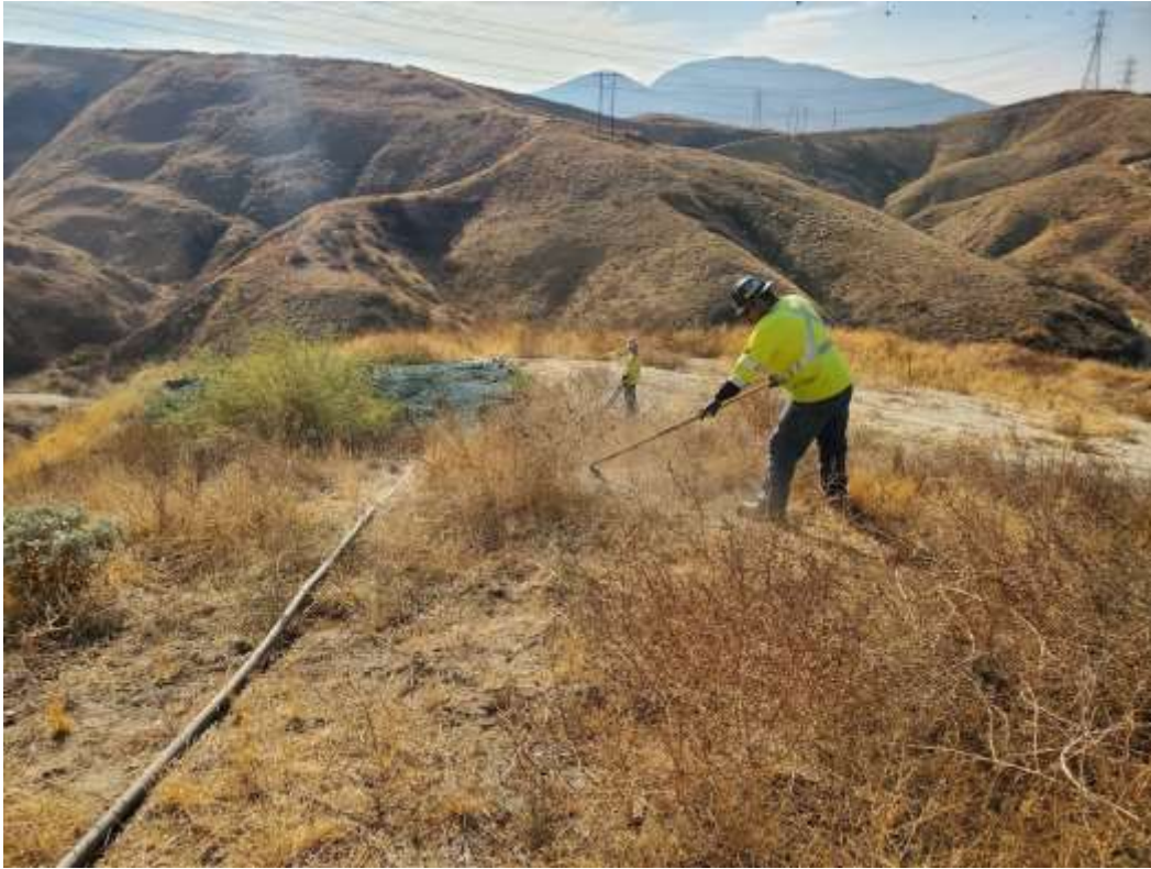
Photo 1 – Scarification and hydroseed activities at Construction Area 2N08, Segment 2 (November 12, 2020).
