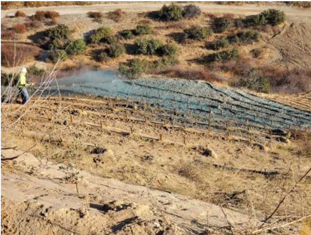
Photo 3 – Hydroseed application at Construction Area 3X64, Segment 3 (November 13, 2020).
