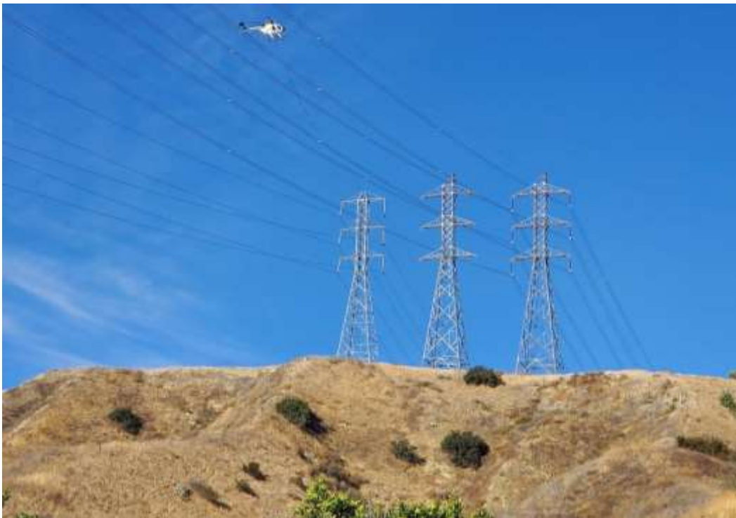
Photo 2 – Helicopter wire wreck-out activities at Construction Area 3X40, Segment 3 (November 11, 2020).
