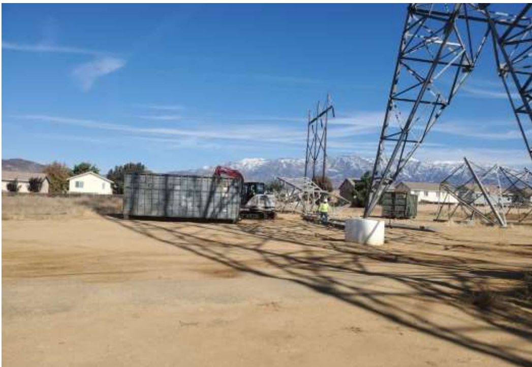
Photo 4 – Tower wreck-out activities at Construction Area 4X30, Segment 4 (November 11, 2020).
