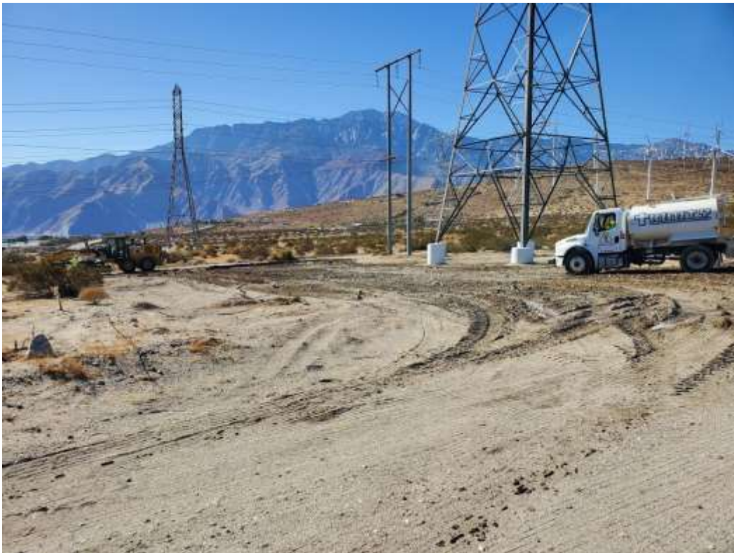
Photo 6 – Site restoration grading at Construction Area 6N16, Segment 6 (November 18, 2020).
