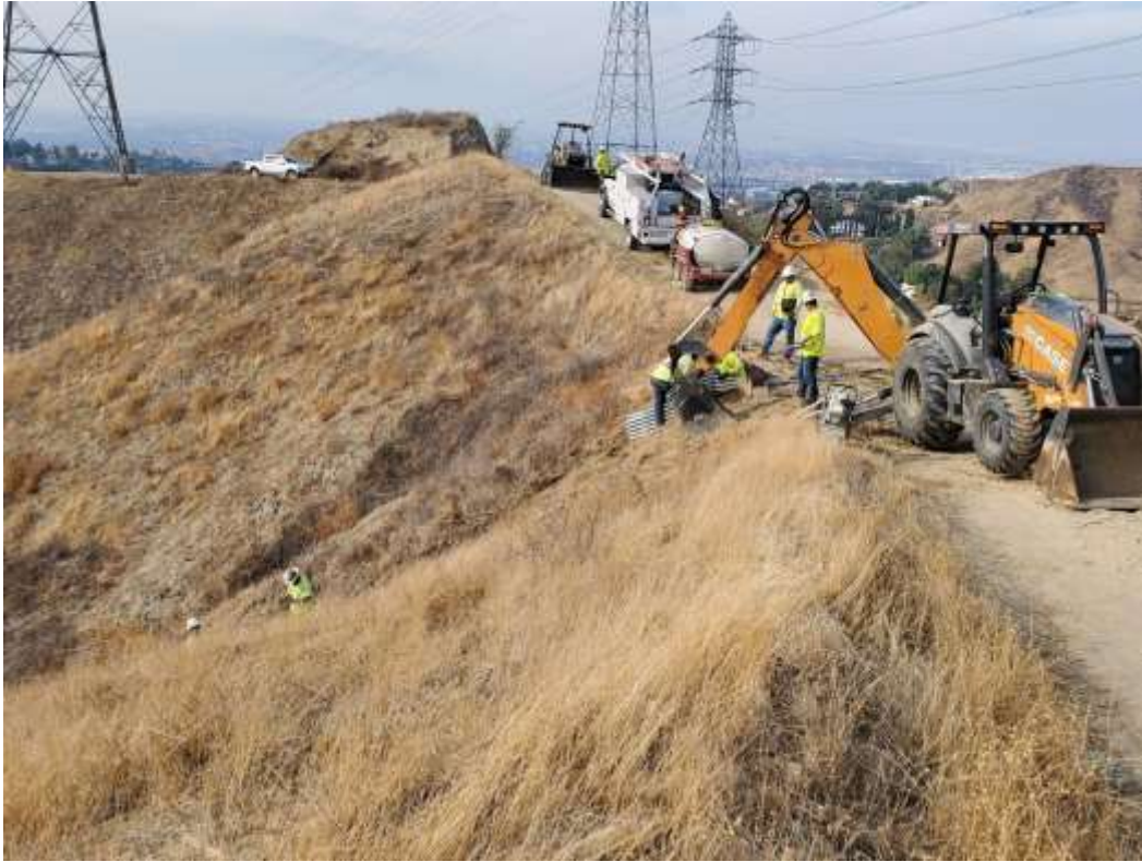
Photo 1 – MAC drain installation near Construction Area 2N18, Segment 2 (November 23, 2020).
