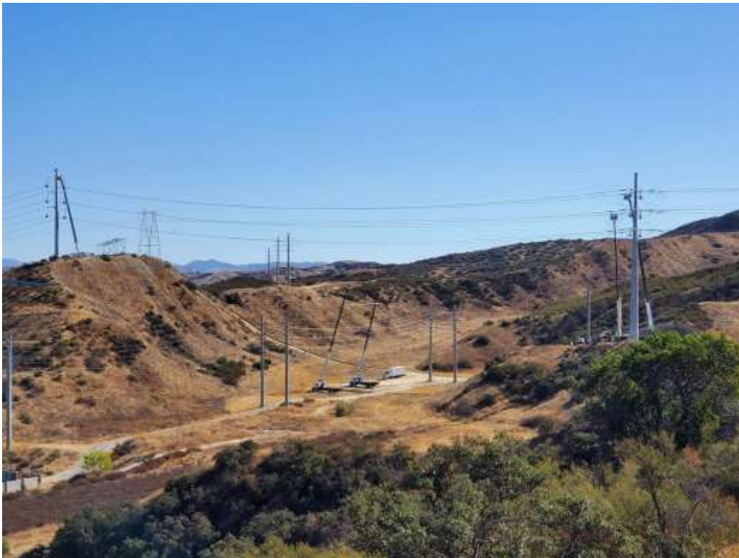
Photo 3 – Wire stringing activities at Construction Areas 3S02 through 3S03, Segment 3 (November 17, 2020).
