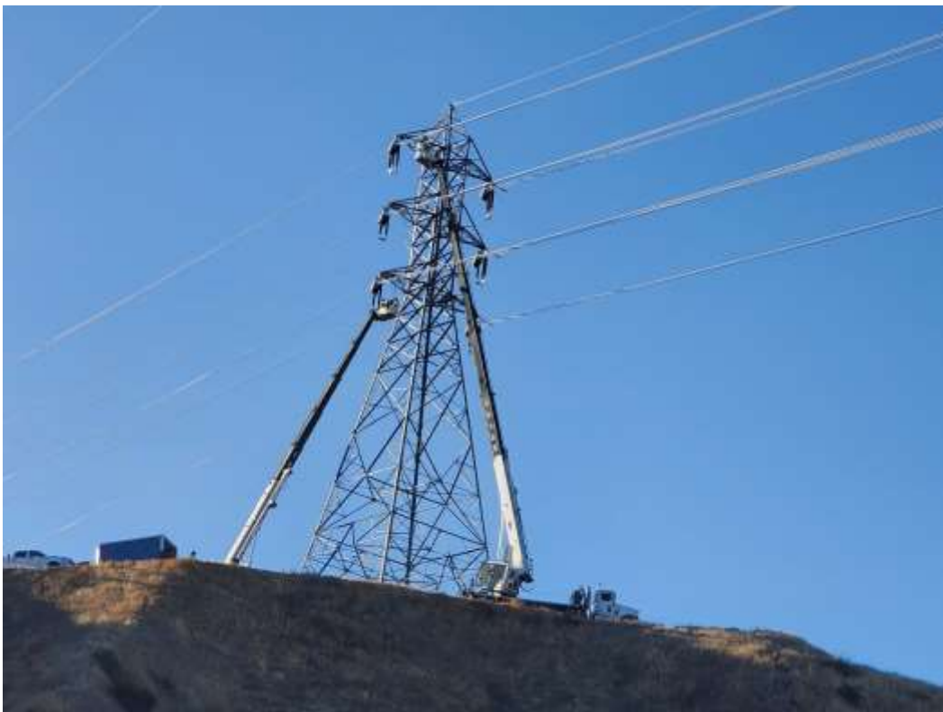
Photo 4 – Wire stringing activities at Construction Area 4X57, Segment 4 (November 19, 2020).
