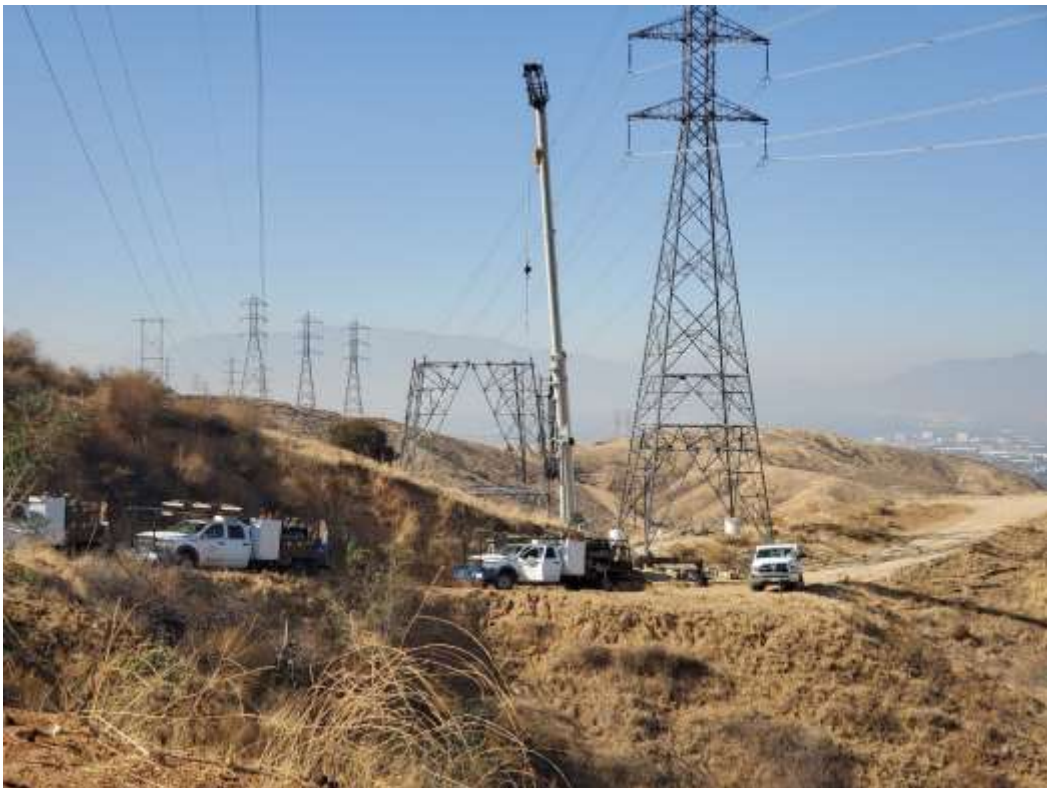
Photo 2 – Tower assembly at Construction Area 3X62, Segment 3 (November 18, 2020).
