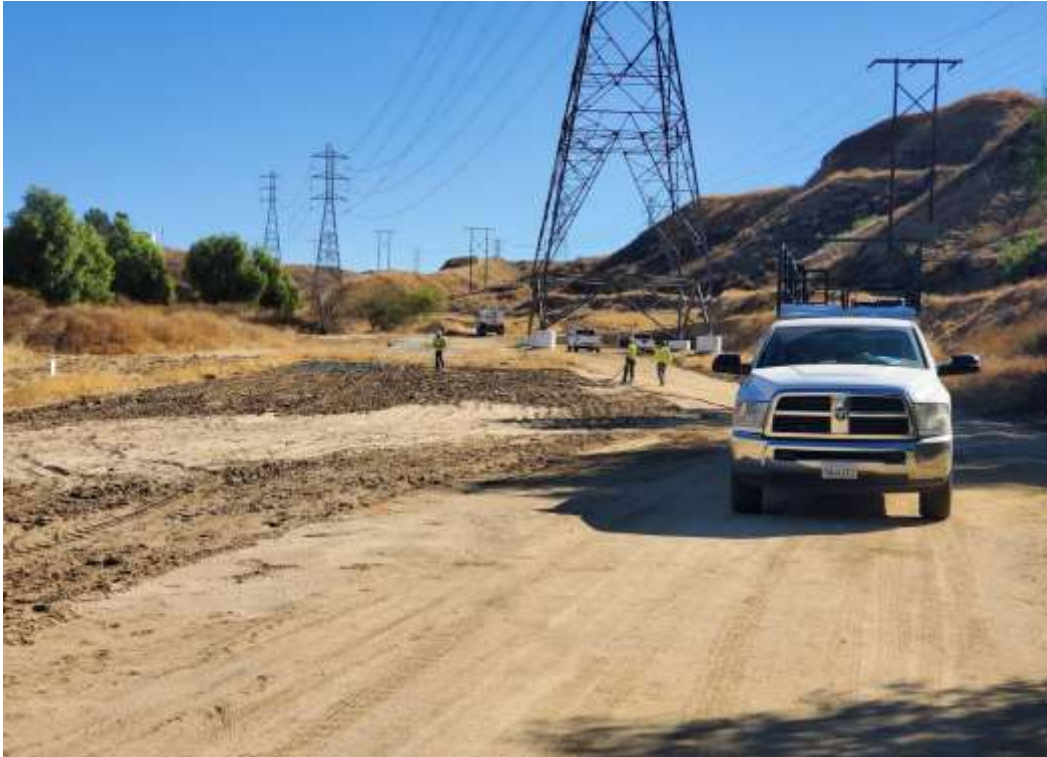
Photo 1 – Hydroseed application at Construction Area WSS-2-2N26-1-MPR-28, Segment 2 (November 30, 2020).
