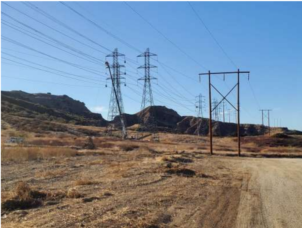
Photo 3 – Wire stringing activities at Construction Areas 3X14 and 3X15, Segment 3 (December 4, 2020).
