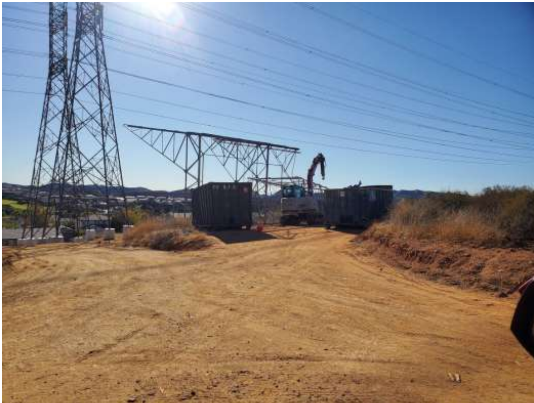
Photo 4 – Tower wreck-out activities at Construction Area 4X52, Segment 4 (December 1, 2020).
