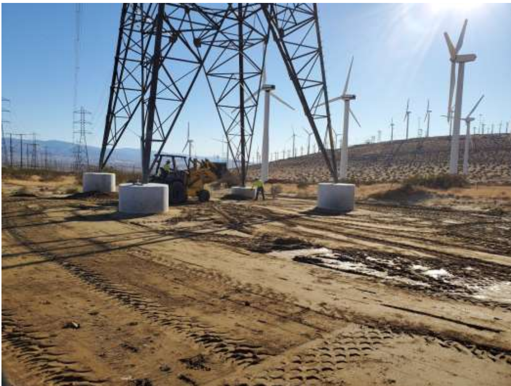
Photo 6 – Site restoration grading at Construction Area 6X24, Segment 6 (December 4, 2020).
