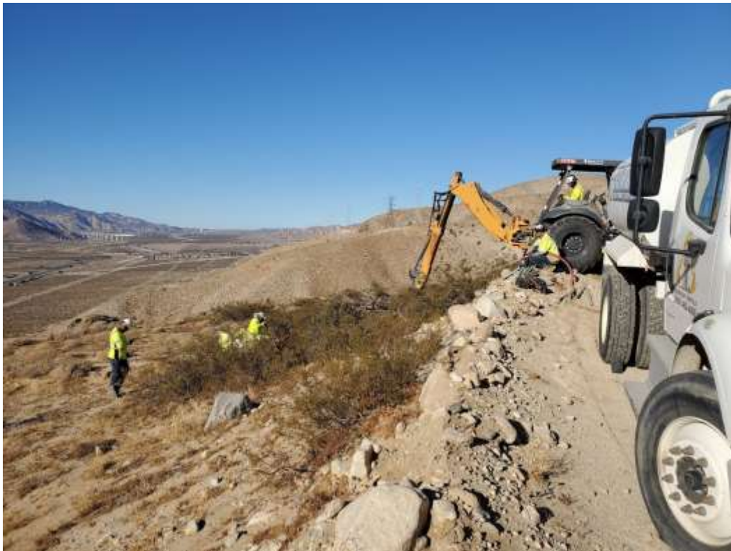
Photo 5 – MAC drain installation near Construction Area 6S28, Segment 6 (December 1, 2020).
