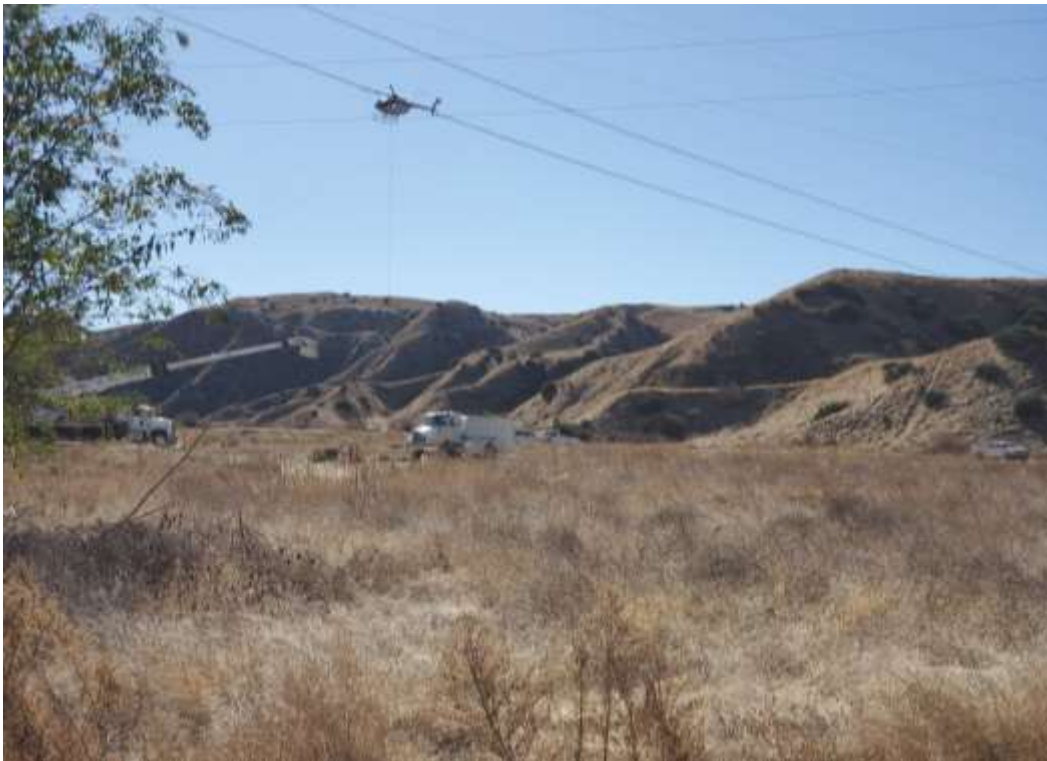
Photo 2 – Helicopter wire wreck-out activities at Construction Area 3X29, Segment 3 (December 1, 2020).
