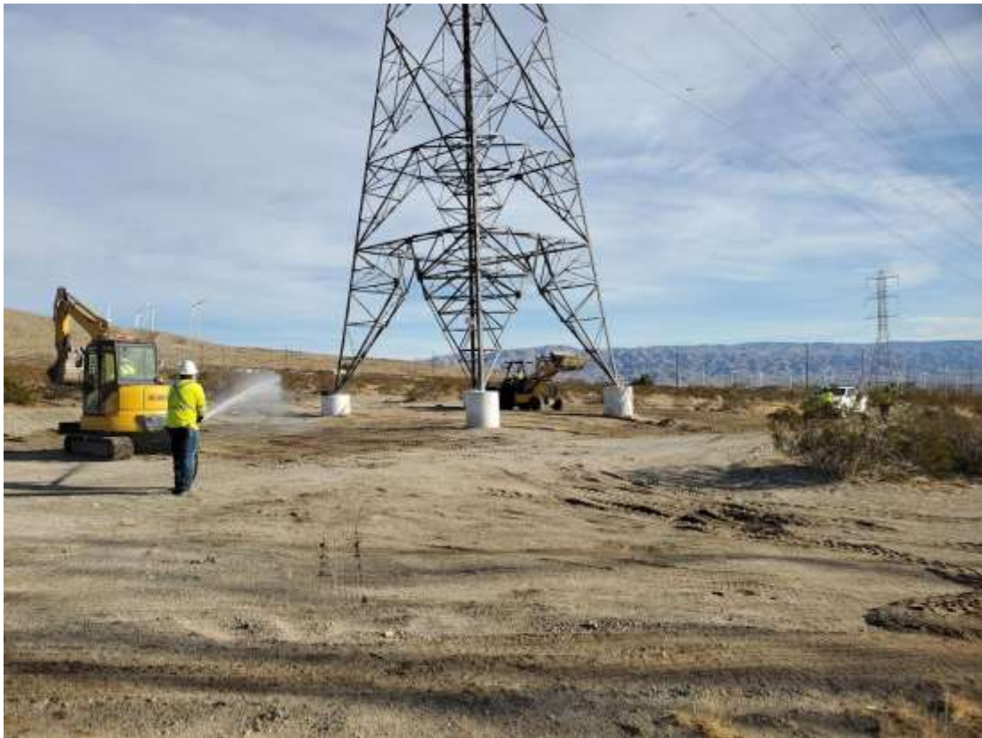
Photo 5 – Site restoration activities at Construction Area 6X22, Segment 6 (January 6, 2021).
