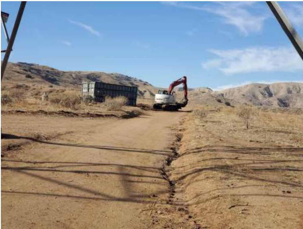
Photo 3 – Tower wreck-out activities at Construction Areas 3X56 (M98-T1), Segment 3 (January 5, 2021).
