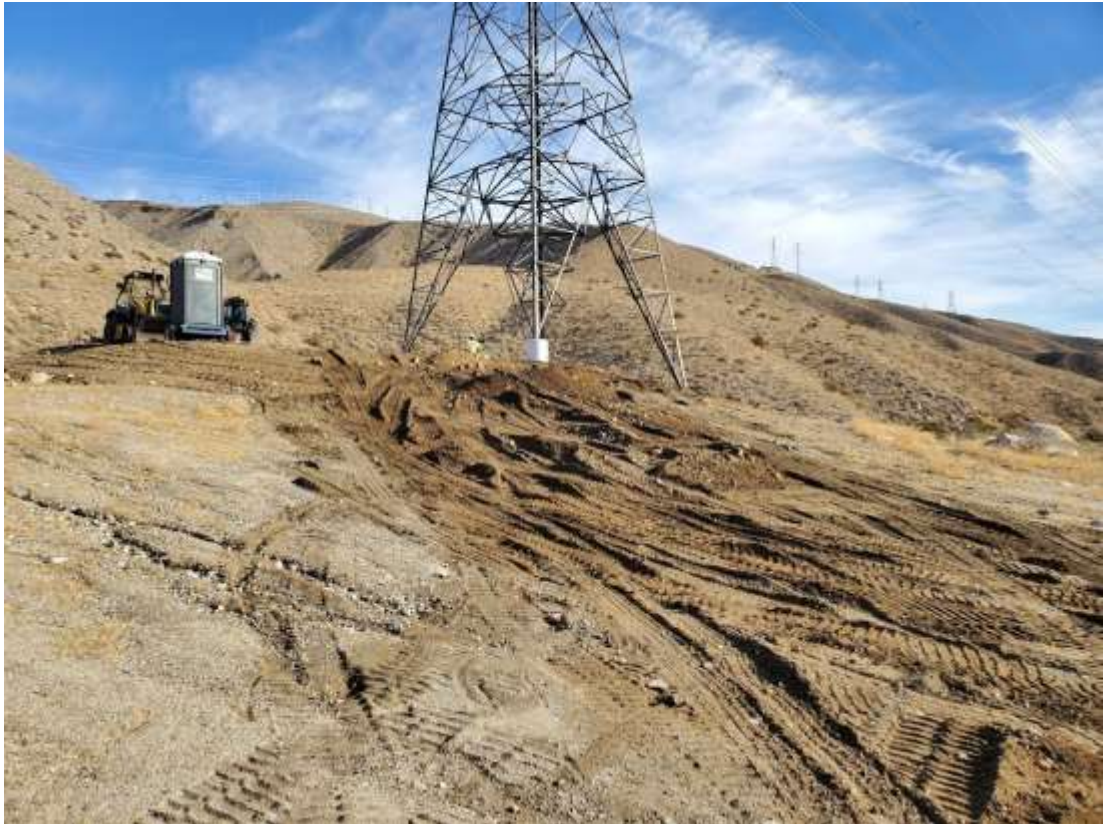
Photo 6 – Site restoration activities at Construction Area 6S32, Segment 6 (January 6, 2021).
