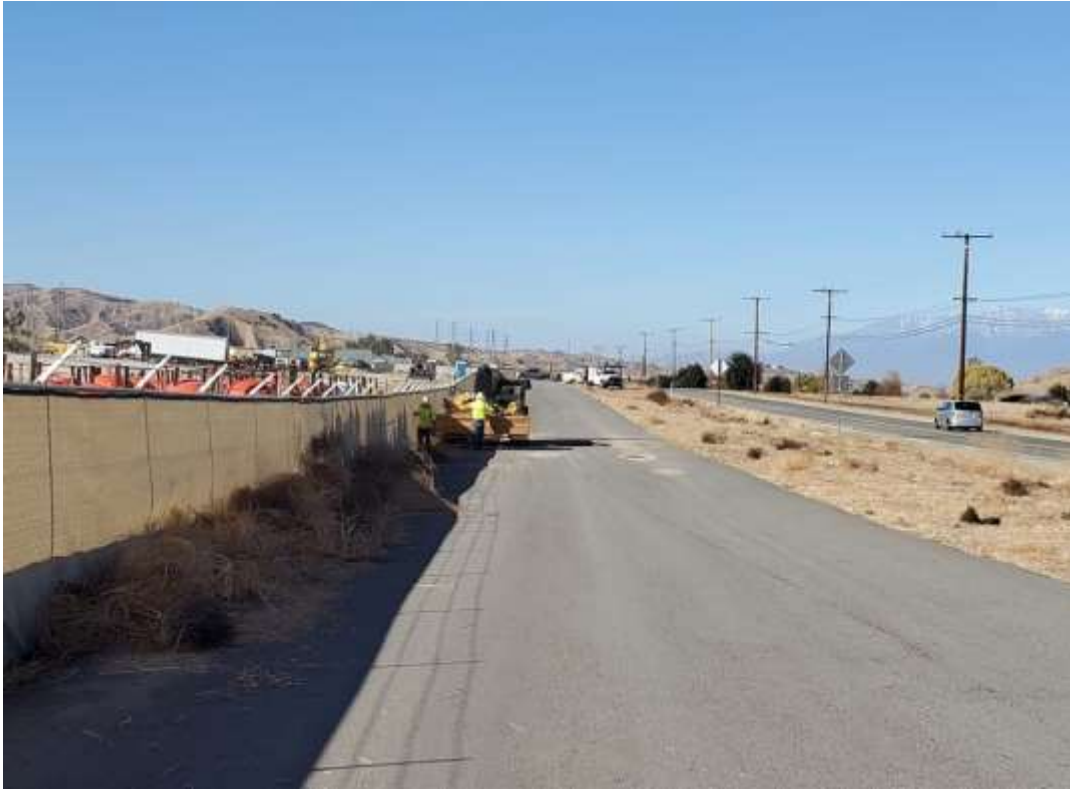
Photo 1 – Maintenance activities at the Poultry MY (January 4, 2021).
