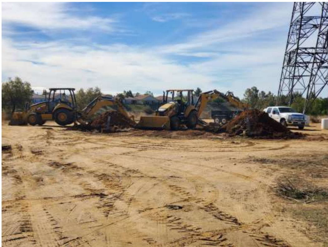
Photo 4 – Foundation wreck-out activities at Construction Area 4X39, Segment 4 (February 2, 2021).
