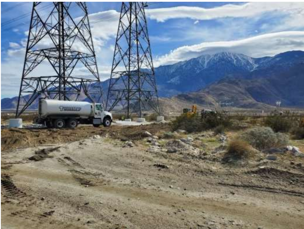
Photo 6 – Site restoration activities at Construction Area 6X44, Segment 6 (February 2, 2021).
