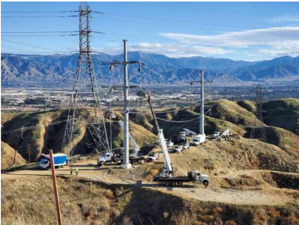
Photo 2 – Wire stringing activities at Construction Areas 1W01 through 1W02, Segment 1 (February 2, 2021).
