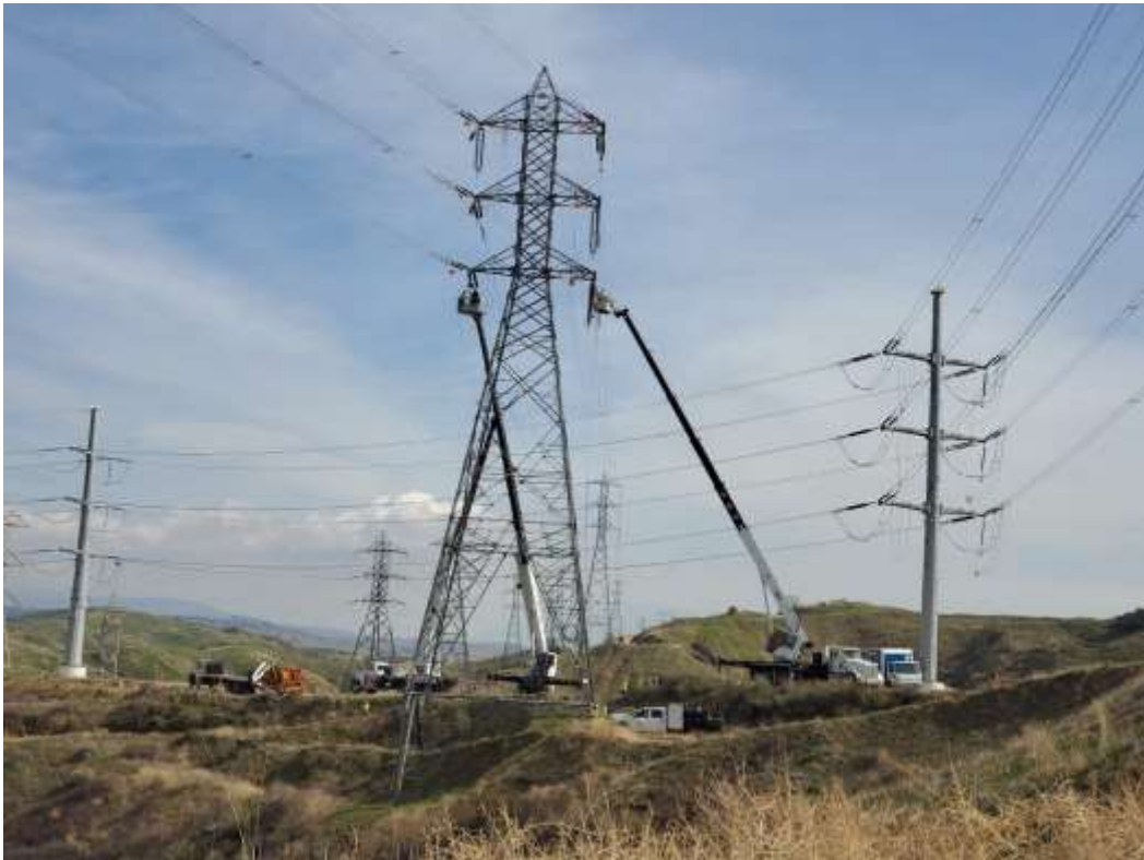
Photo 2 – Wire stringing activities at Construction Area 2N02, Segment 2 (February 16, 2021).
