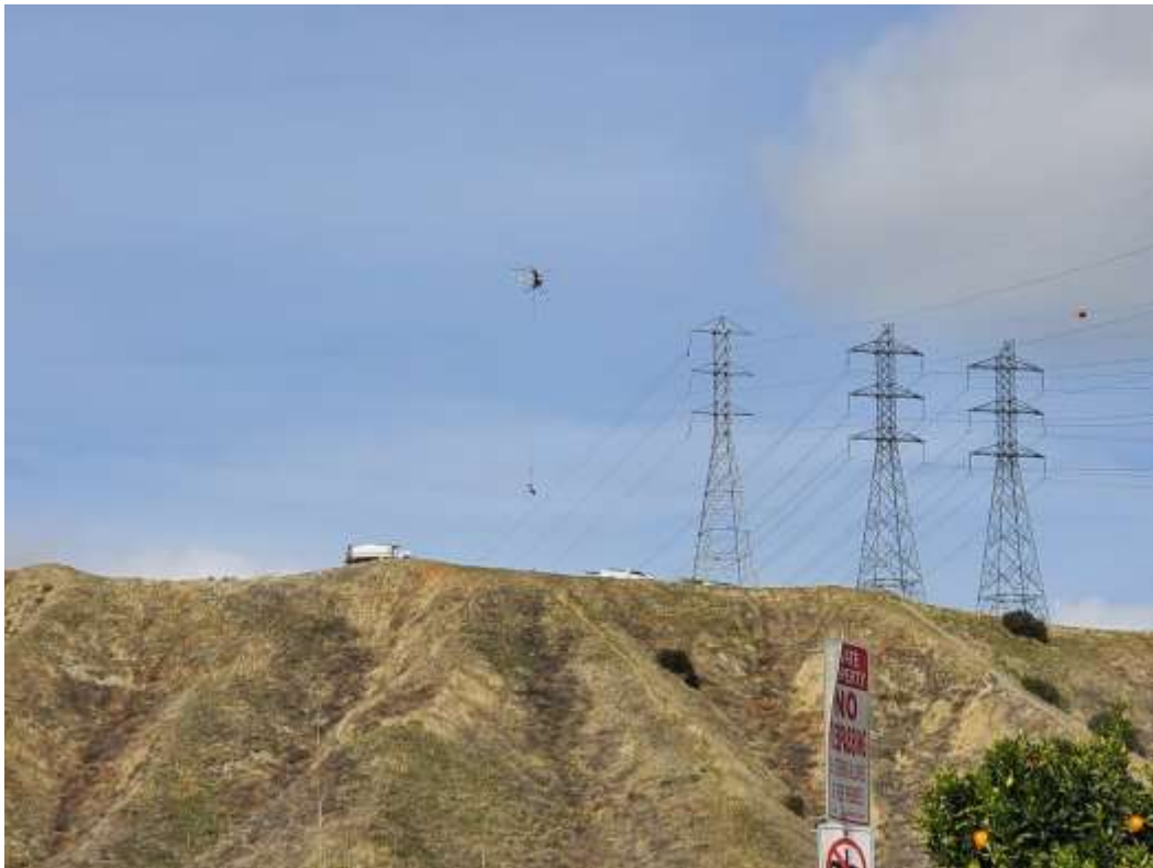
Photo 3 – Helicopter wire wreck-out activities at Construction Area 3X39, Segment 3 (February 16, 2021).
