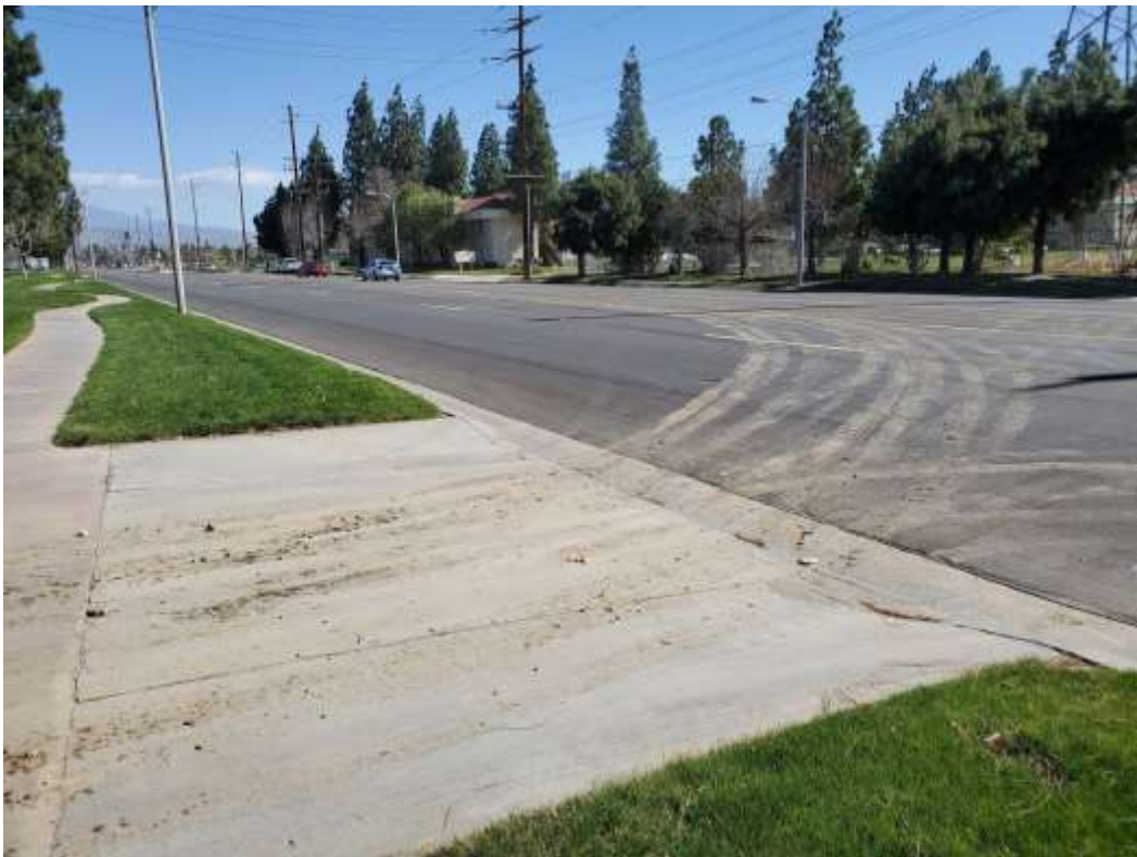
Photo 6 – Track-out observed by CPUC EM at Construction Area 1X19, Segment 1 (February 17, 2021).
