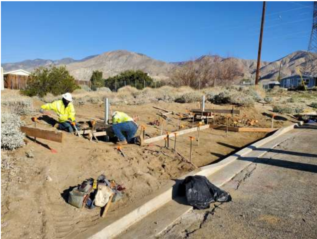
Photo 5 – Gate installation at Construction Area 6S39, Segment 6 (February 17, 2021).
