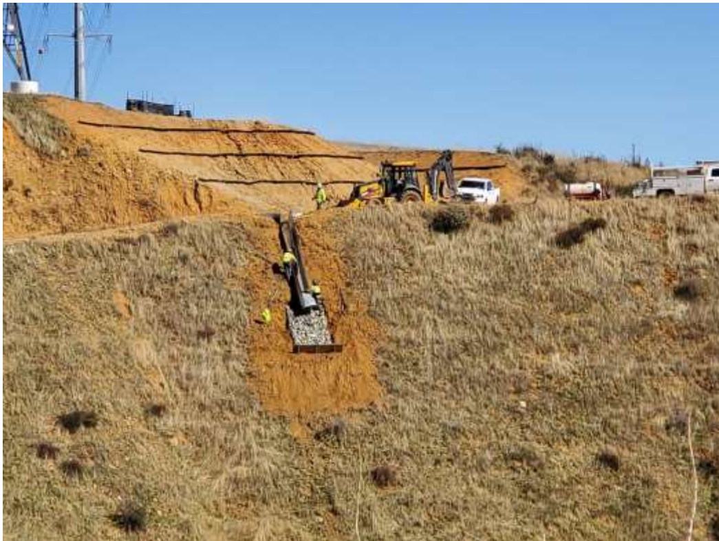
Photo 4 – MAC drain installation at Construction Area 4X06, Segment 4 (February 18, 2021).
