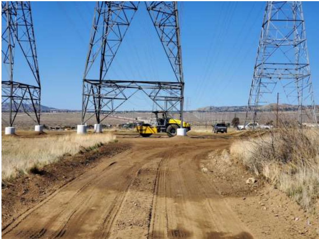
Photo 4 – Site restoration activities at Construction Area 5X24, Segment 5 (March 2, 2021).
