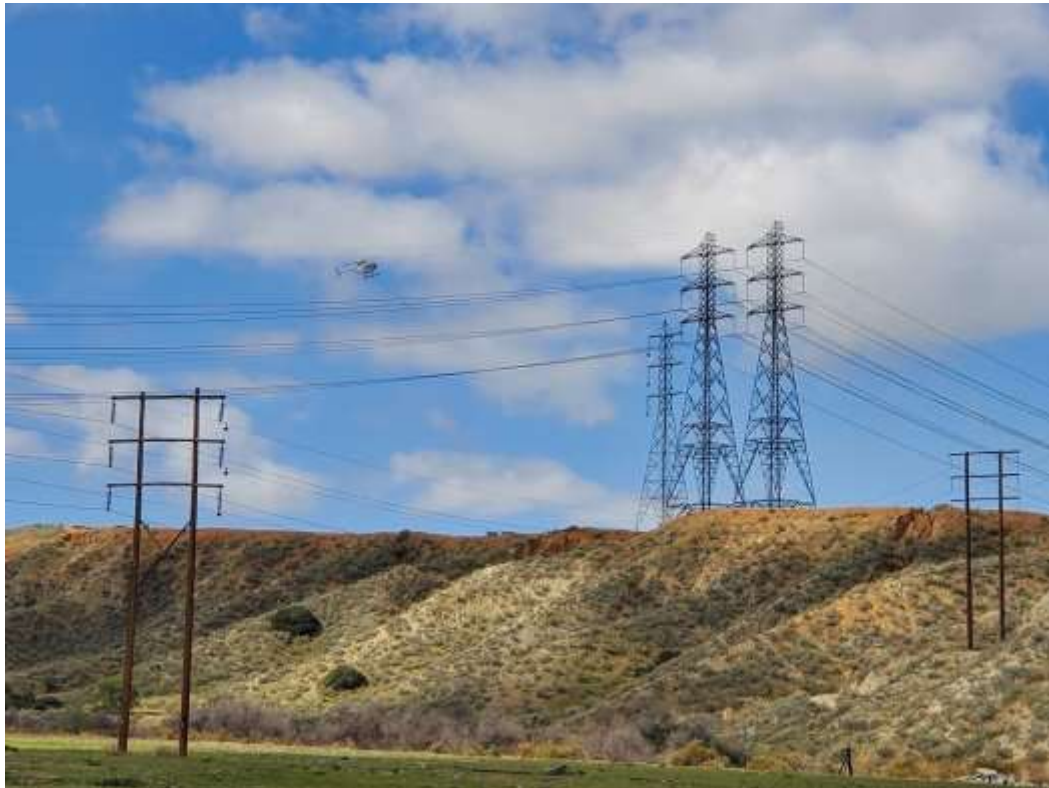
Photo 2 – Helicopter wire wreck-out activities at Construction Area 3X50, Segment 3 (March 4, 2021).
