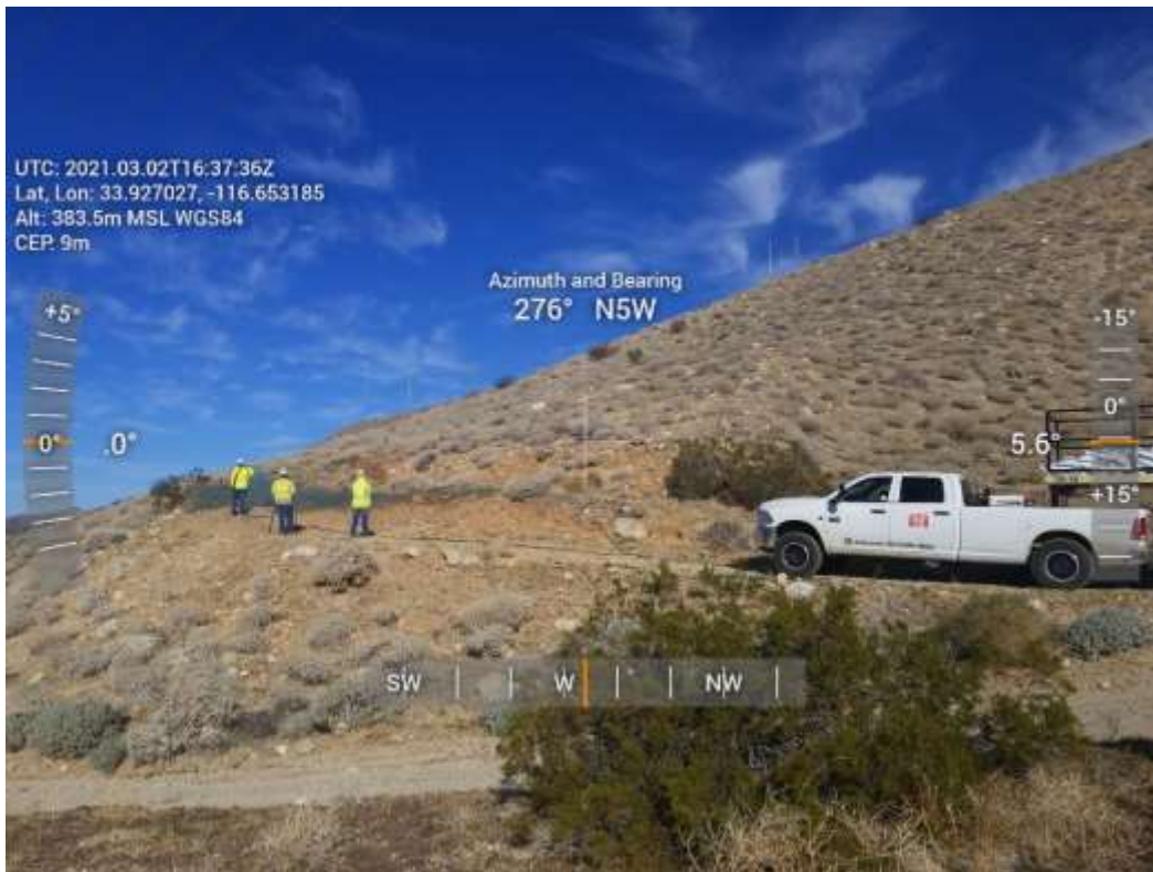
Photo 7 – Hydroseed application at Construction Area 6S39, Segment 6 (Photo courtesy of SCE) (March 2, 2021).
