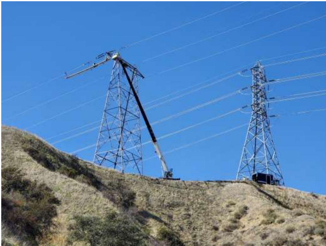
Photo 3 – Wire wreck-out activities at Construction Area 4S58 (M88-T2), Segment 4 (March 4, 2021).
