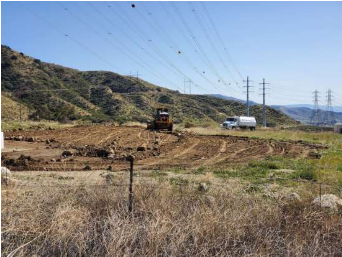
Photo 3 – Site restoration grading at Construction Area 4X01, Segment 4 (March 22, 2021).
