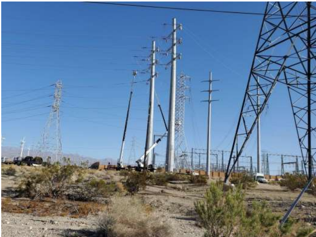
Photo 6 – Wire stringing activities at Construction Areas 6X07 and 6X08, Segment 6 (March 24, 2021).
