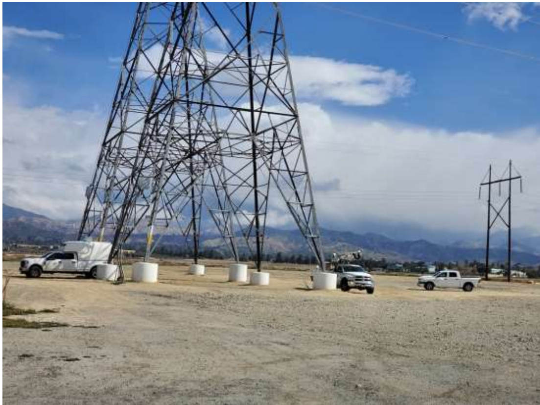
Photo 4 – Telecom testing and splicing at Construction Area 4X35, Segment 4 (March 23, 2021).
