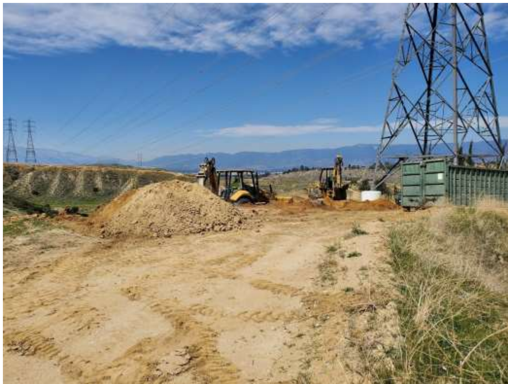
Photo 2 – Foundation wreck-out activities at Construction Area 3X48, Segment 3 (March 22, 2021).
