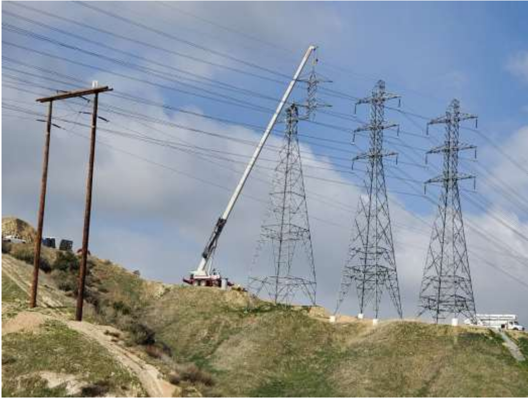
Photo 1 – Tower wreck-out at Construction Area 3X08, Segment 3 (March 23, 2021).
