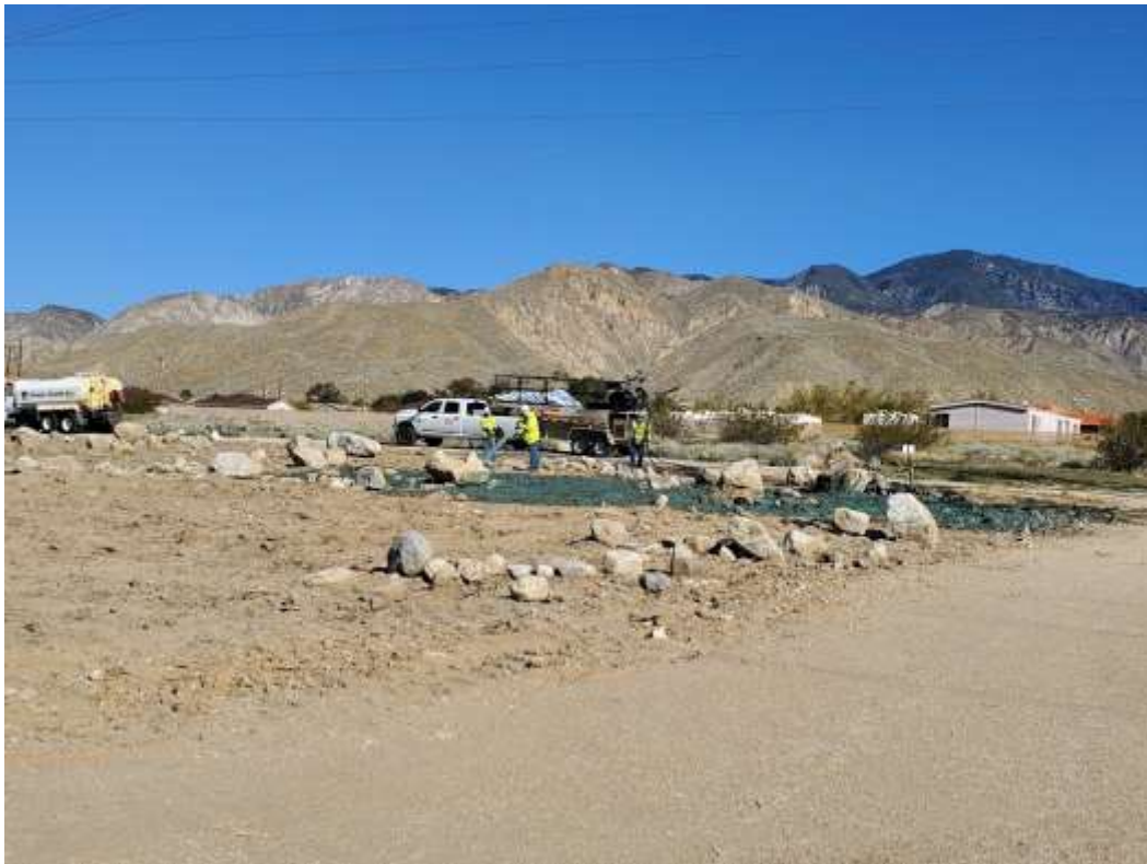
Photo 5 – Hydroseed application at Construction Area 5X01, Segment 5 (March 22, 2021).
