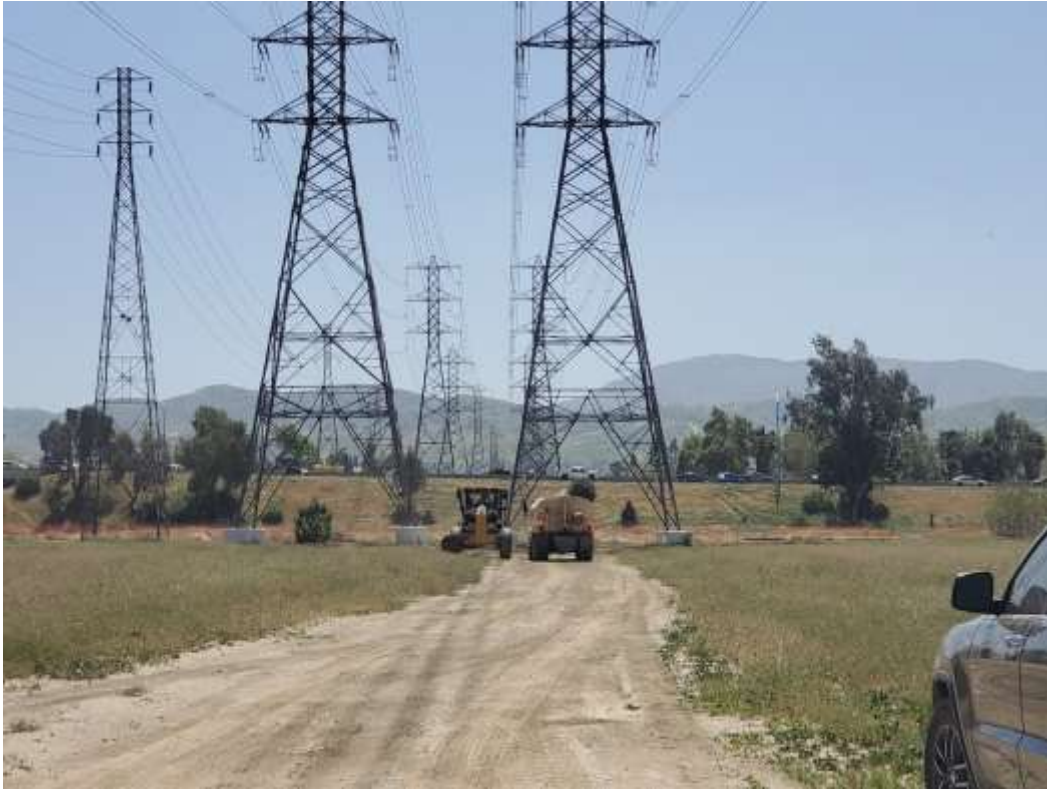
Photo 1 – Site restoration activities at Construction Area 1X21, Segment 1 (April 8, 2021).
