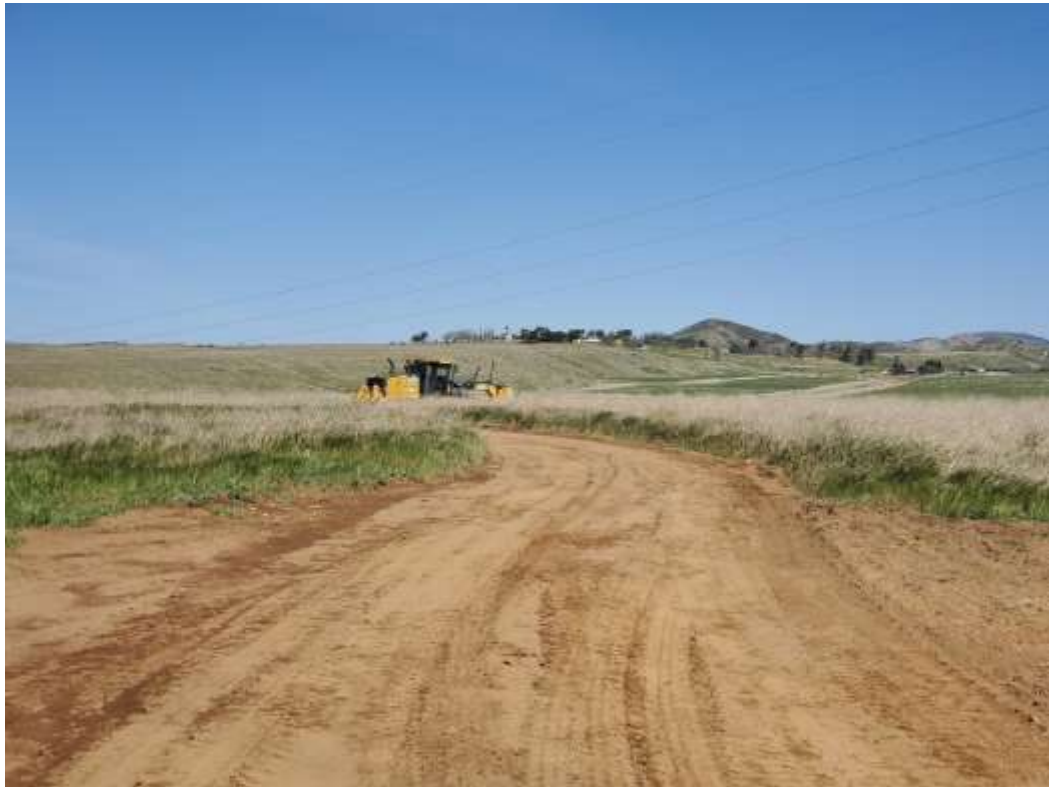
Photo 4 – Access road maintenance at Construction Area 4X06, Segment 4 (April 5, 2021).
