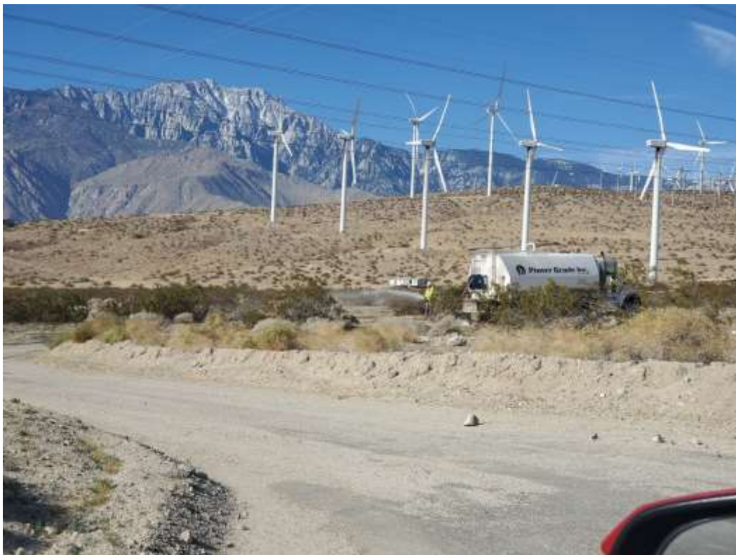
Photo 6 – Hydroseed watering at Construction Area 6S18, Segment 6 (April 8, 2021).
