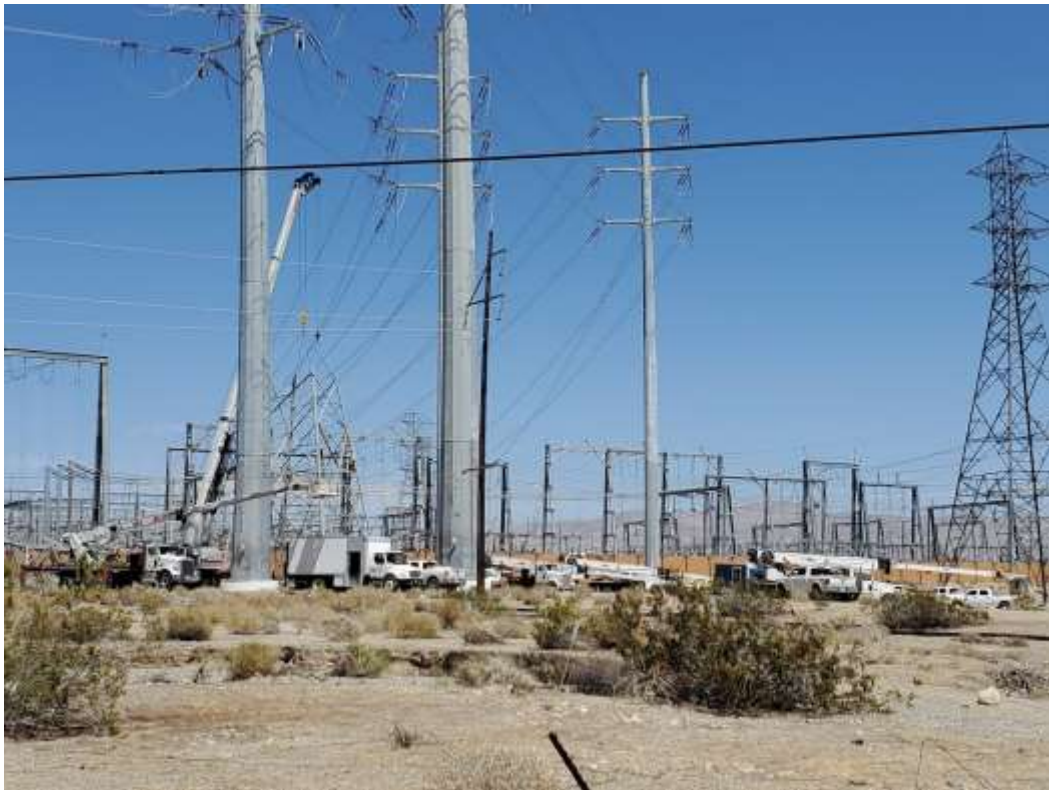
Photo 5 – Tower wreck-out activities at Construction Area 6X08, Segment 6 (April 7, 2021).
