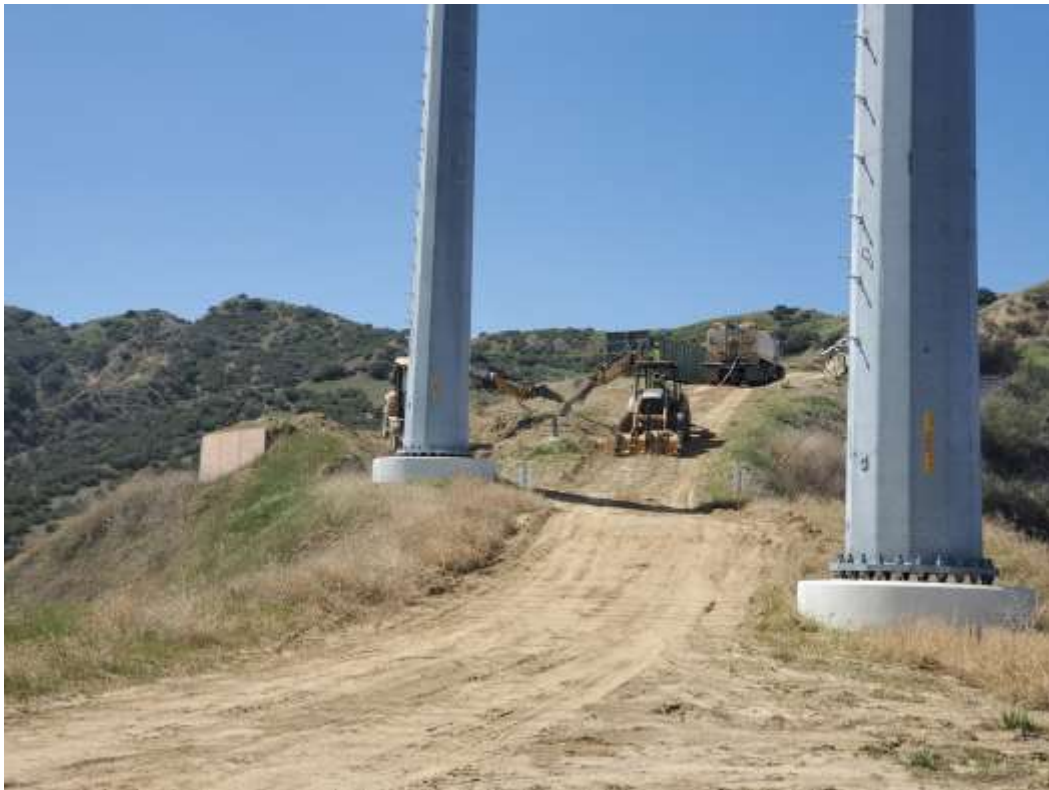
Photo 3 – Foundation wreck-out at Construction Area 3X16, Segment 3 (April 8, 2021).
