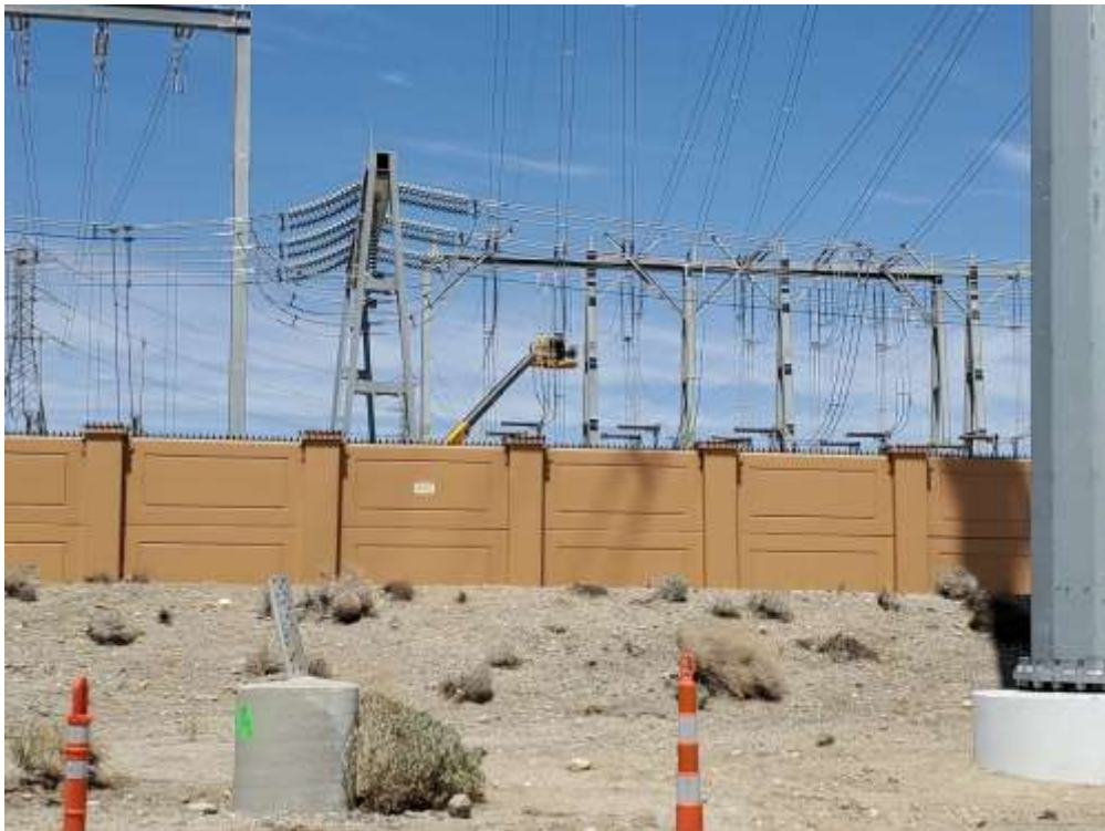
Photo 2 – Wire stringing activities at the Devers Substation (April 15, 2021).
