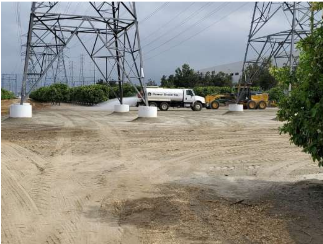
Photo 3 – Site restoration activities at Construction Area 1X24, Segment 1 (April 14, 2021).
