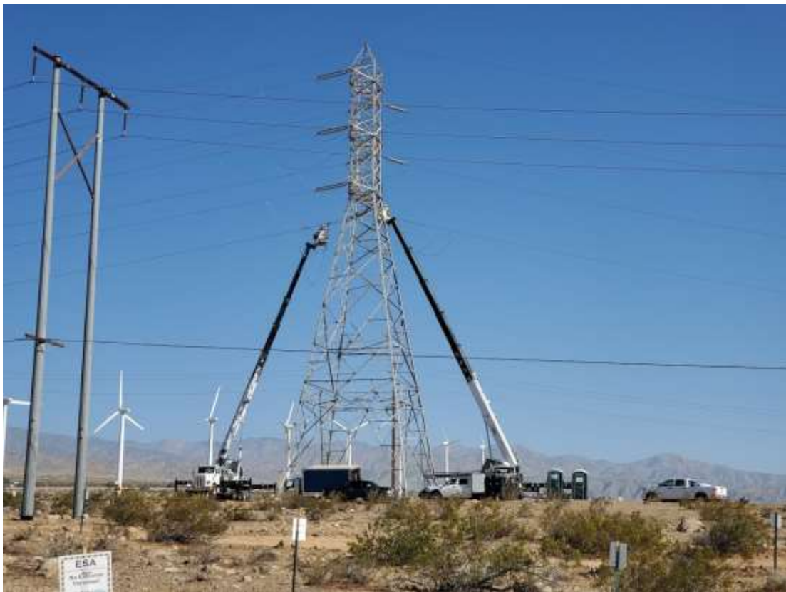
Photo 6 – Wire wreck-out activities at Construction Area M0-T4, Segment 6 (April 12, 2021).
