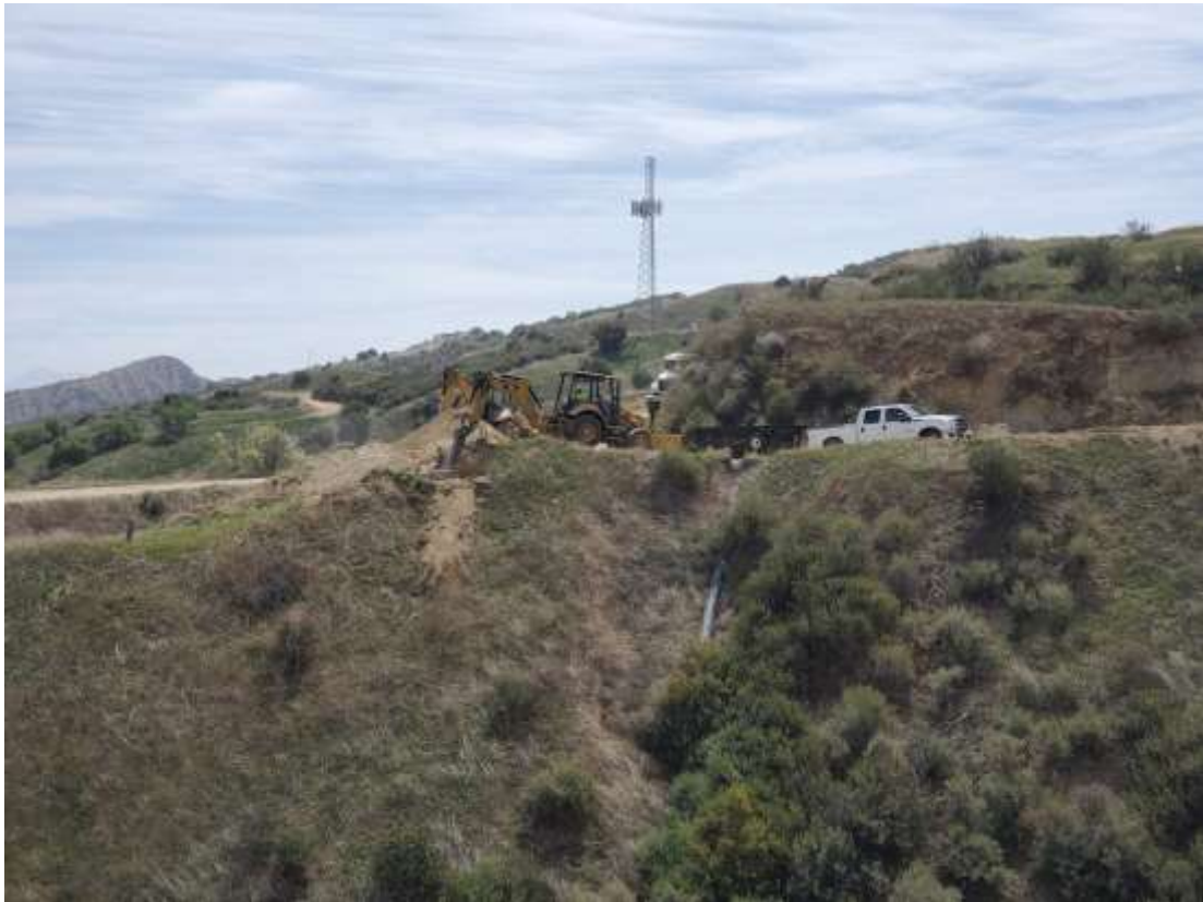
Photo 5 – Foundation wreck-out activities at Construction Area 3X28, Segment 3 (April 15, 2021).
