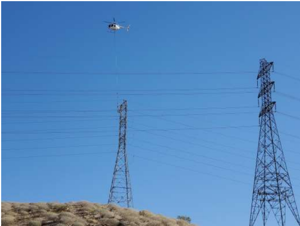
Photo 5 – Wire wreck-out activities at Construction Area 6X35, Segment 6 (April 20, 2021).
