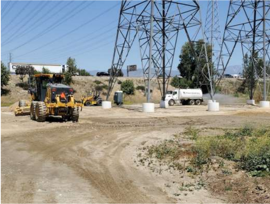
Photo 1 – Site restoration and grading at Construction Area 1X21, Segment 1 (April 20, 2021).
