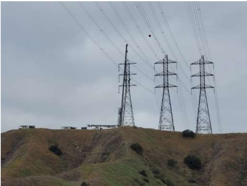
Photo 2 – Tower wreck-out at Construction Area 3X40, Segment 3 (April 21, 2021).
