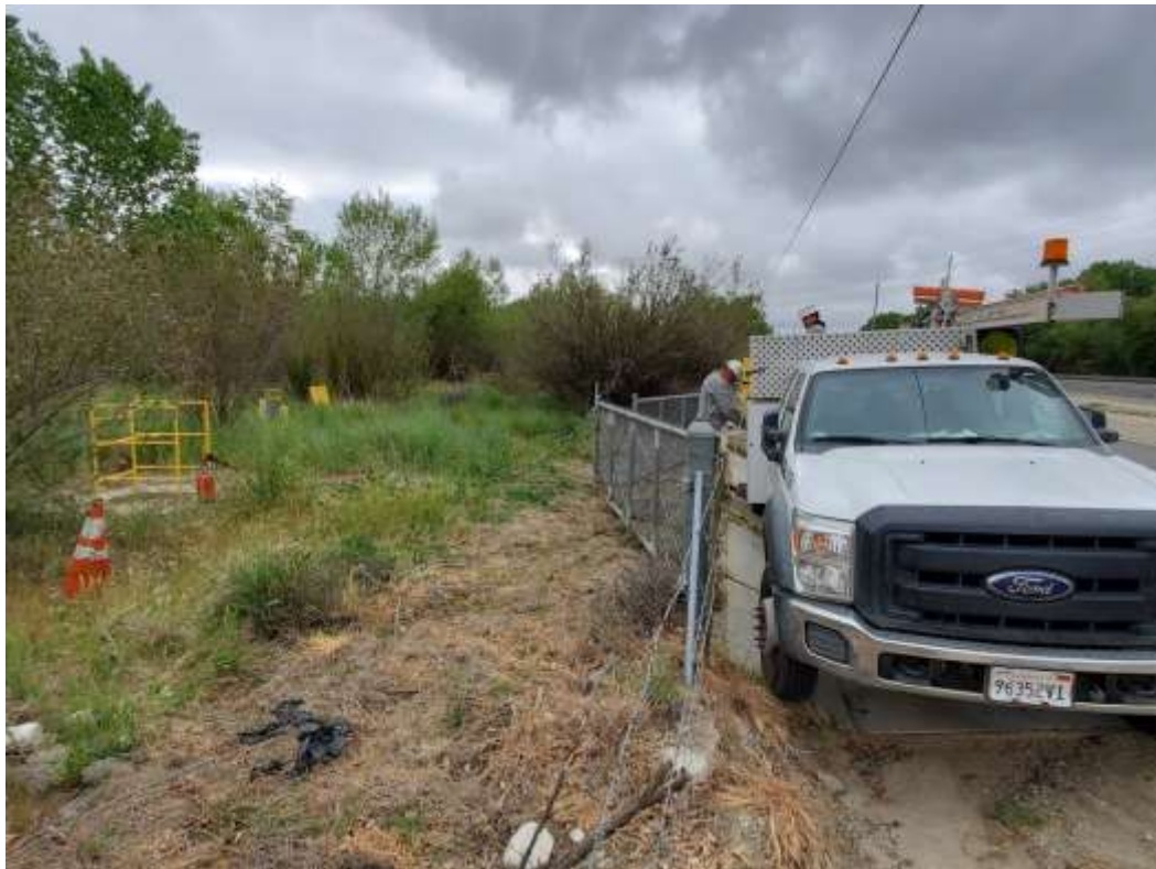
Photo 4 – Telecom vault de-watering at Construction Area TEWS-31, Segment 3 (April 21, 2021).
