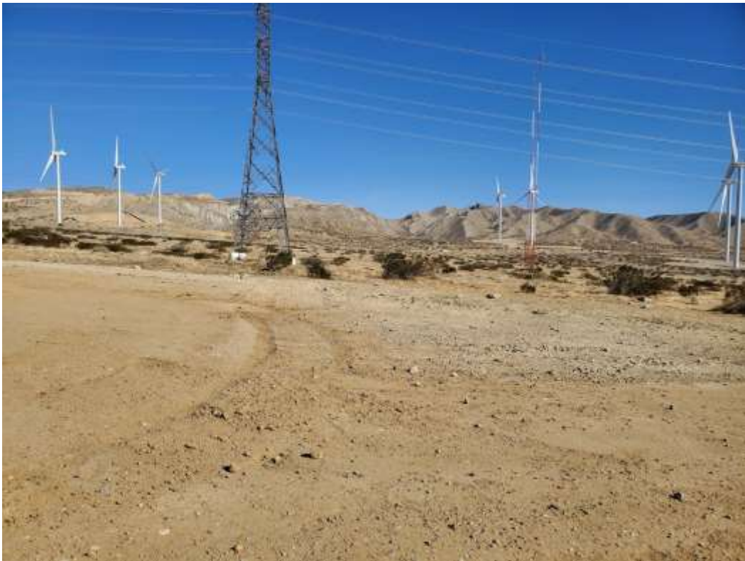
Photo 7 – Hydroseeded area at Construction Area 6S25, Segment 6 (March 8, 2021).
