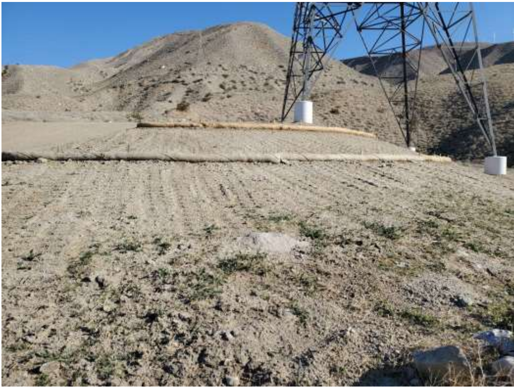
Photo 9 – Hydroseeded area at Construction Area 6S32, Segment 6 (March 16, 2021).
