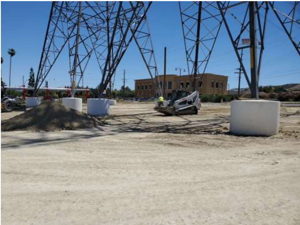
Photo 3 – Site restoration and foundation compaction at Construction Area 1X10, Segment 1 (April 29, 2021).
