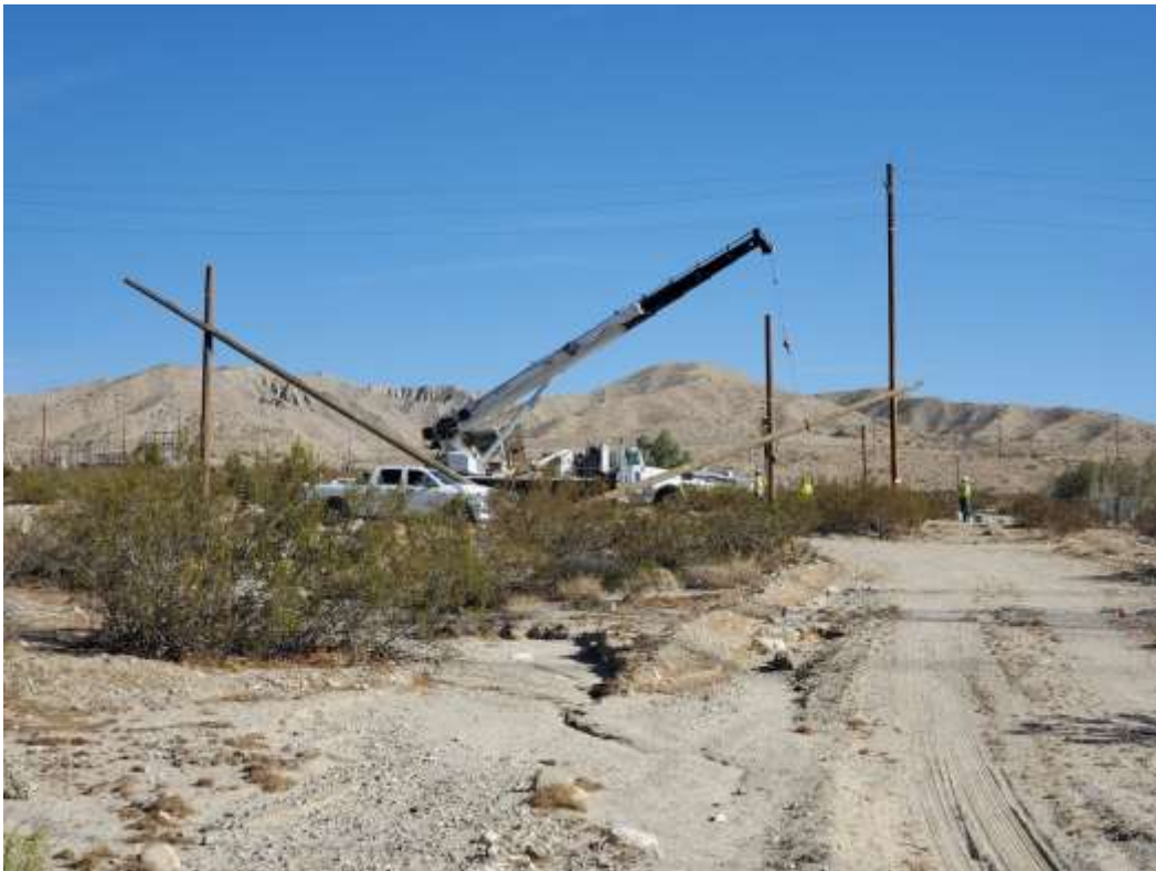
Photo 8 – Guard pole removal at Construction Area GS-6N20-6N21-1, Segment 6 (April 30, 2021).
