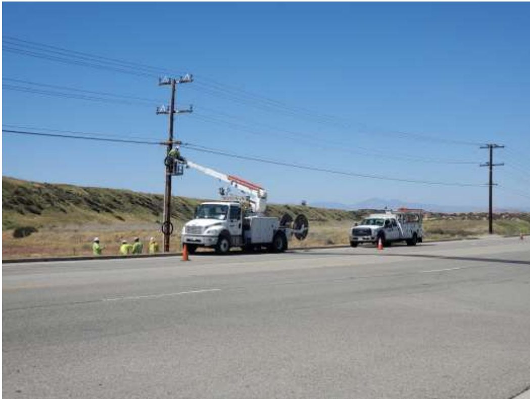
Photo 6 – Fiber optic installation at Construction Area SWA-OakValleyParkwayTelecom-MPR-46, Segment 4 (April 30, 2021).
