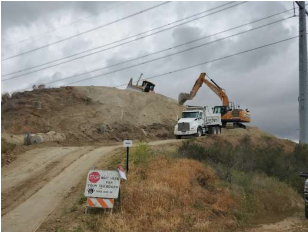
Photo 5 – Tower pad recontouring at Construction Area 3S02, Segment 3 (April 26, 2021).
