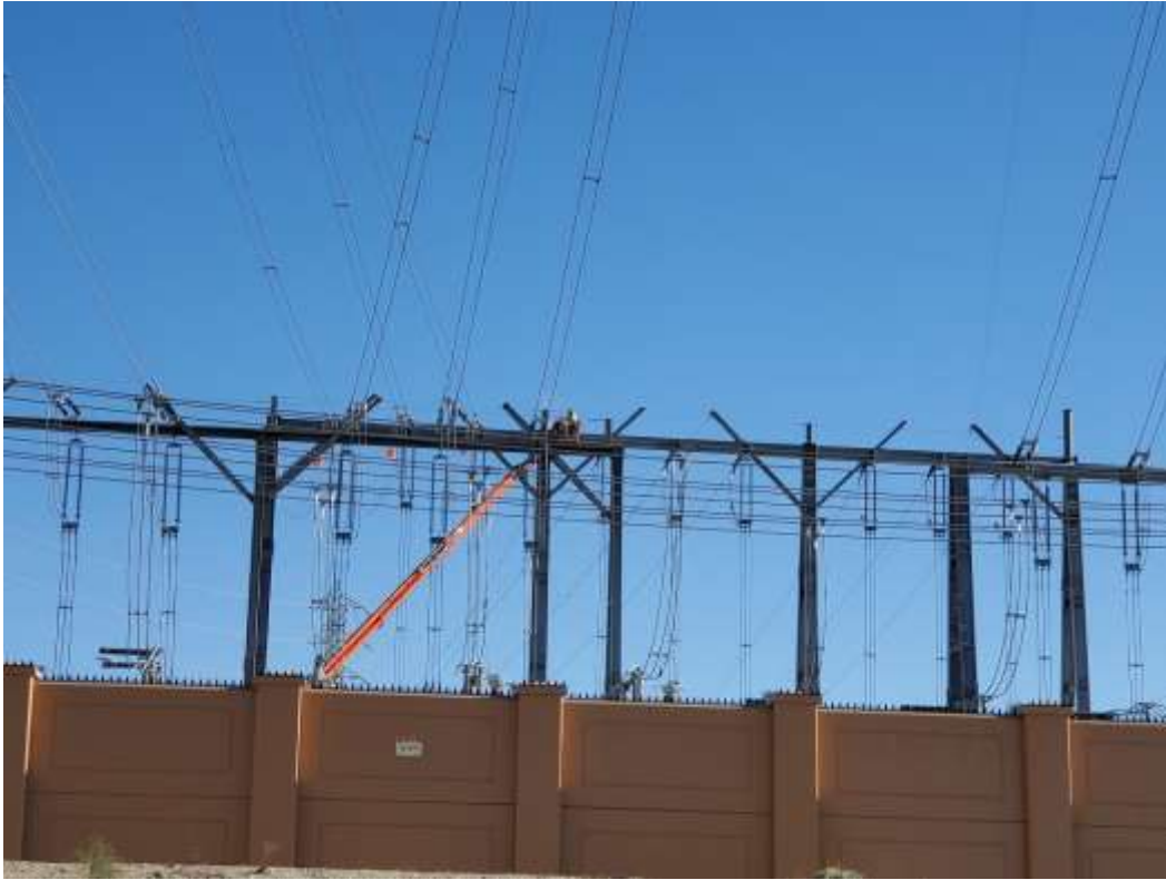
Photo 1 – Support welding at the Devers Substation (April 30, 2021).
