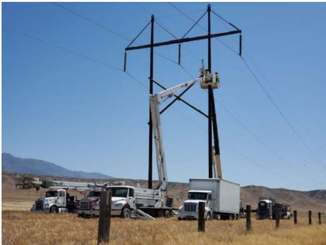
Photo 4 – Wire wreck-out activities at Construction Area 4X21, Segment 4 (May 12, 2021).
