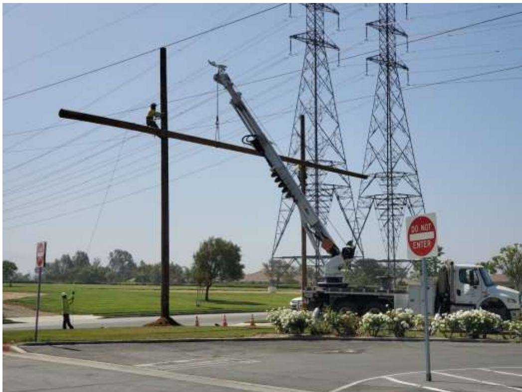
Photo 5 – Guard pole installation at Construction Area GS-4-W-4X38-1-MPR-32, Segment 4 (May 14, 2021).
