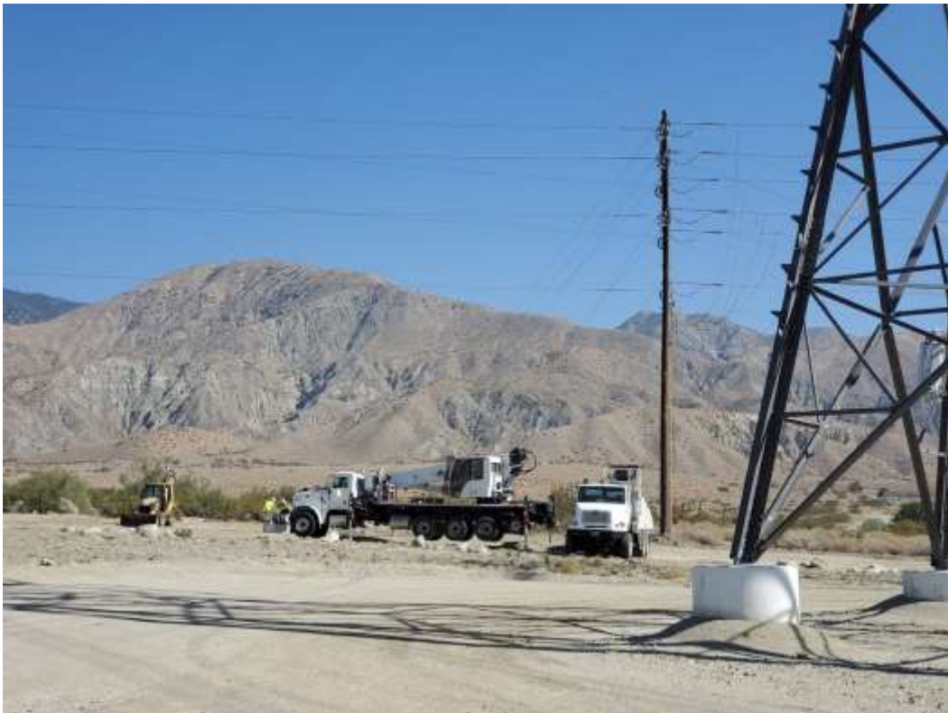
Photo 7 – Wire wreck-out activities at Construction Area 6X42, Segment 6 (May 11, 2021).
