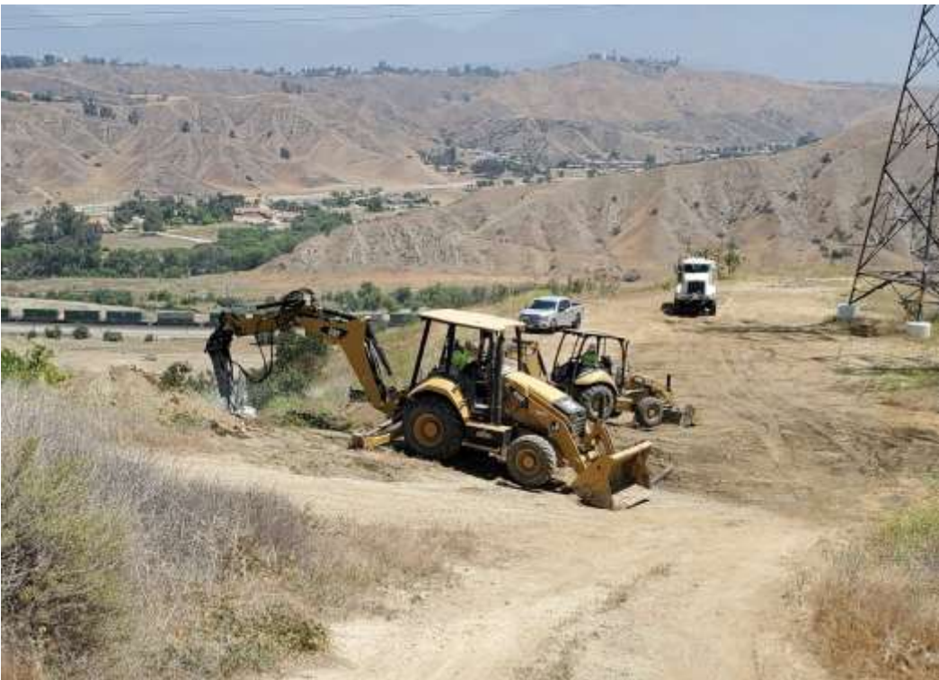
Photo 2 – Foundation wreck-out activities at Construction Area 3X38, Segment 3 (May 12, 2021).
