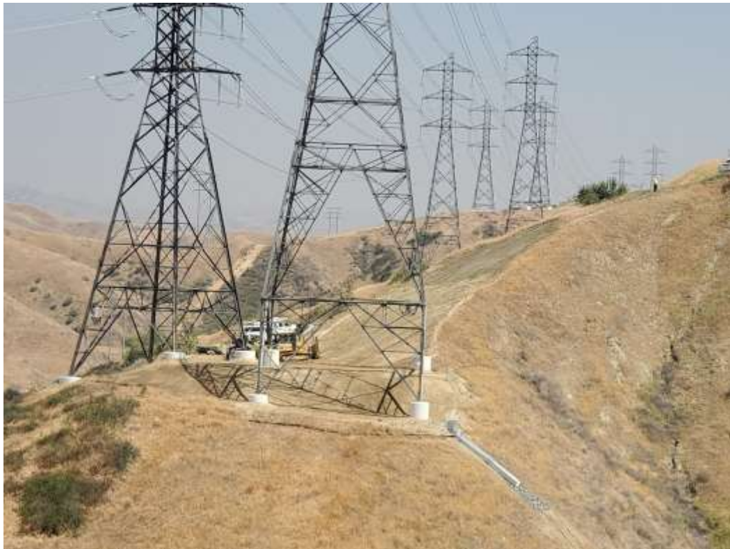
Photo 3 – Site restoration activities at Construction Area 3X65, Segment 3 (May 11, 2021).
