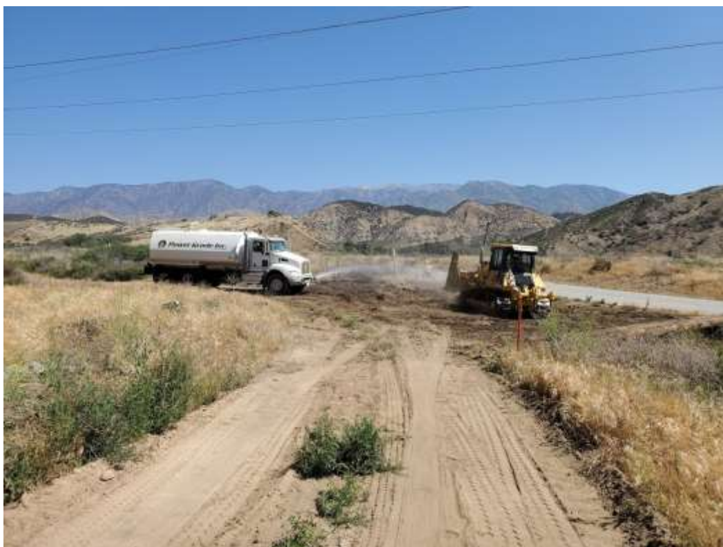
Photo 6 –Vegetation clearing and grading activities at Construction Area SWA-4-PP123353-4-MPR-46, Segment 4 (May 12, 2021).
