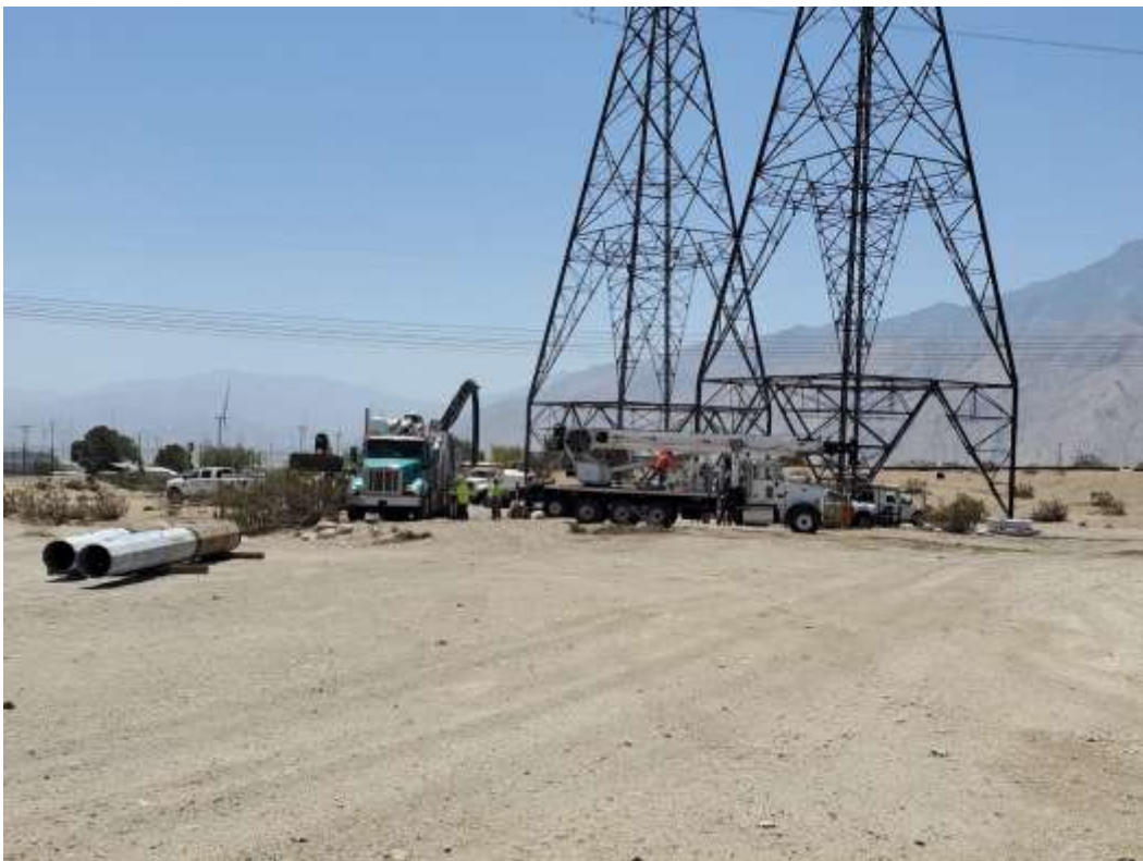
Photo 8 – Shoofly tower base removal at Construction Area 6X09-6X10, Segment 6 (May 14, 2021).
