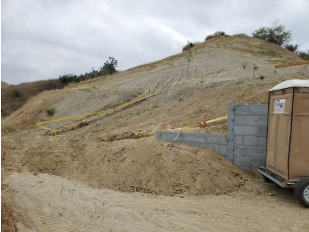
Photo 1 – V-ditch excavation at Construction Area 3X36, Segment 3 (May 17, 2021).
