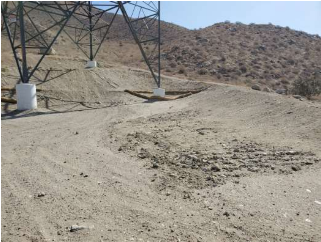
Photo 9 – Hydroseeded area at Construction Area 6S31, Segment 6 (May 21, 2021).
