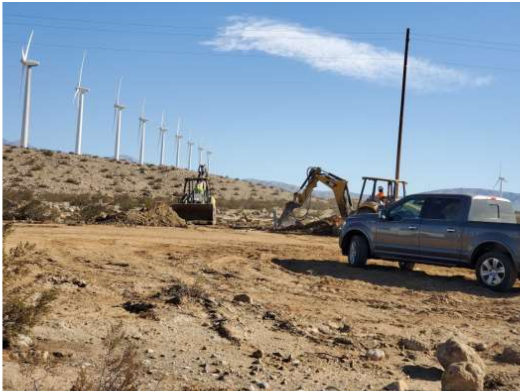
Photo 5 – Foundation wreck-out at Construction Area M0-T5(1), Segment 6 (May 20, 2021).
