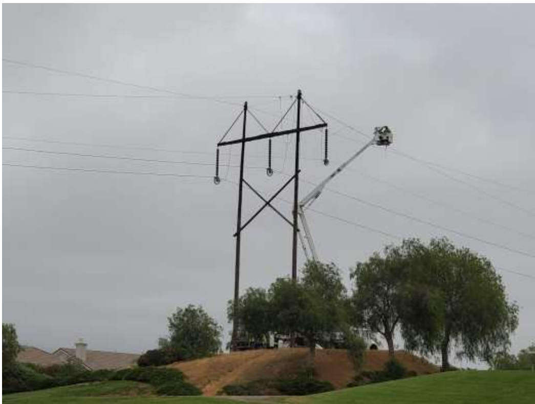
Photo 2 – Wire wreck-out activities at Construction Area PP#123307, Segment 4 (May 20, 2021).
