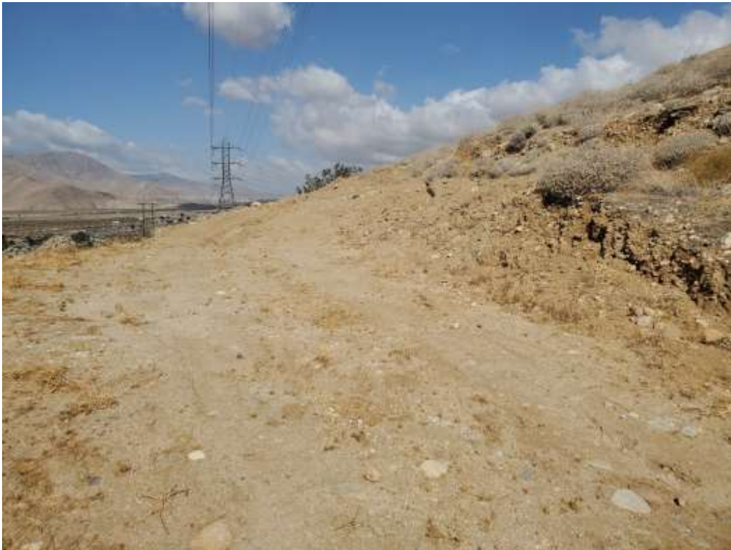
Photo 8 – Hydroseeded area at Construction Area T247, Segment 6 (May 21, 2021).
