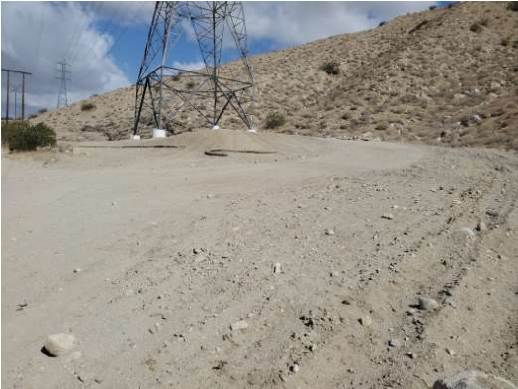
Photo 10 – Hydroseeded area at Construction Area 6S31A, Segment 6 (May 21, 2021).
