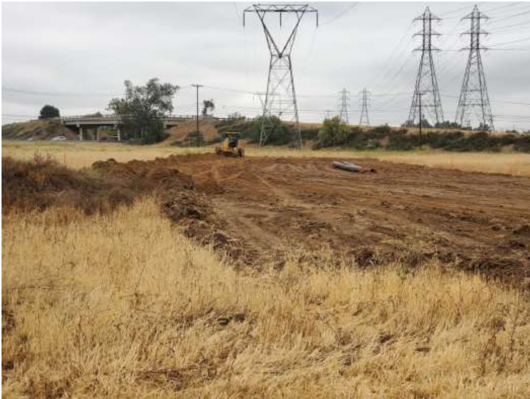
Photo 4 – Vegetation clearing and grading at Construction Area WSS-4X45-4X46, Segment 4 (May 17, 2021).
