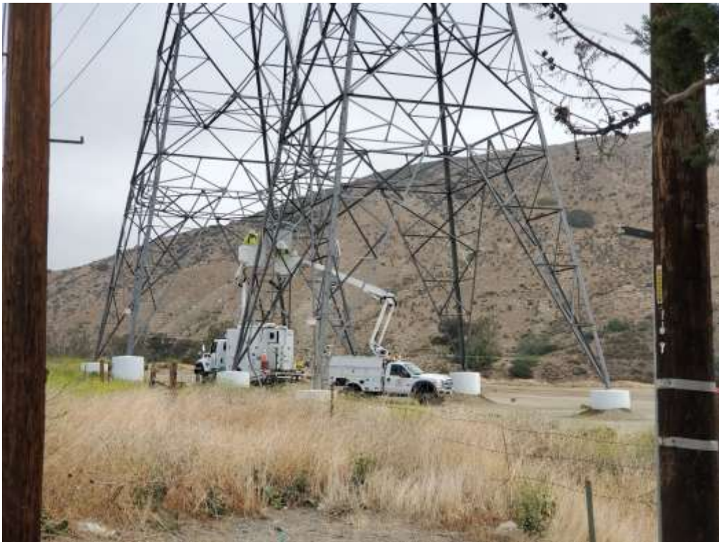
Photo 3 – Fiber splicing activities at Construction Area 4X01, Segment 4 (May 20, 2021).
