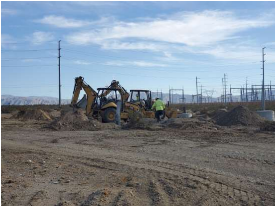
Photo 5 – Foundation wreck-out at Construction Area M0-T2(1), Segment 6 (May 25, 2021).
