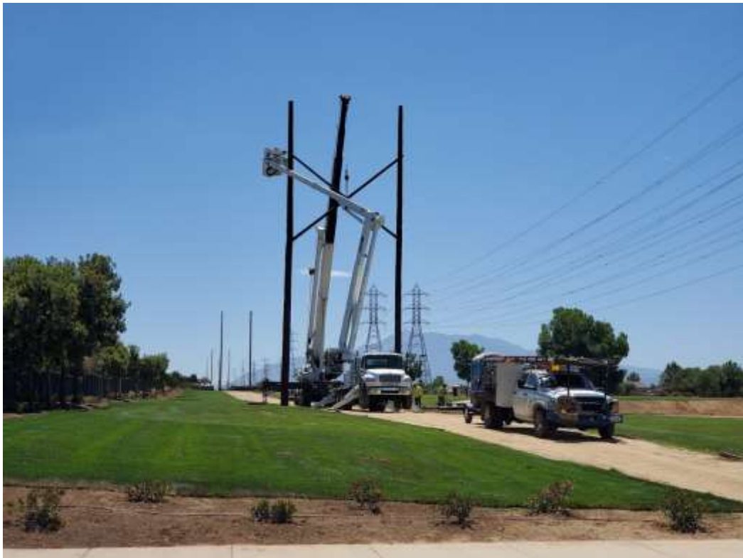
Photo 3 – Tower wreck-out activities at Construction Area PP123296, Segment 4 (May 26, 2021).
