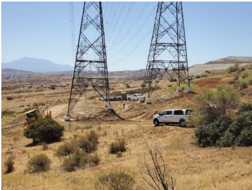
Photo 2 – Site restoration activities at Construction Area 3X61, Segment 3 (May 24, 2021).
