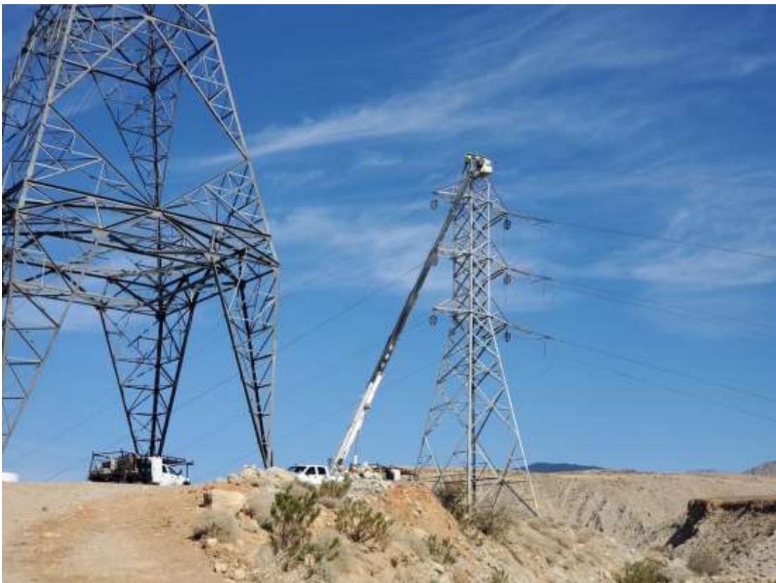
Photo 6 – Wire wreck-out activities at Construction Area 6N28, Segment 6 (May 25, 2021).
