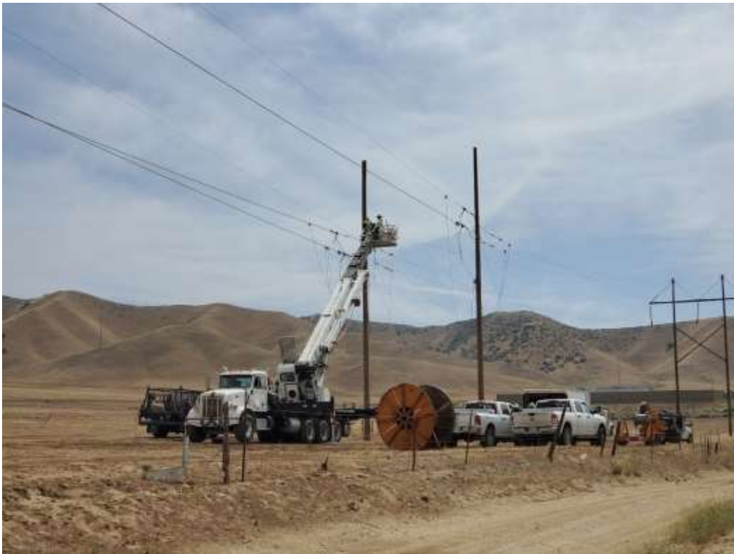
Photo 3 – Wire wreck-out activities at Construction Area 4X16, Segment 4 (June 7, 2021).
