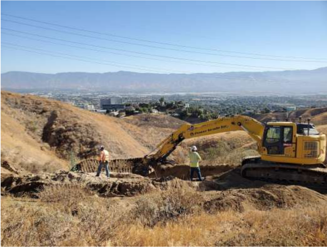
Photo 1 – Hilfiker wall excavation at Construction Area SWA-2-2N12-2-MPR-43, Segment 2 (June 10, 2021).
