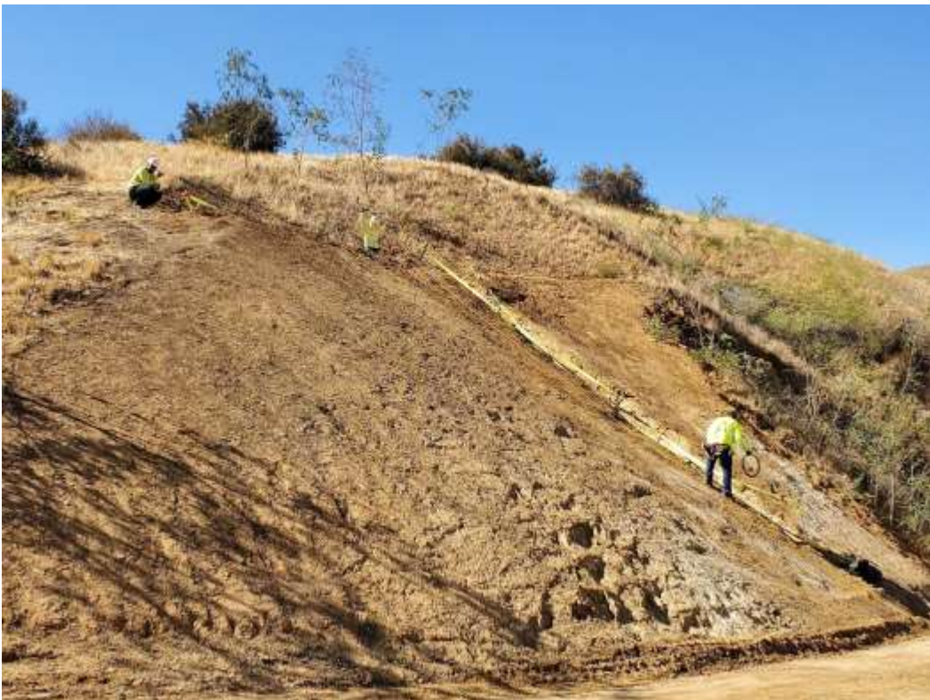
Photo 2 – V-ditch excavation at Construction Area 3X62, Segment 3 (June 10, 2021).
