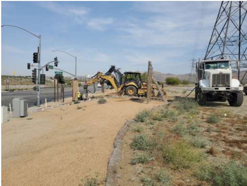
Photo 5 – Foundation wreck-out at Construction Area 4175193E (5X29), Segment 5 (June 15, 2021).
