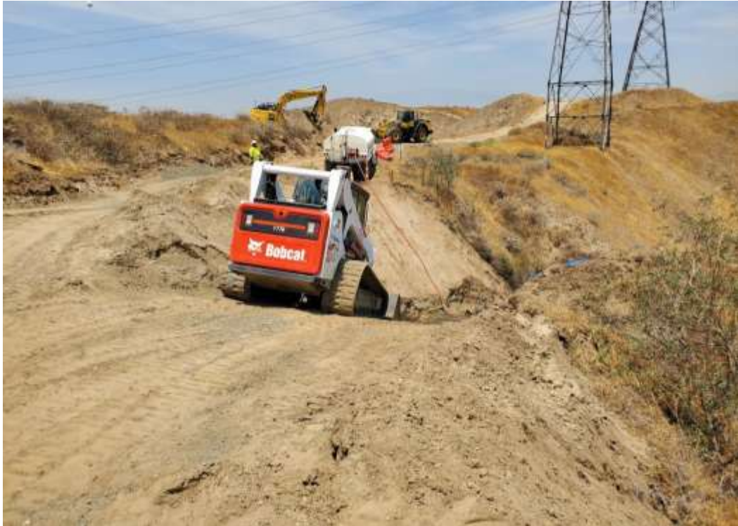
Photo 1 – Hilfiker wall excavation at Construction Area SWA-2-2N12-2-MPR-43, Segment 2 (June 16, 2021).
