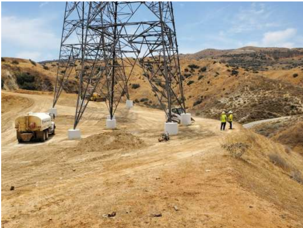
Photo 2 – Site restoration activities at Construction Area 3X44, Segment 3 (June 15, 2021).
