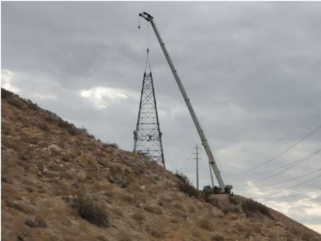
Photo 6 – Tower wreck-out at Construction Area 6N31, Segment 6 (June 22, 2021).
