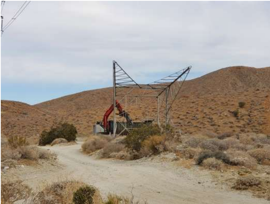
Photo 5 – Tower shearing at Construction Area 5X06, Segment 5 (June 22, 2021).
