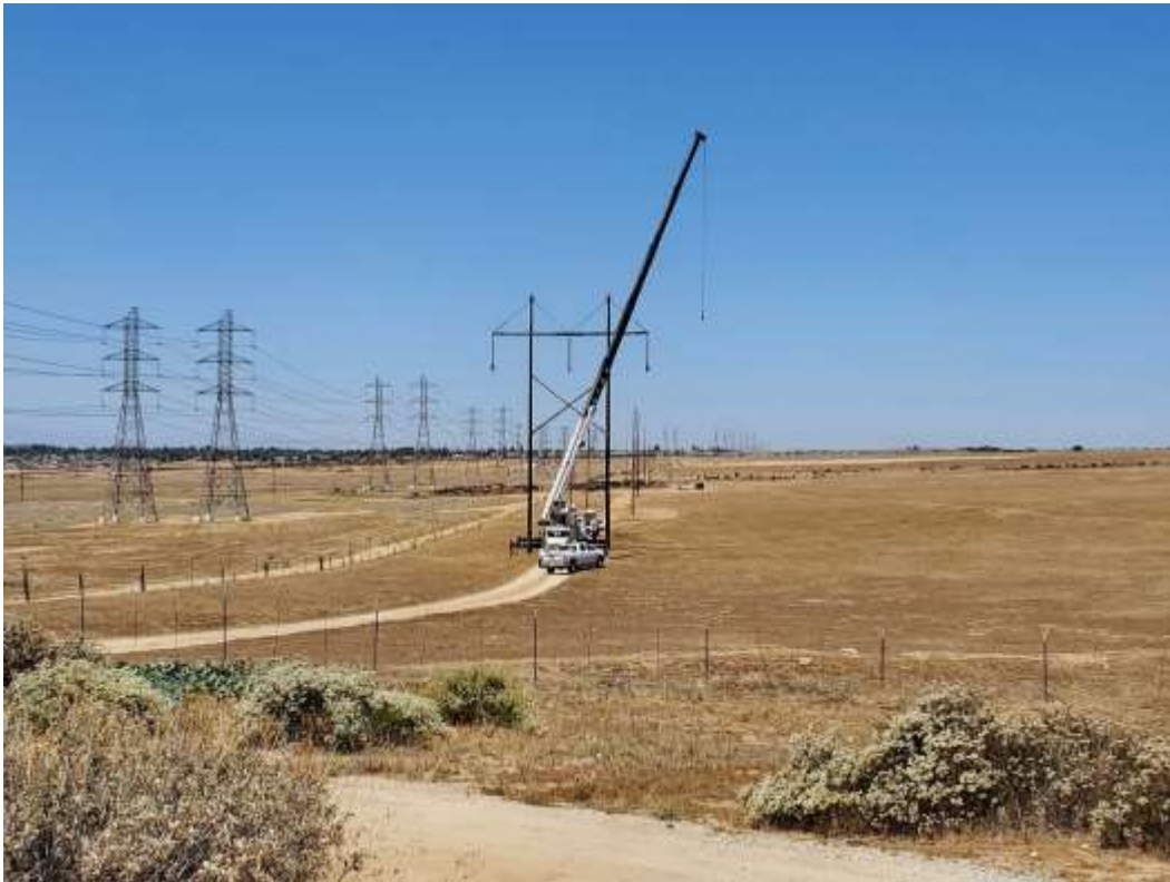
Photo 3 – H-frame pole wreck-out activities at Construction Area 4X16, Segment 4 (June 21, 2021).
