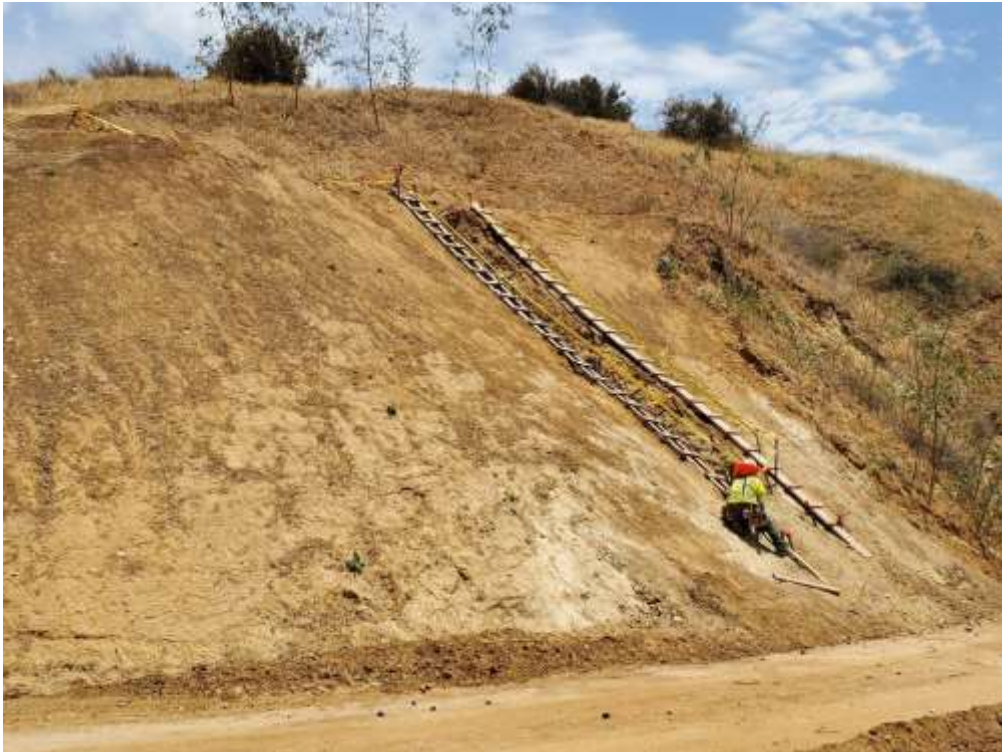
Photo 2 – V-ditch installation at Construction Area 3X62, Segment 3 (June 22, 2021).
