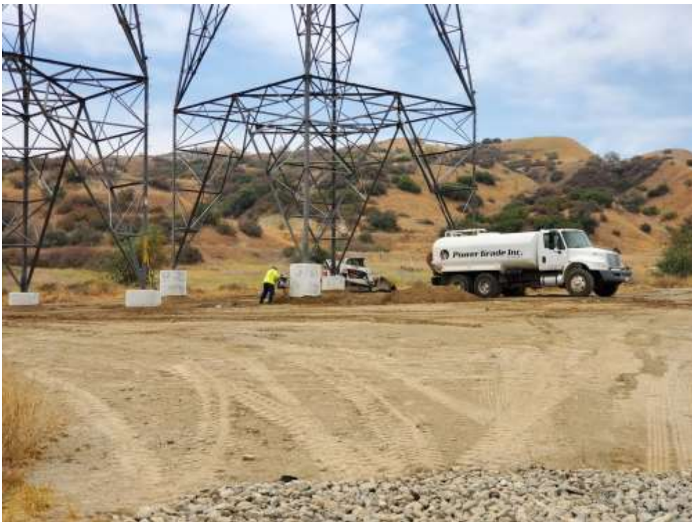
Photo 2 – Site restoration and foundation compaction at Construction Area 3X29, Segment 3 (June 29, 2021).
