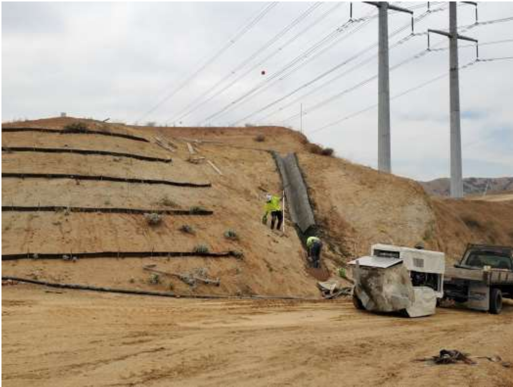
Photo 3 – V-ditch installation at Construction Area 3X46, Segment 3 (June 29, 2021).
