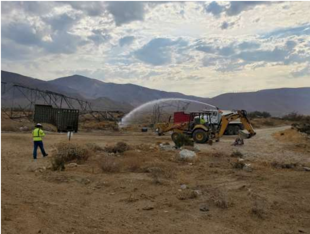
Photo 5 – Foundation wreck-out at Construction Area M7-T4, Segment 6 (June 29, 2021).
