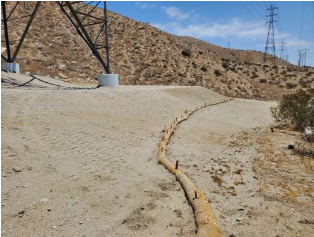
Photo 7 – Hydroseeded area at Construction Area 6S31A, Segment 6 (June 30, 2021).
