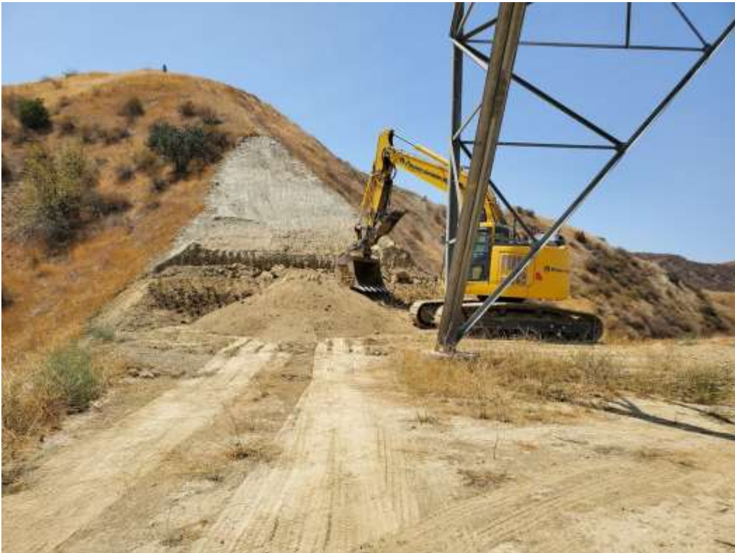
Photo 2 – Site restoration at Construction Area 3S04, Segment 3 (July 14, 2021).
