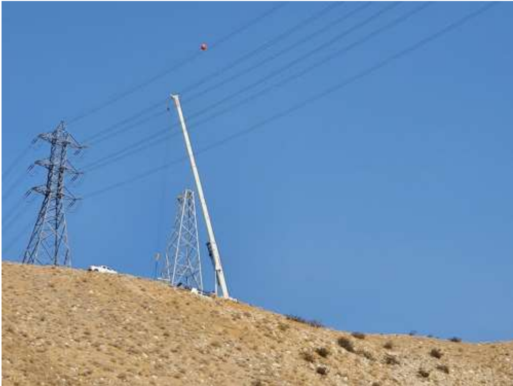
Photo 6 – Tower wreck-out at Construction Area 6N29, Segment 6 (July 12, 2021).
