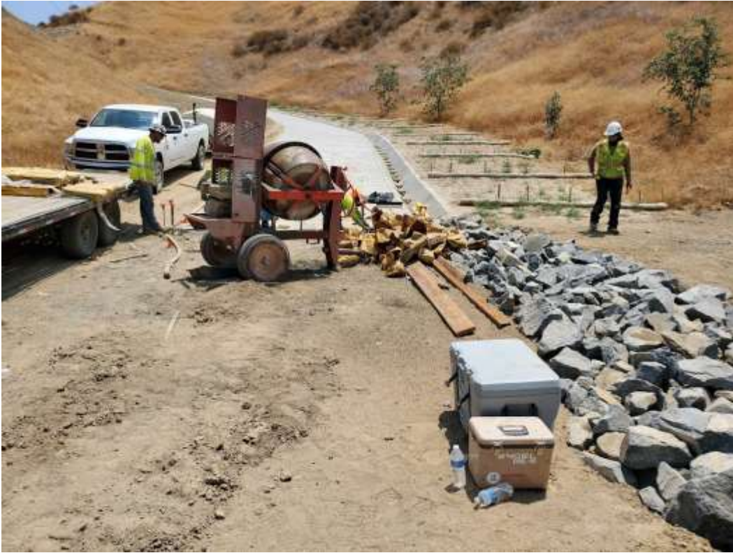
Photo 1 – Bollard installation at Construction Area 2N18, Segment 2 (July 14, 2021).
